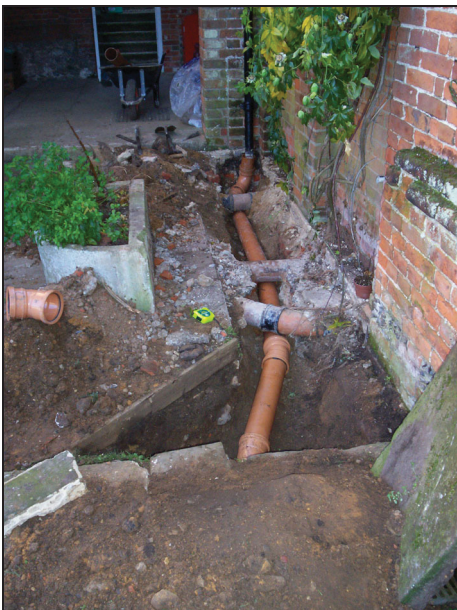
Plate 3 Area 2: Excavated trench looking north
