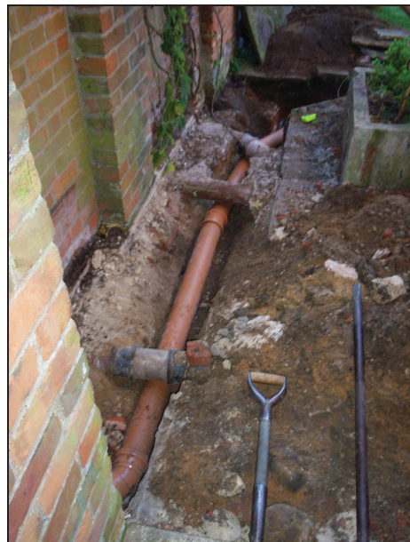
Plate 4 Area 2: Excavated trench looking south
