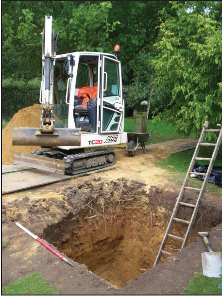
Plate 1 Area 1: Soakaway pit looking NW (1m scale)
