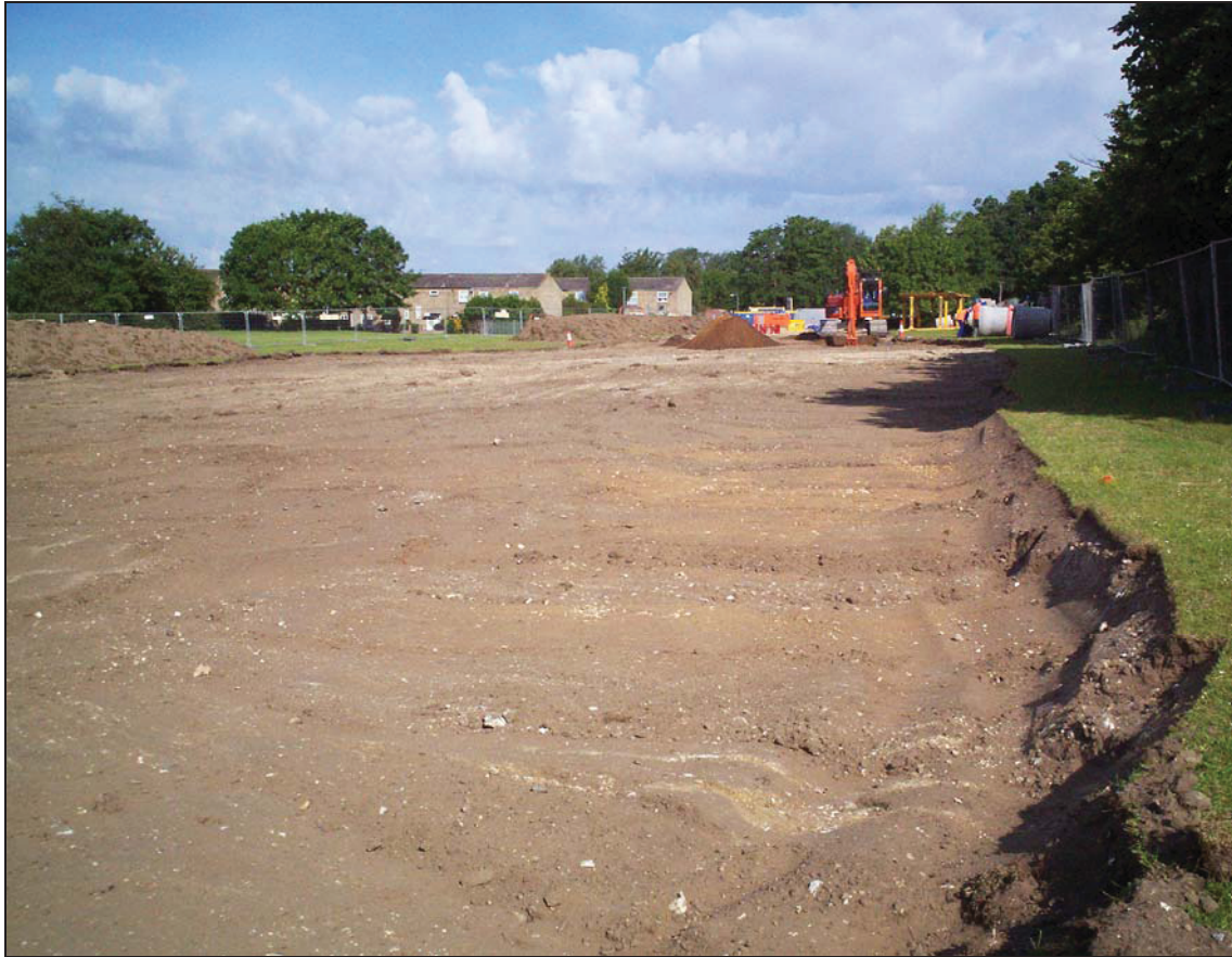
Plate 1 The storm tank area, facing north-west
