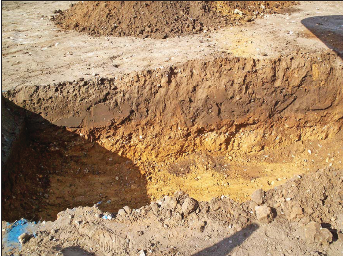
Plate 2 The sewer trench, facing south-west
