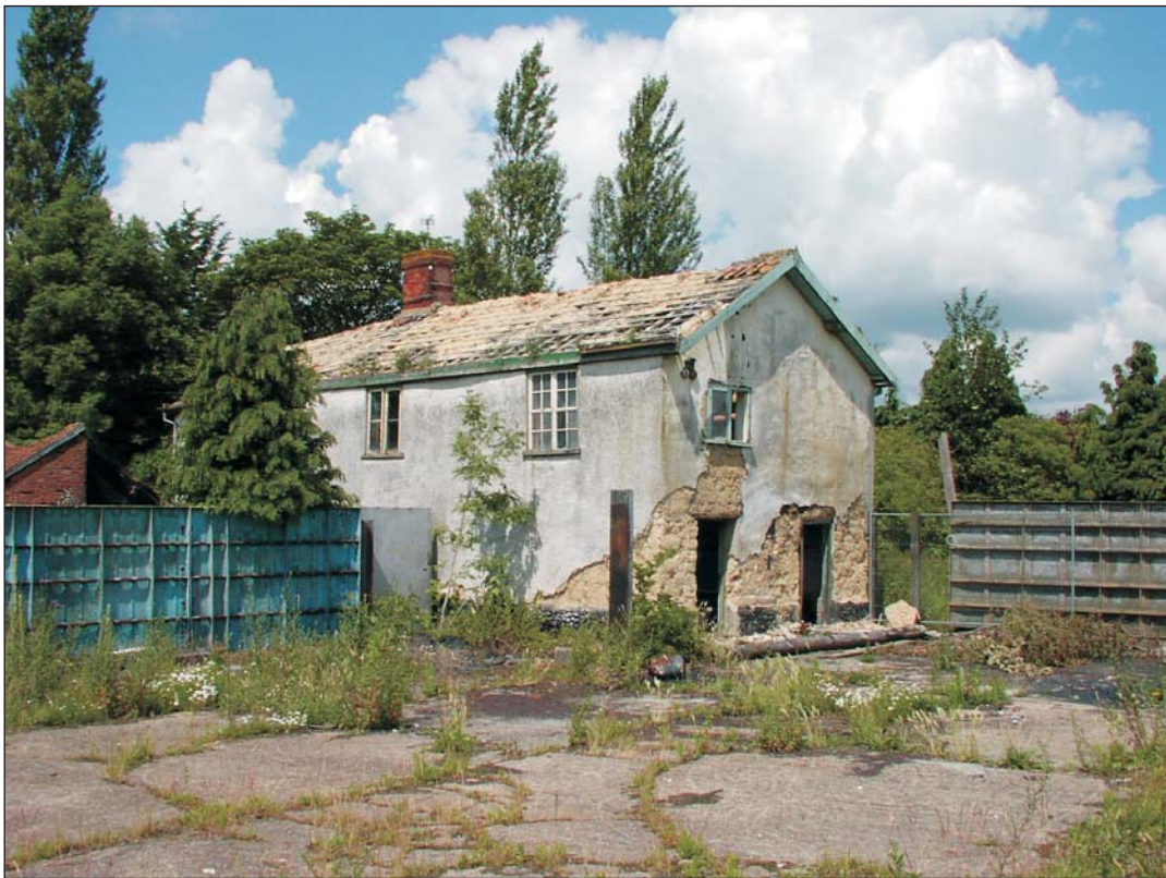
Plates 2. South elevation looking north-west
