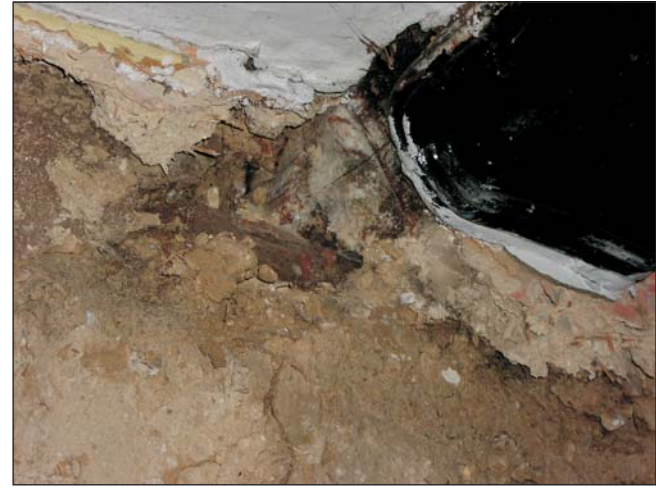
Plate 12. Chamfer stop partly within wall
