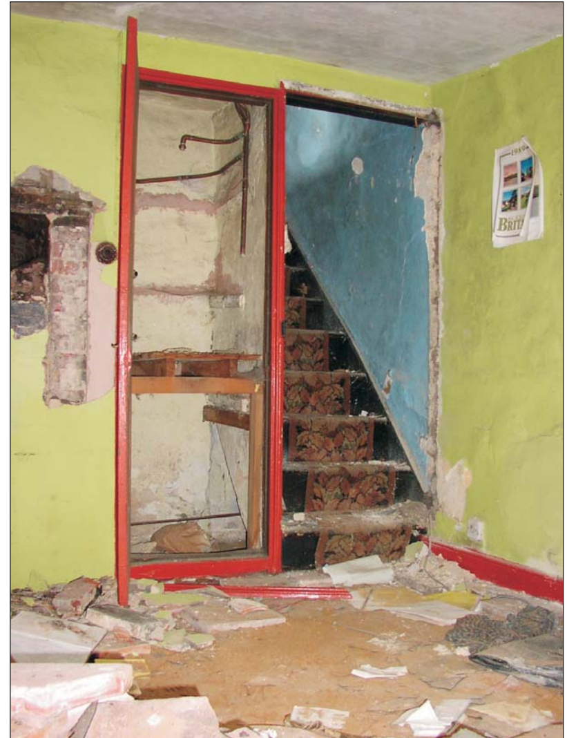
Plate 10. Stairs up to first floor level
