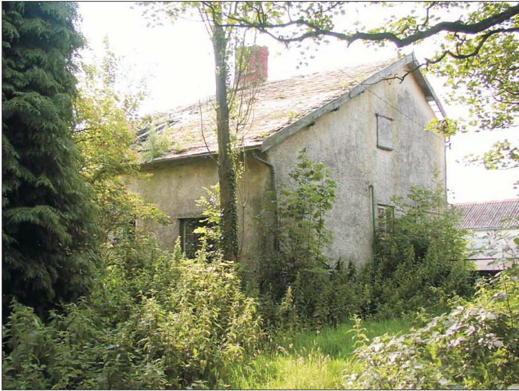
Plate 14. The west end and part of the north elevation
