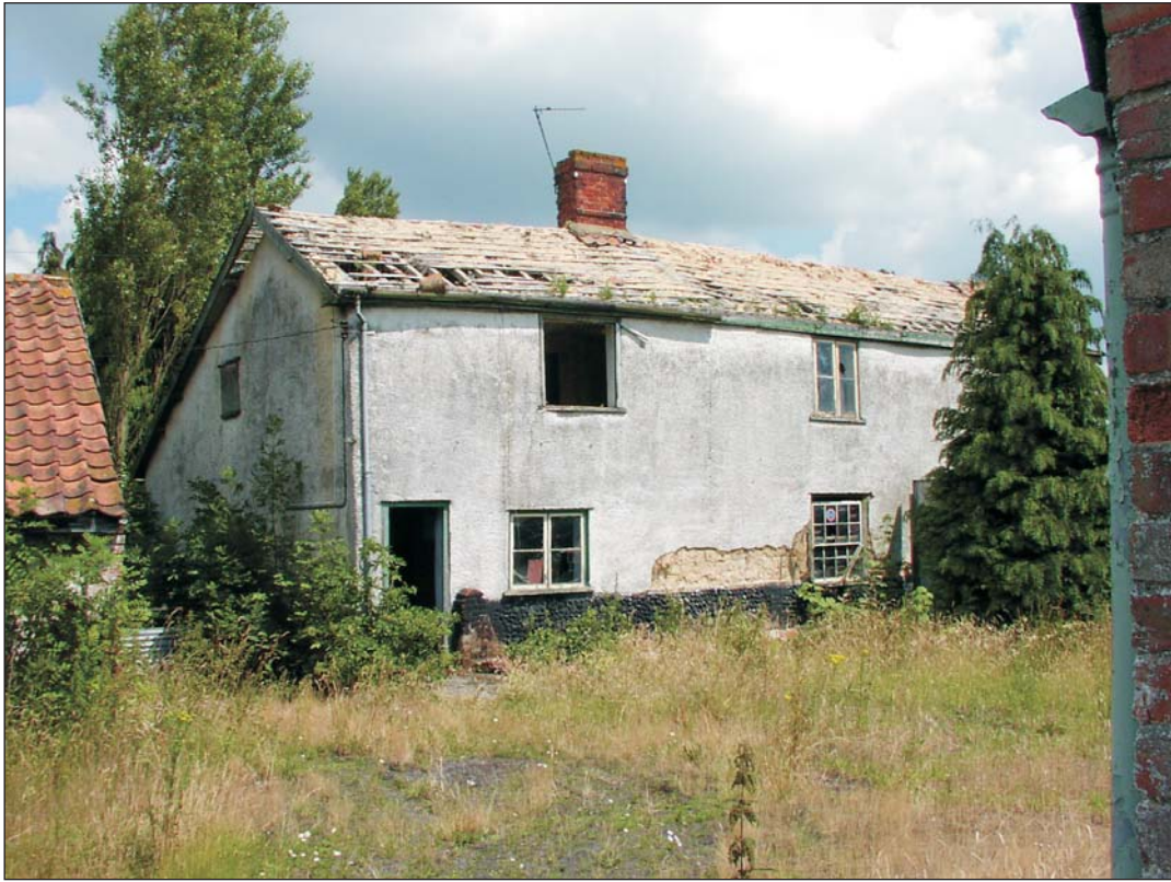
Plates 1. South elevation looking north-east
