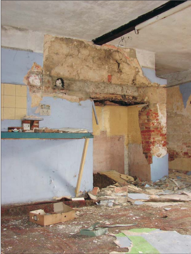
Plate 6. Fireplace in the west room
