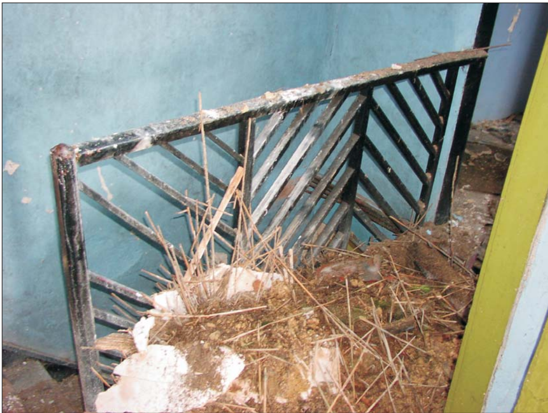
Plate 15. The baluster associated with the ?replacement stair
