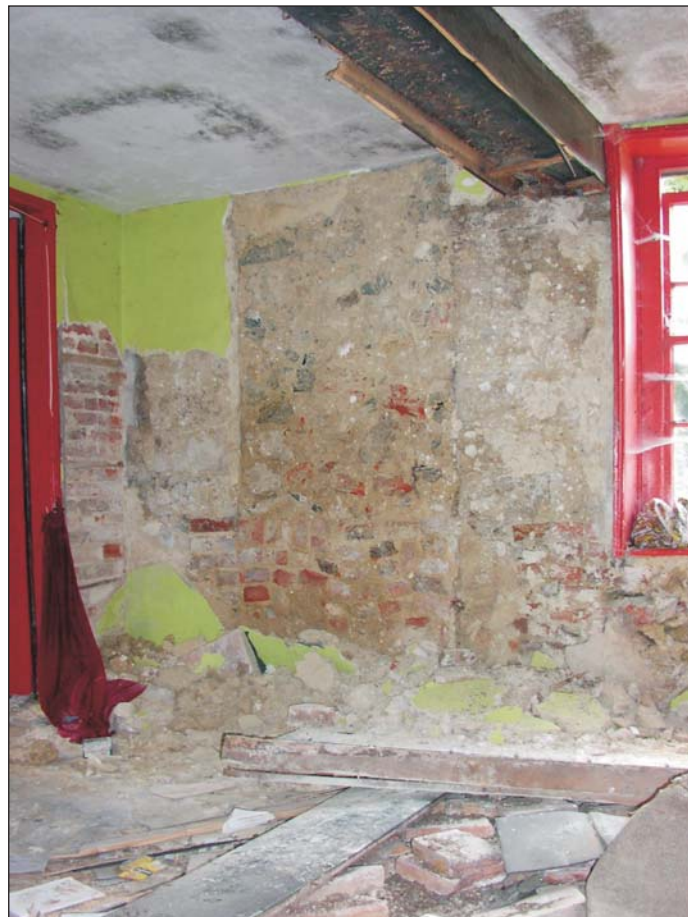
Plate 8. Blocked doorway in the south wall of the central room
