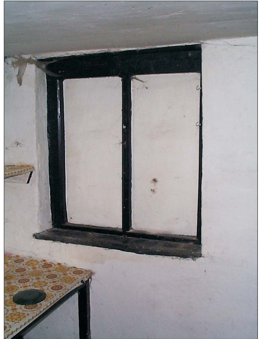
Plate 4. Room 3, former window
