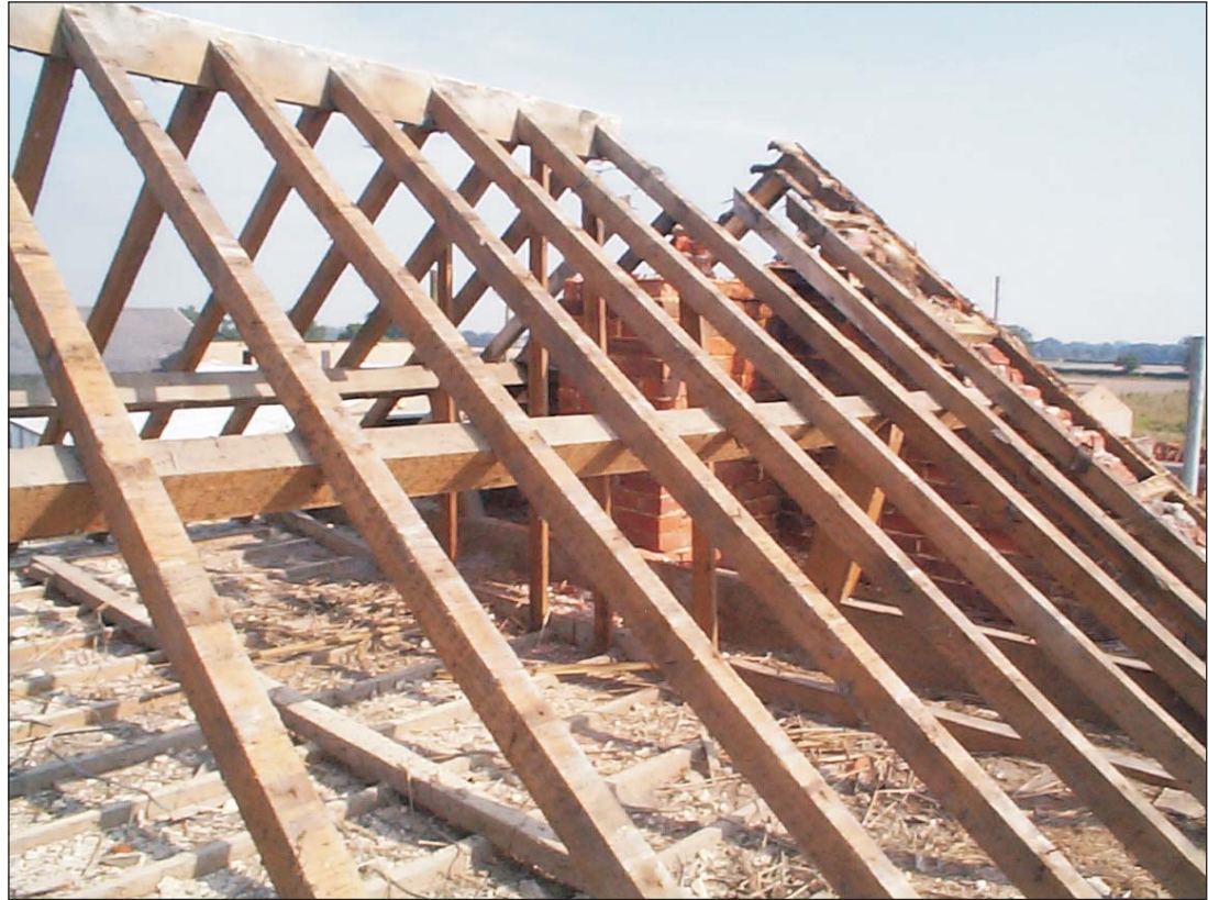
Plate 6. Roof timbers
