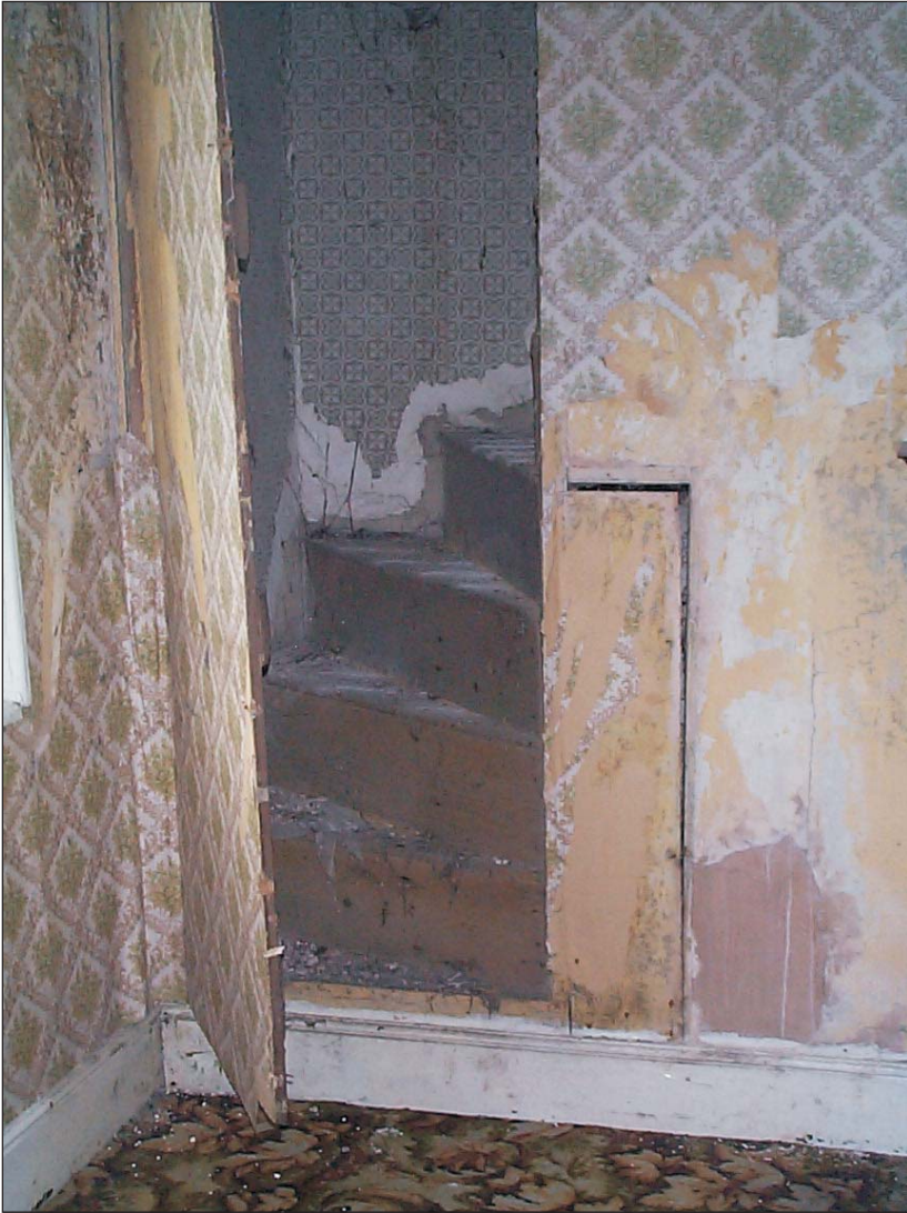
Plate 3. Room 1, stairs by stack
