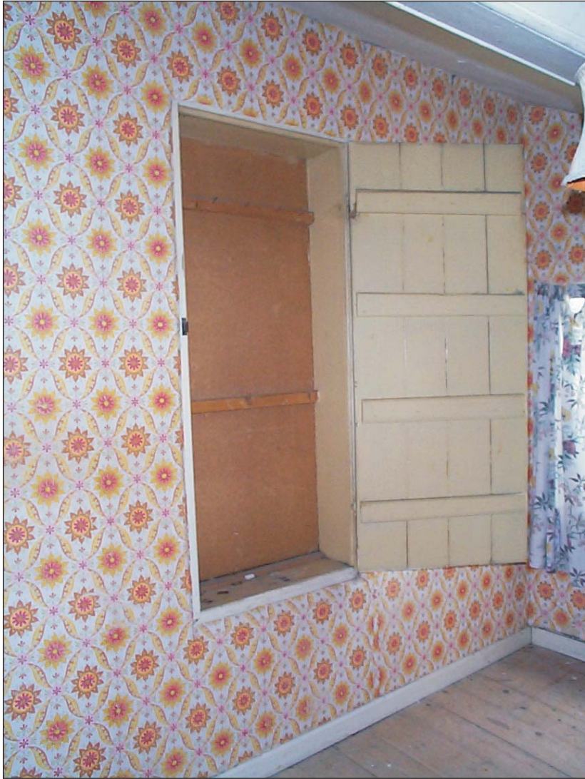
Plate 5. Room 9, door to Room 6
