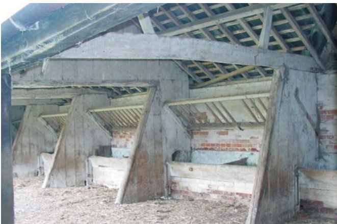
Plate 9 Building C (interior) from south-east
