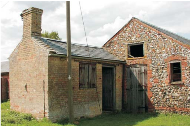
Plate 20 Building F3 Tack Room from south-east
