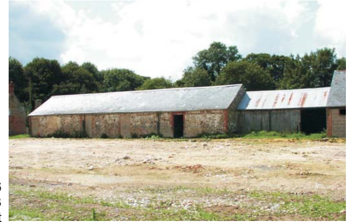
Plate 16 Buildings F2 and F3 from east
