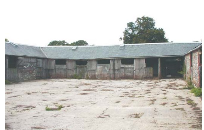
Plate 24 Building G from south
