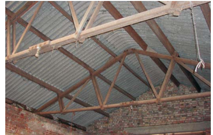
Plate 11 Building E (interior)
