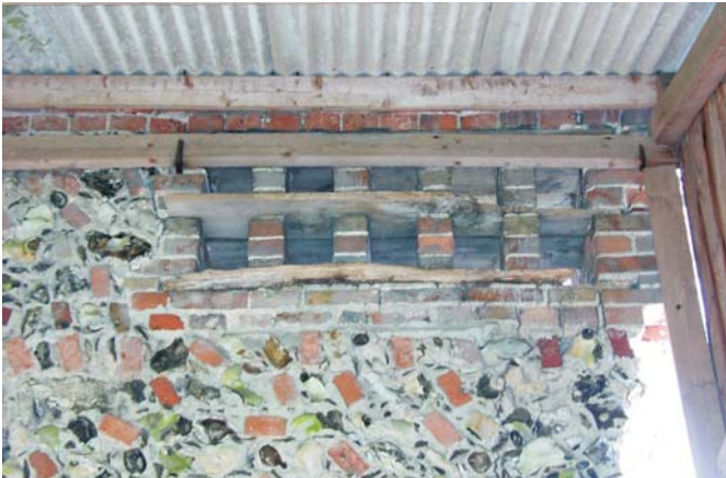
Plate 2 Building A from west (interior)
