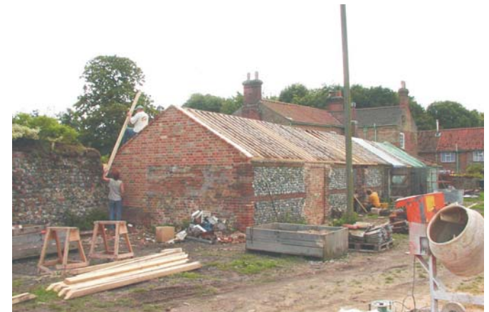
Plate 12 Building E from north-east
