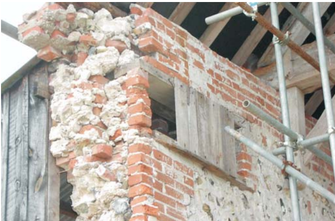
Plate 3 Building A from south
