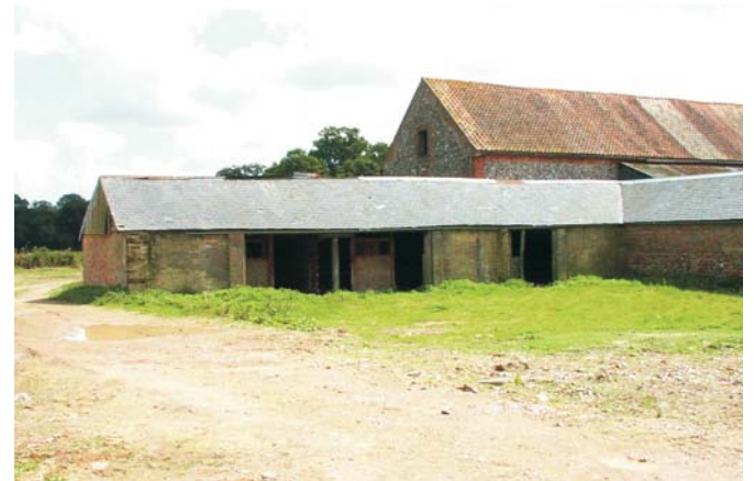
Plate 6 Building B from west
