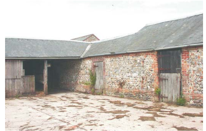
Plate 17 Building F3 from west
