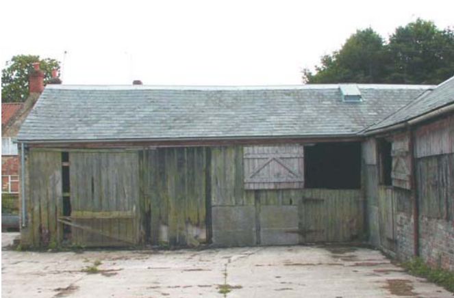
Plate 27 Building G from north
