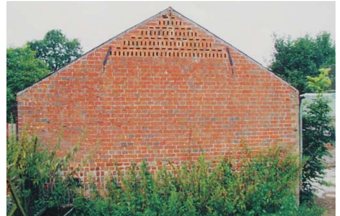
Plate 29 Building G from east
