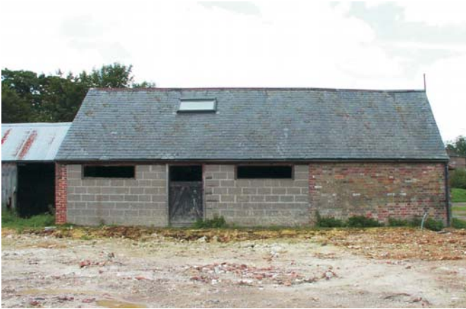
Plate 14 Building F1 from east
