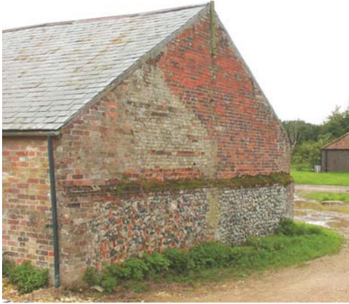
Plate 13 Building F1 from north-east
