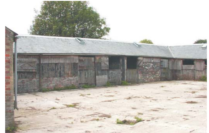
Plate 23 Building G from east
