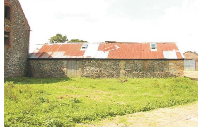
Plate 4 Building B from east
