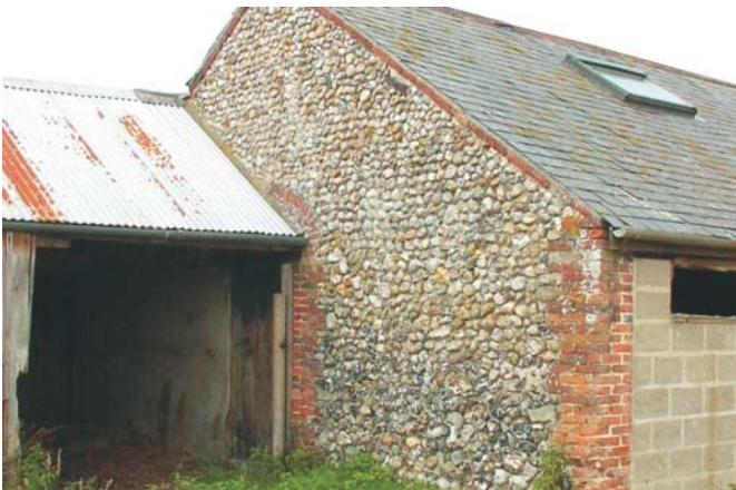
Plate 15 Building F1 from south-east
