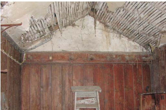
Plate 21 Building F3 Tack Room (interior)
