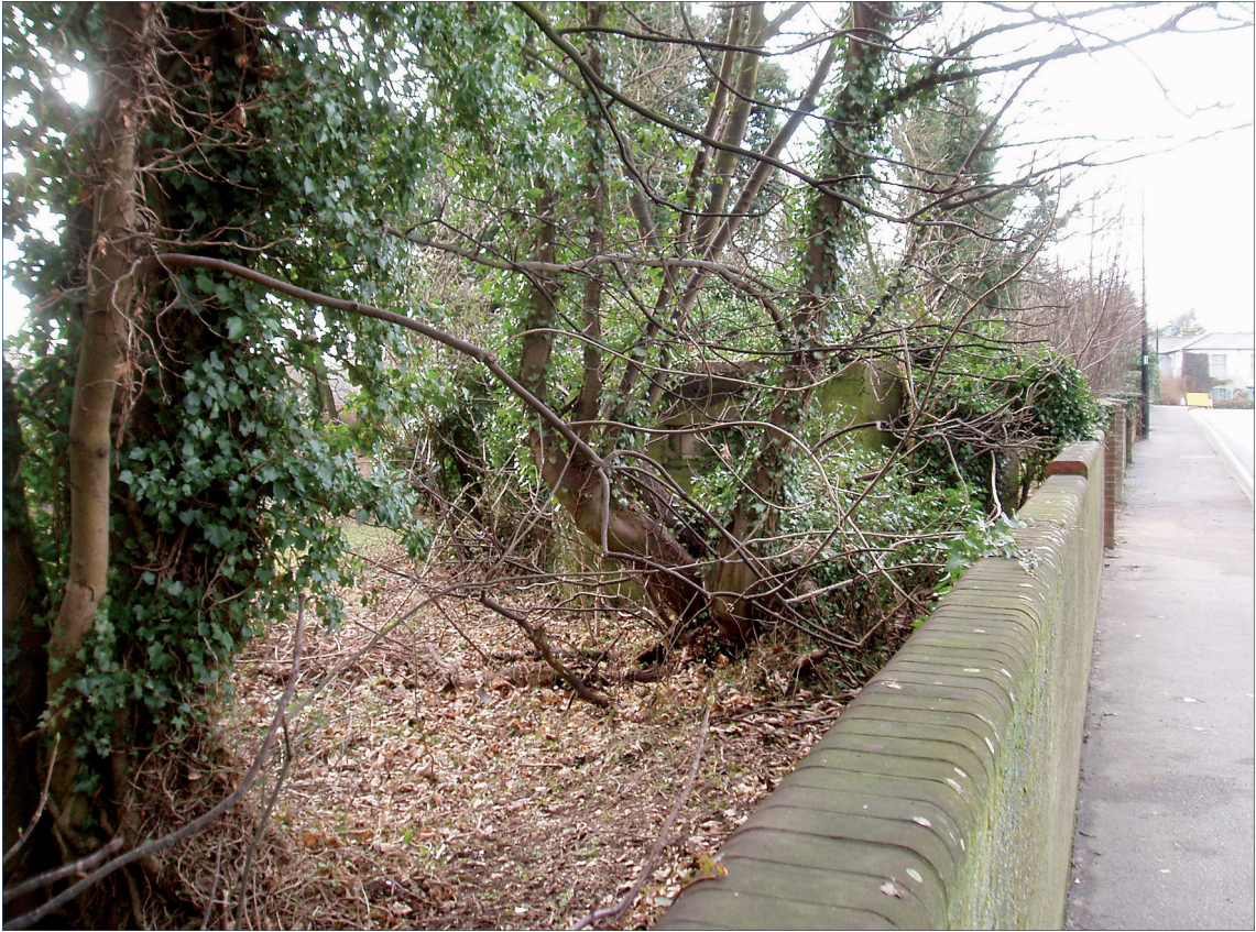
Plate 1 Type 22 pillbox DOB 6304, east of Mill Street, Mildenhall
