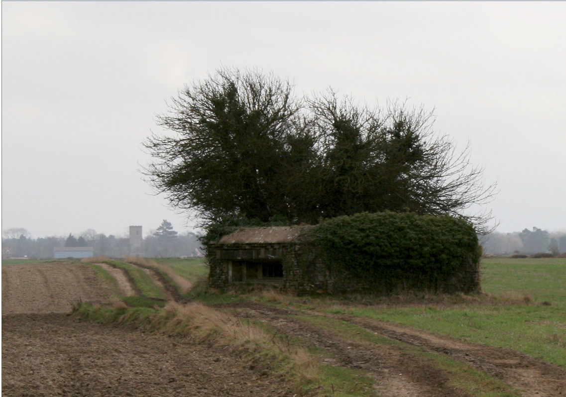
Plate 3 Type 28 pillbox DOB 6440, east of the road leading south from Jude's Ferry Bridge, West Row
