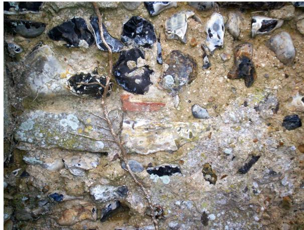
Plate 3. Chancel wall of the parish church showing reused Roman masonry and undated limestone blocks
