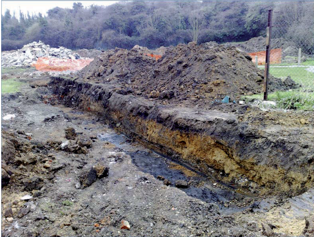
Plate 10. Trench 9, looking north-west.
