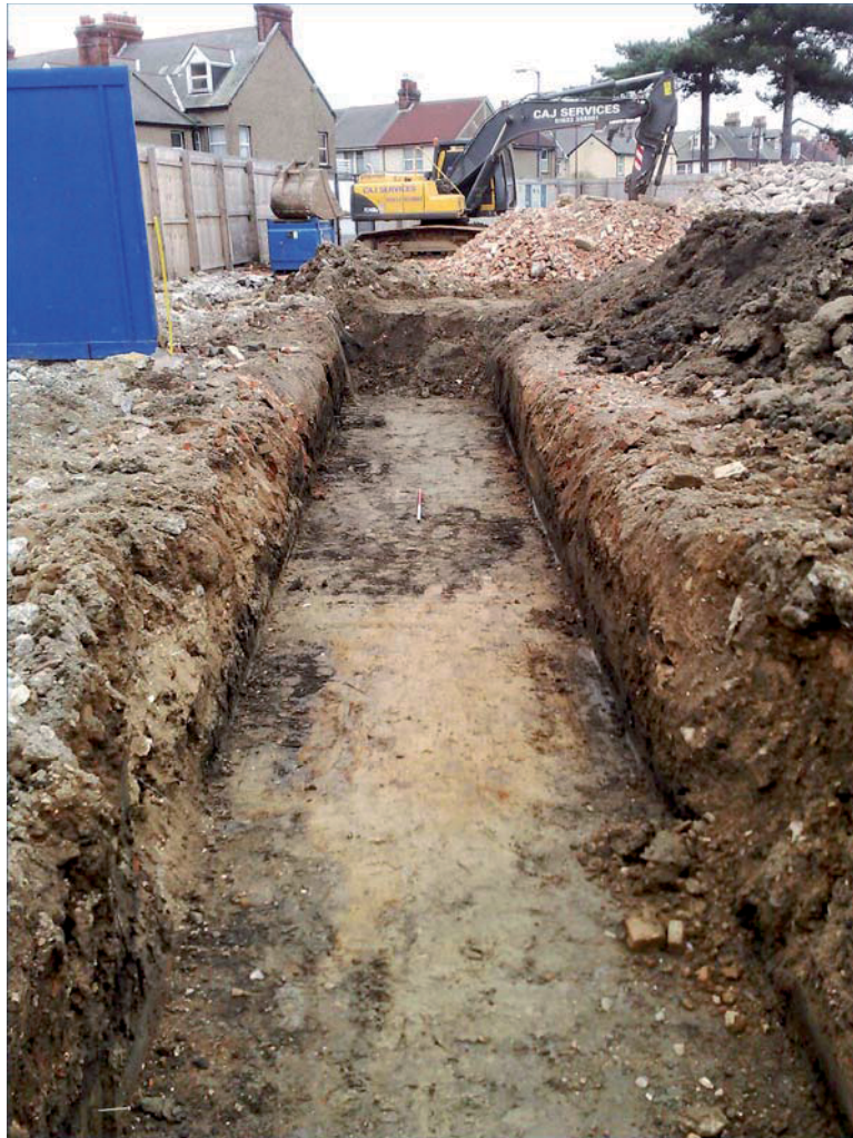
Plate 3. Trench 2, looking south.
