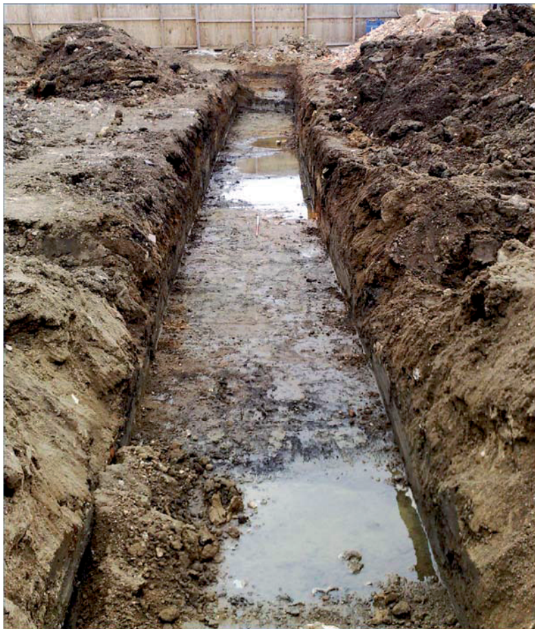
Plate 5. Trench 4, looking east.
