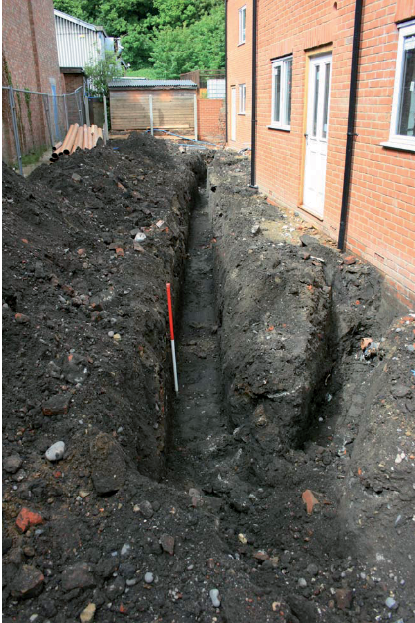
Plate 1: View west along new drainage trench
