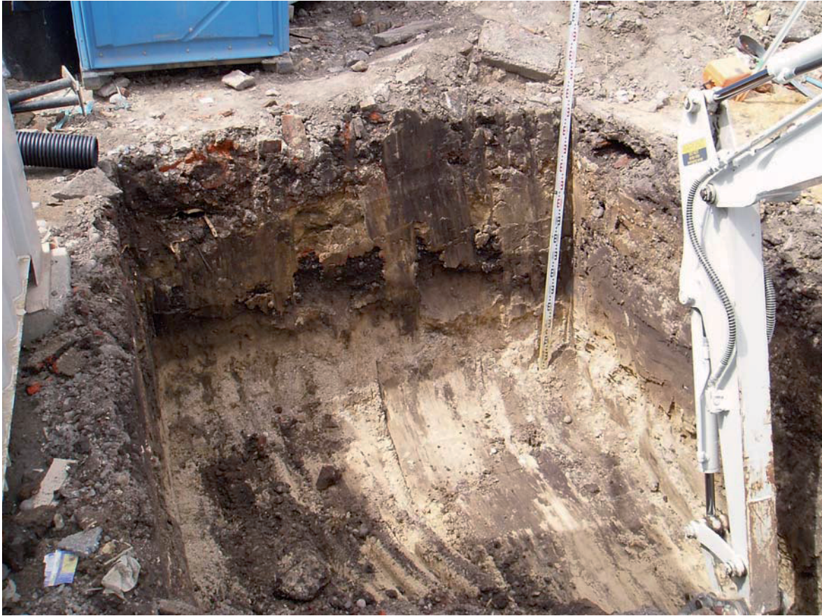
Plate 2: The new soakaway during construction.
