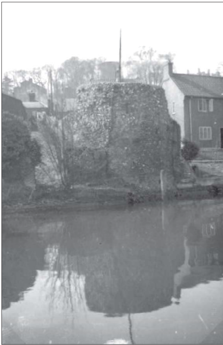
Figure 12. Boom Tower from South 1934. Plunkett
