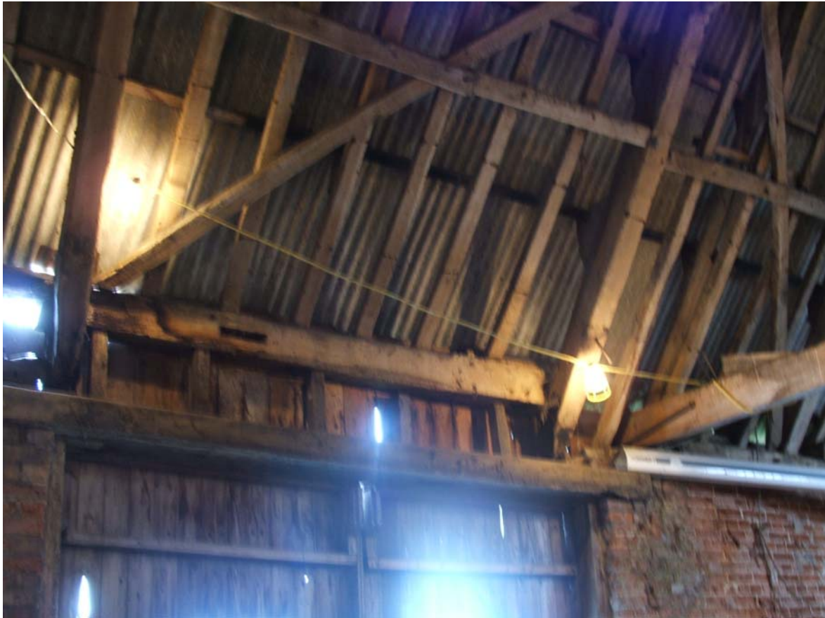
Plate 13. South cart door with inserted reused timber
