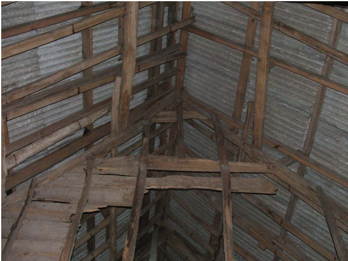
Plate 14. Roof truss at east end above removed wall
