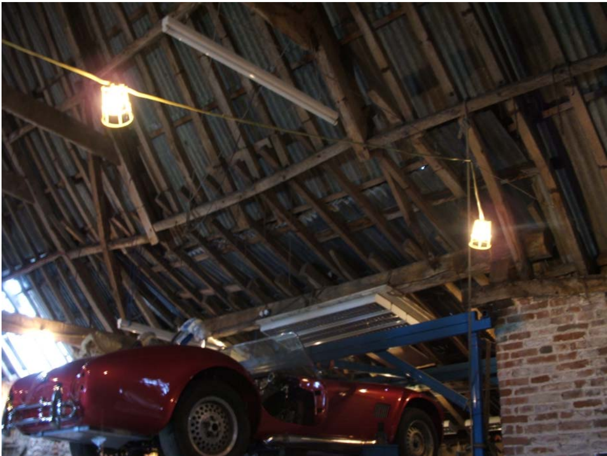
Plate 12. Roof trusses on north side truncated to insert cart porch
