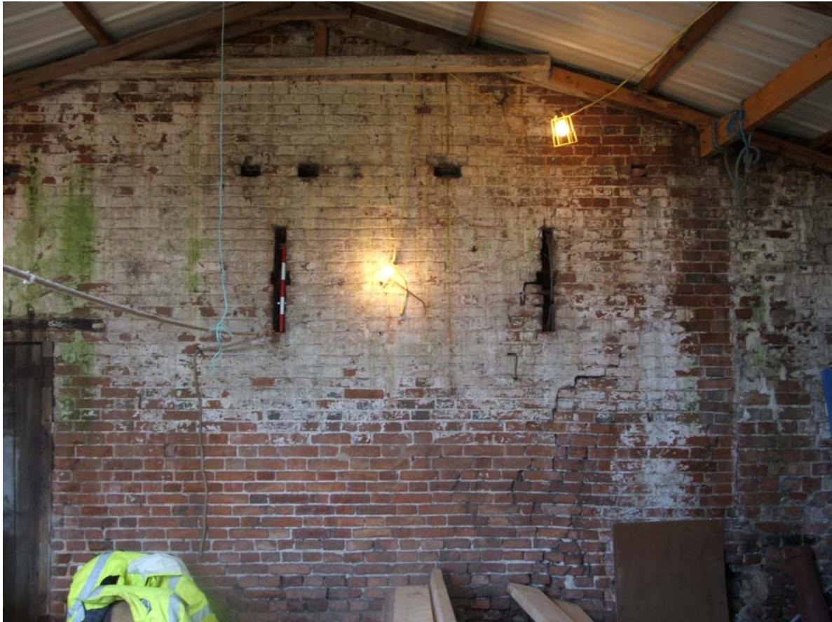
Plate 9. Lower West wall with ventilation slits. (0.5m scale)
