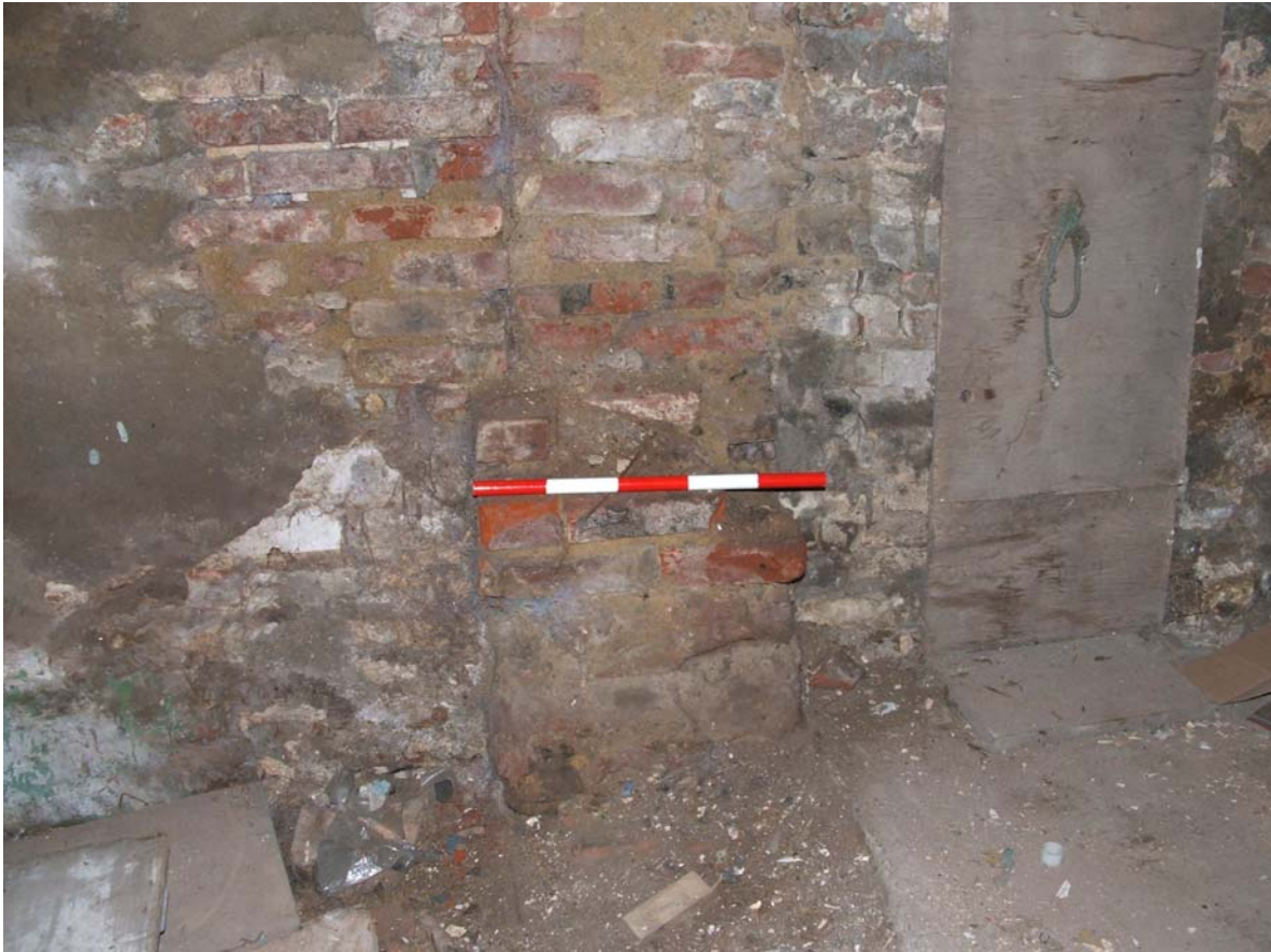
Plate 11. Scar of north-to-south wall with plinth looking south (0.5m scale)
