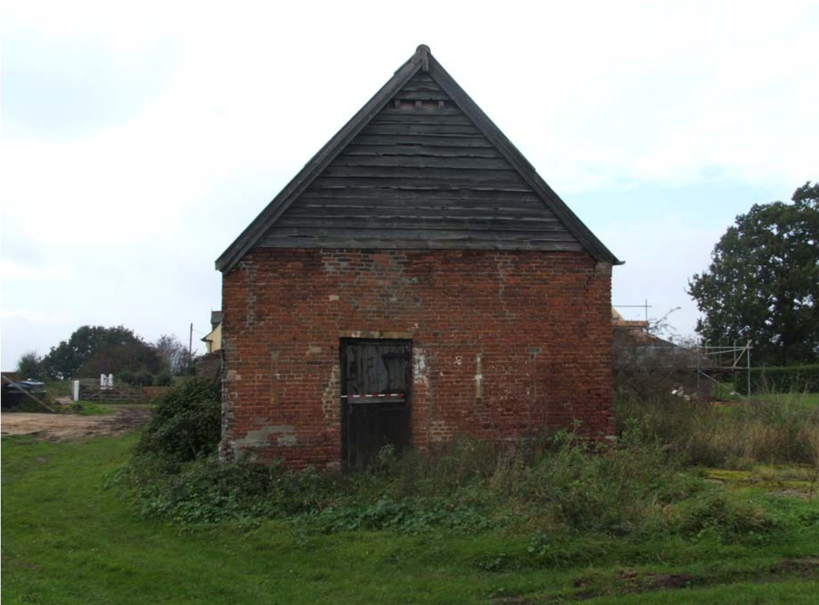
Plate 3. East elevation (1m scale)
