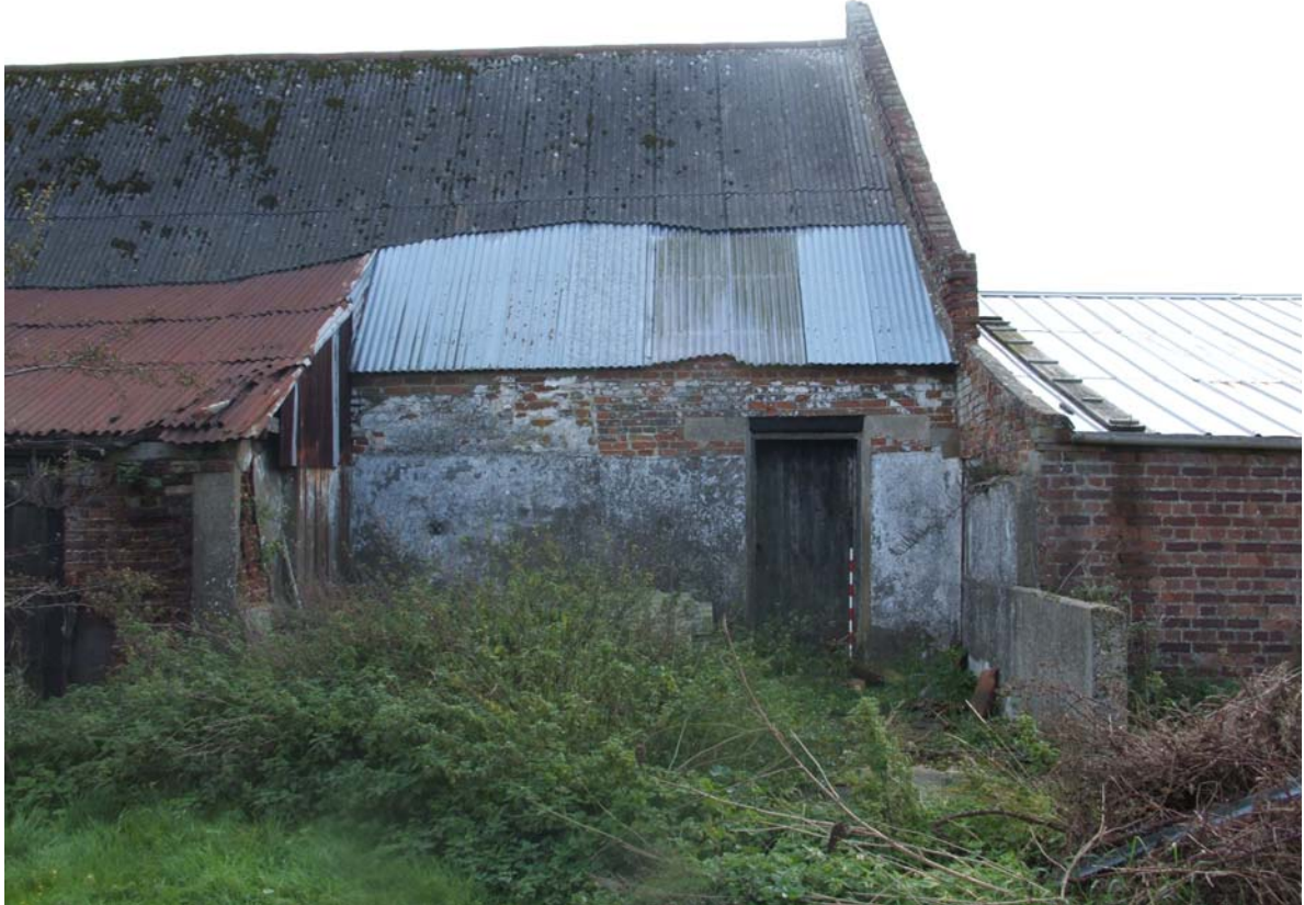
Plate 6. West end of north elevation (1m scale)
