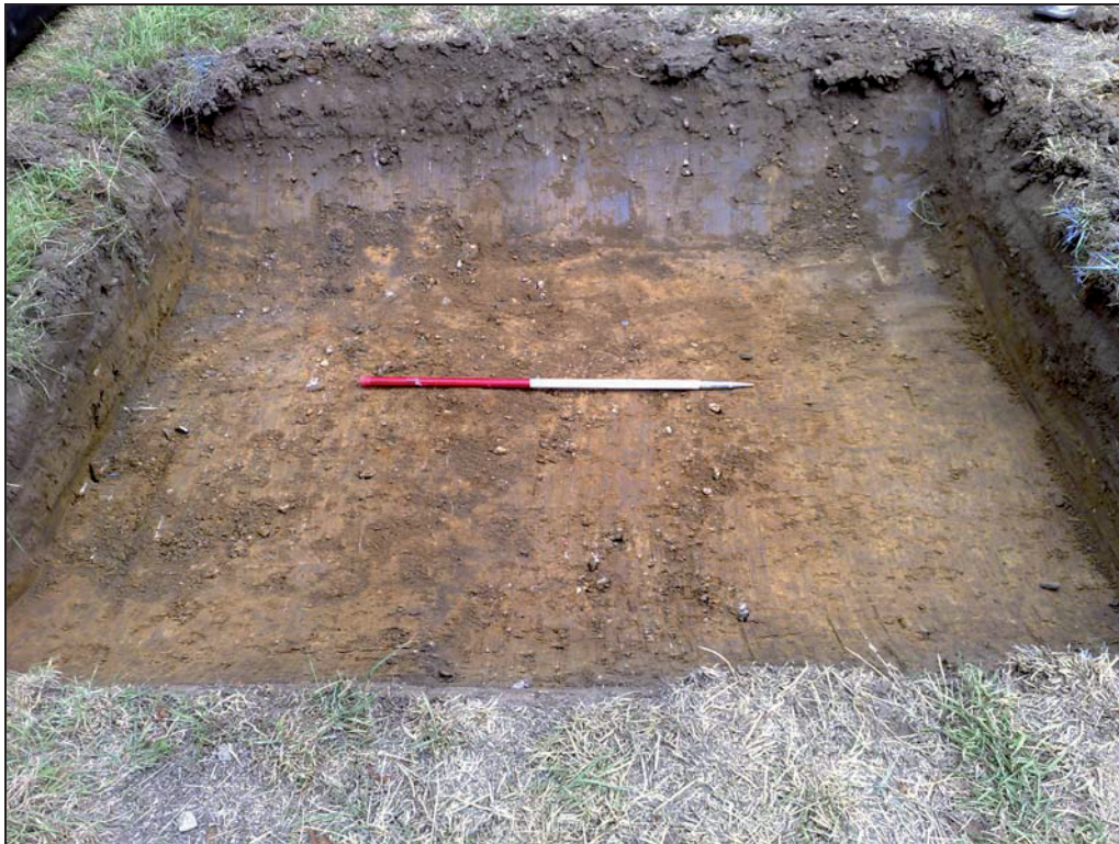
Plate 2. Directional Drilling Pit MH4.
