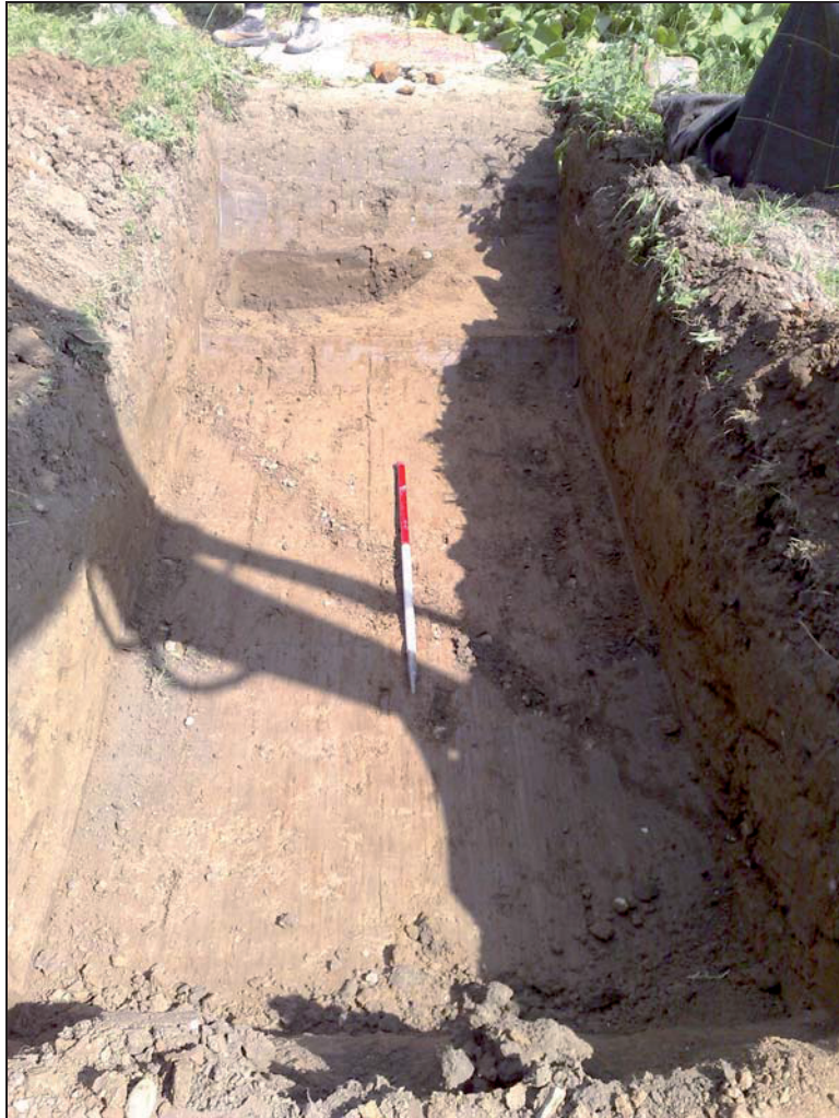
Plate 3. Directional Drilling Pit MH5.
