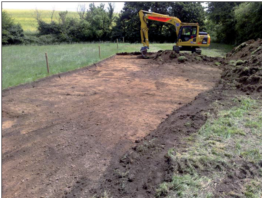
Plate 2. Machining of the easement looking east.
