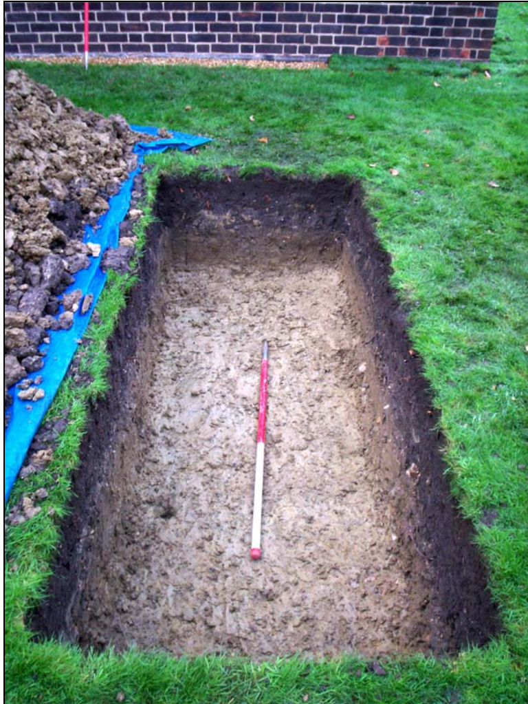
Plate 1. View of the evaluation trench, looking south-west.
