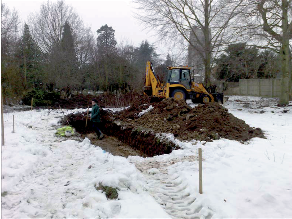
Plate 1. The Site, looking north-west.
