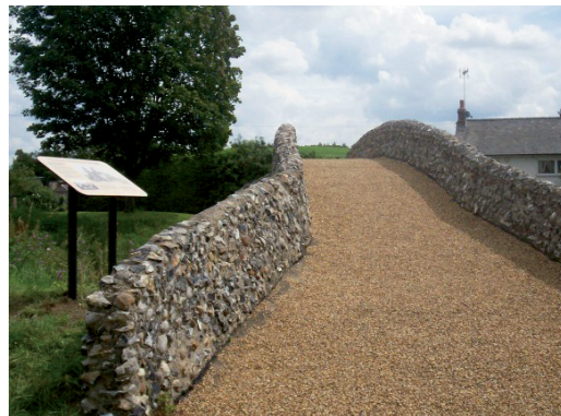
Plate 3. Position of the sign relative to the bridge
