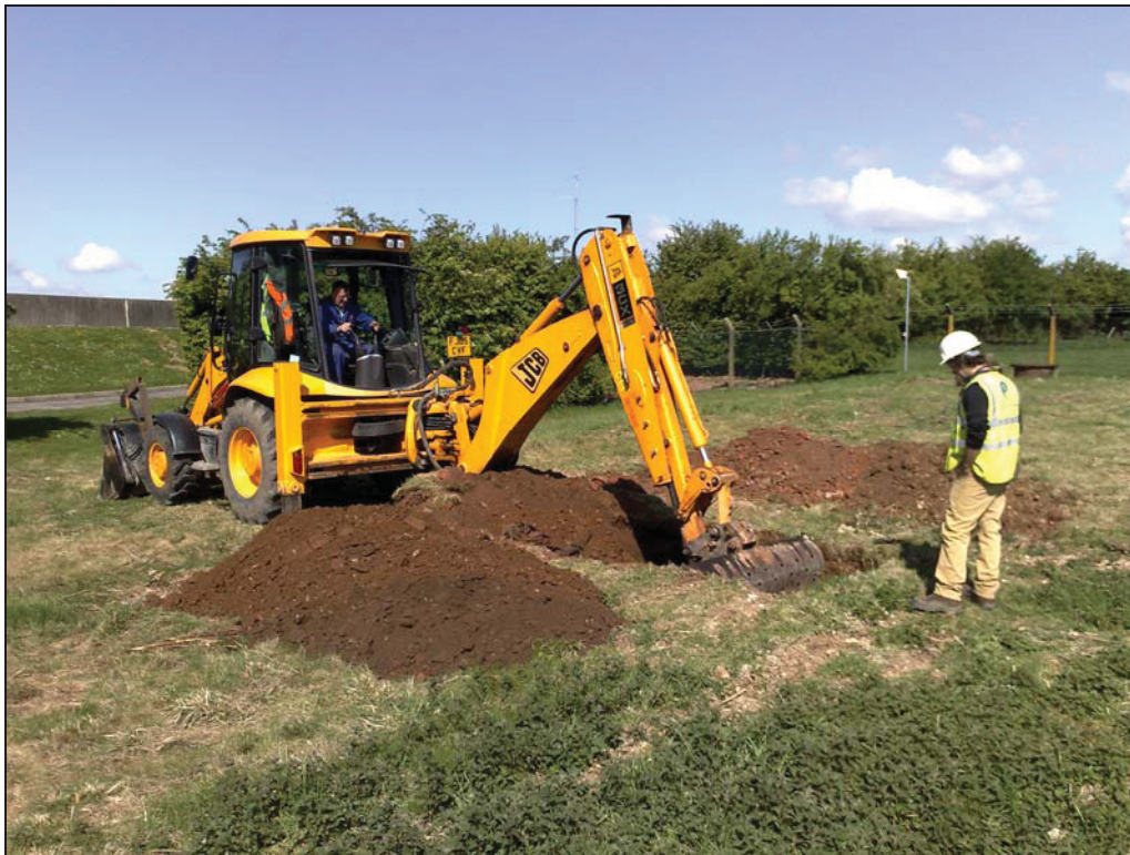
Plate 1. Machining, looking south-west
