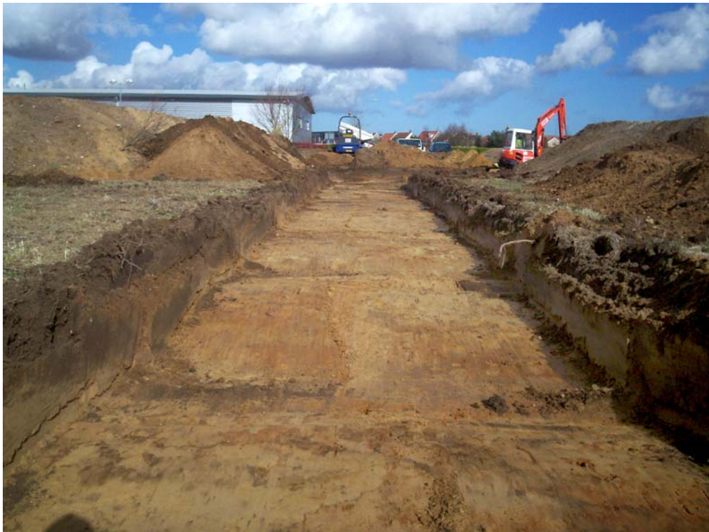
Plate 5. The 3m wide easement south of the ambulance station (looking north).
