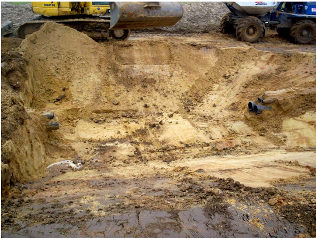
Plate 11. An excavated joint bay
