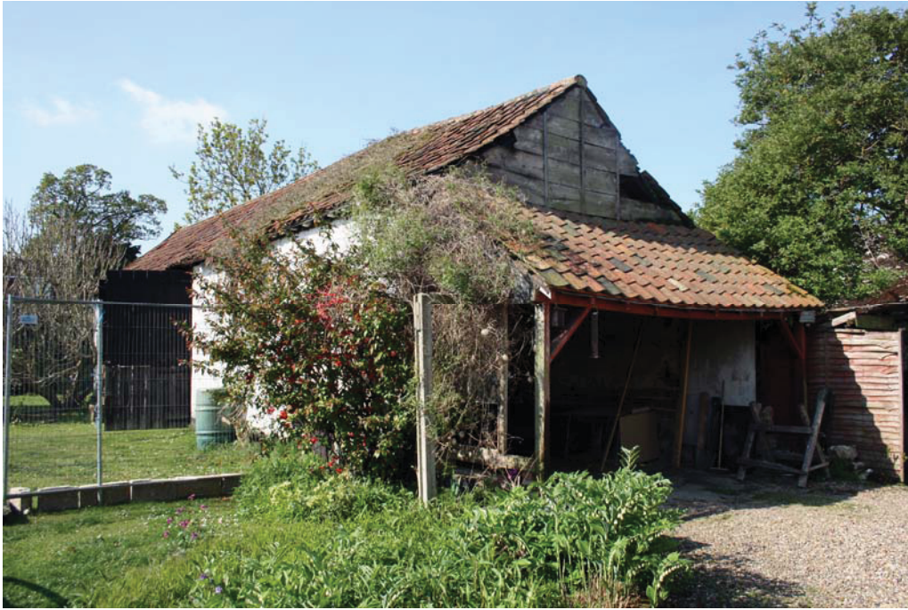
Plate 4. Northern elevation of Building A
