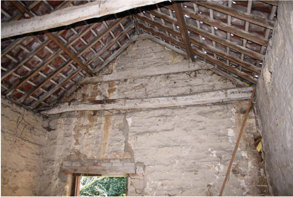
Plate 10. Roof truss in Building A
