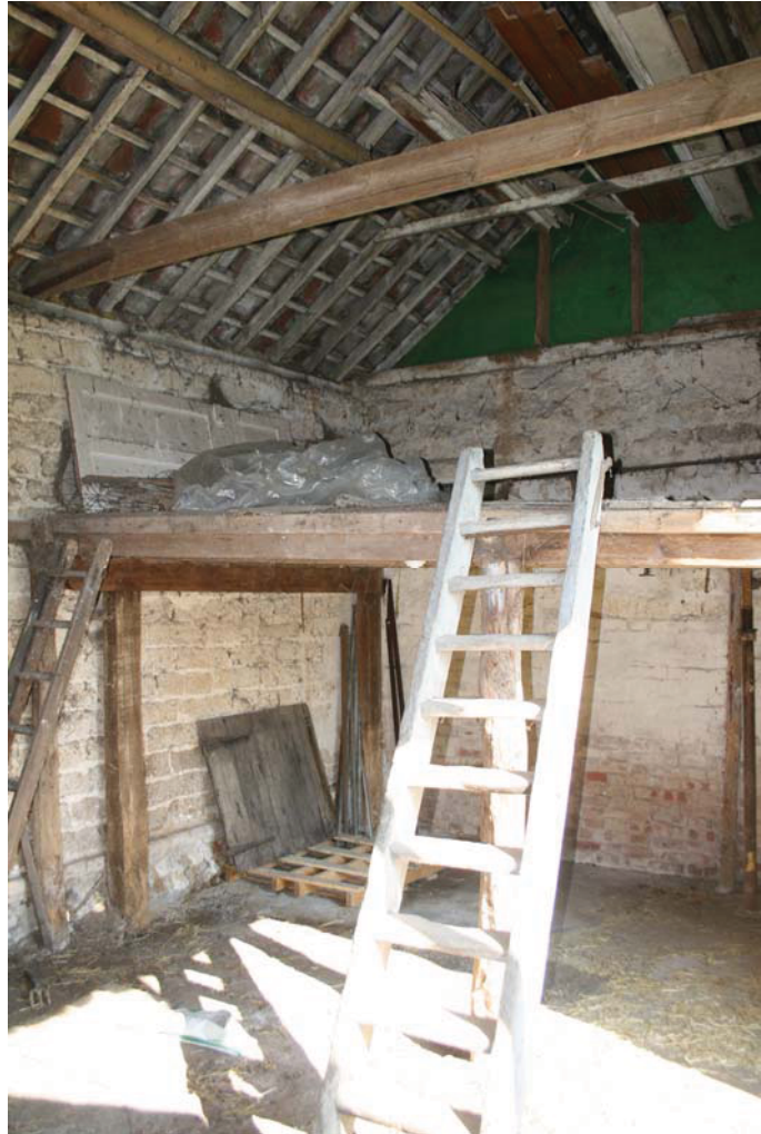
Plate 7. Mezzanine floor in central cell
