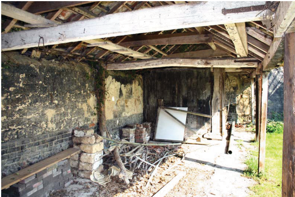
Plate 13. Northern partition in Building B
