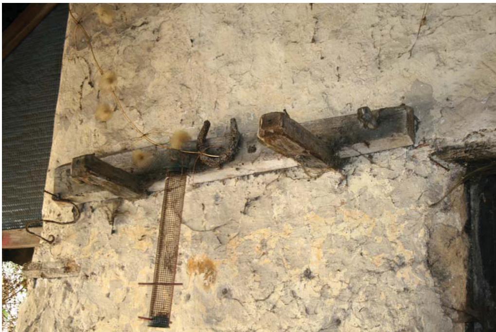
Plate 9. Protruding beams from the southern wall of Building A
