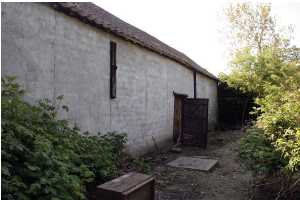
Plate 3. Western elevation of Building A
