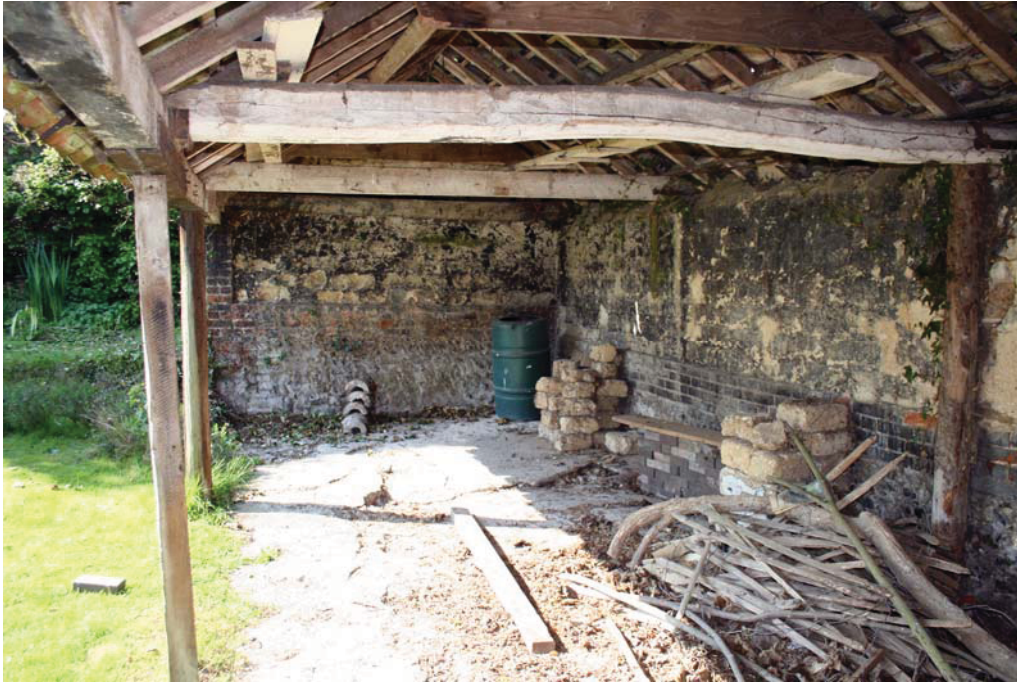
Plate 14. Interior of Building B facing south
