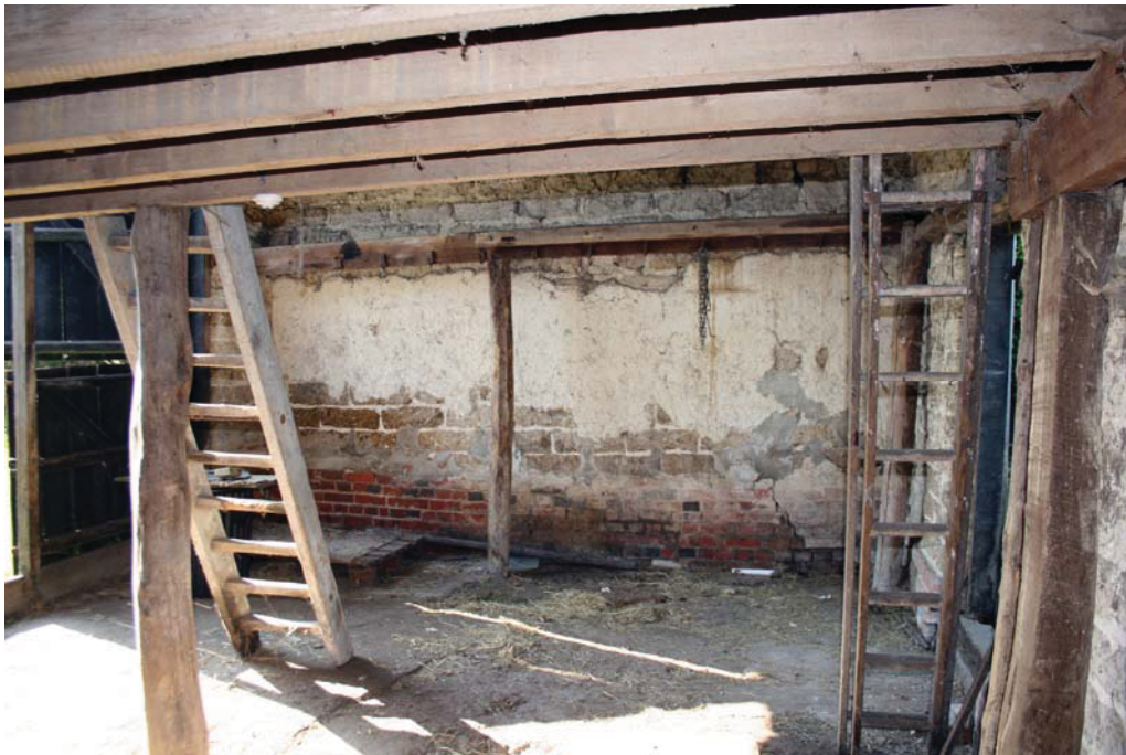
Plate 6. Northern elevation of southern cross wall
