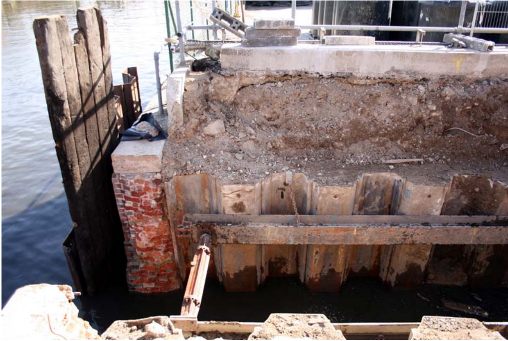
Plate 1. South Cofferdam, showing revetment wall, looking east
