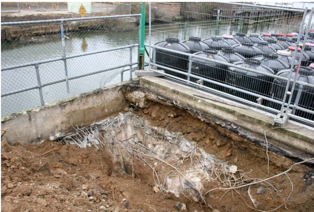
Plate 2. South Cofferd Dam, modern make up and reinforced concrete, looking north-east
