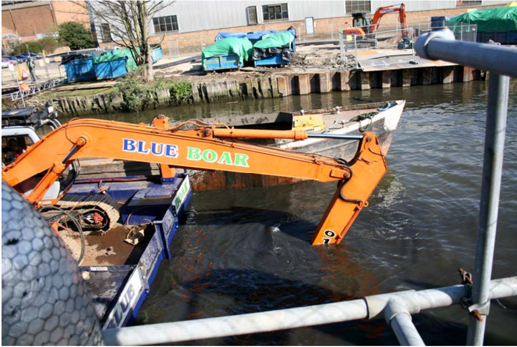
Plate 4. Excavation of trench across river bed, looking north from south bank of River Wensum
