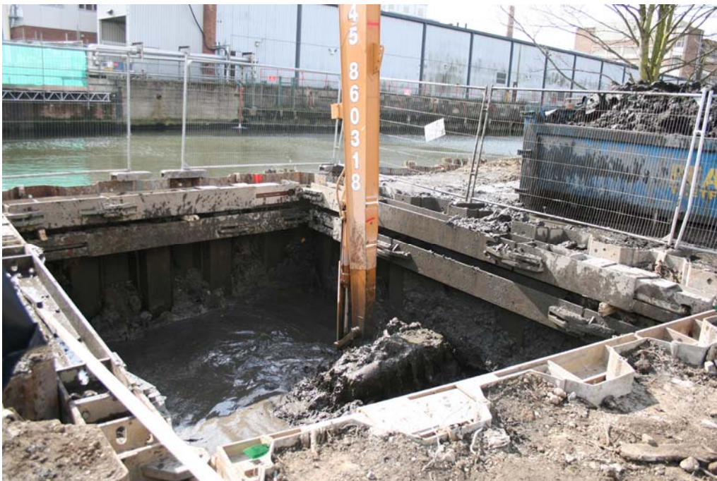
Plate 3. North Coffers Dam, mechanical excavation of peat, looking south.
