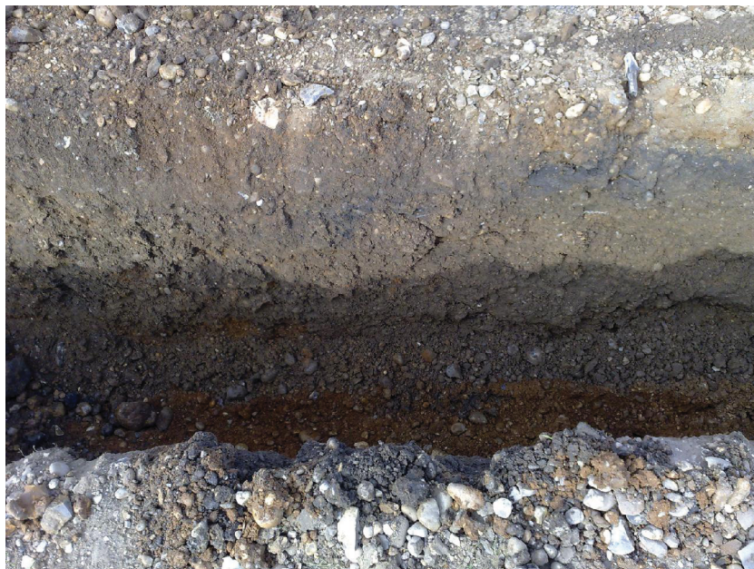
Plate 3 Close-up of pipe trench walls showing backfill of other pipe cuts, looking south
