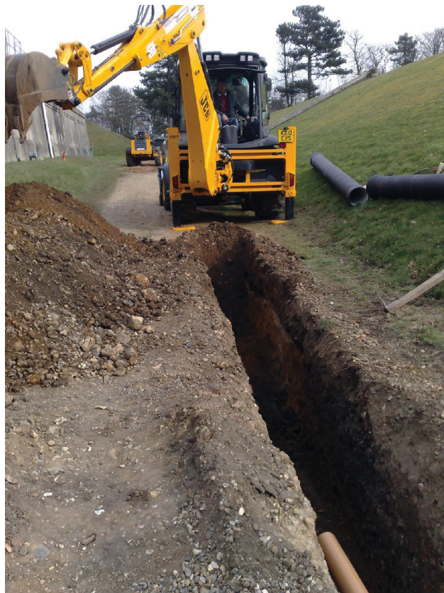
Plate 1 Machining the pipe trench, looking west
