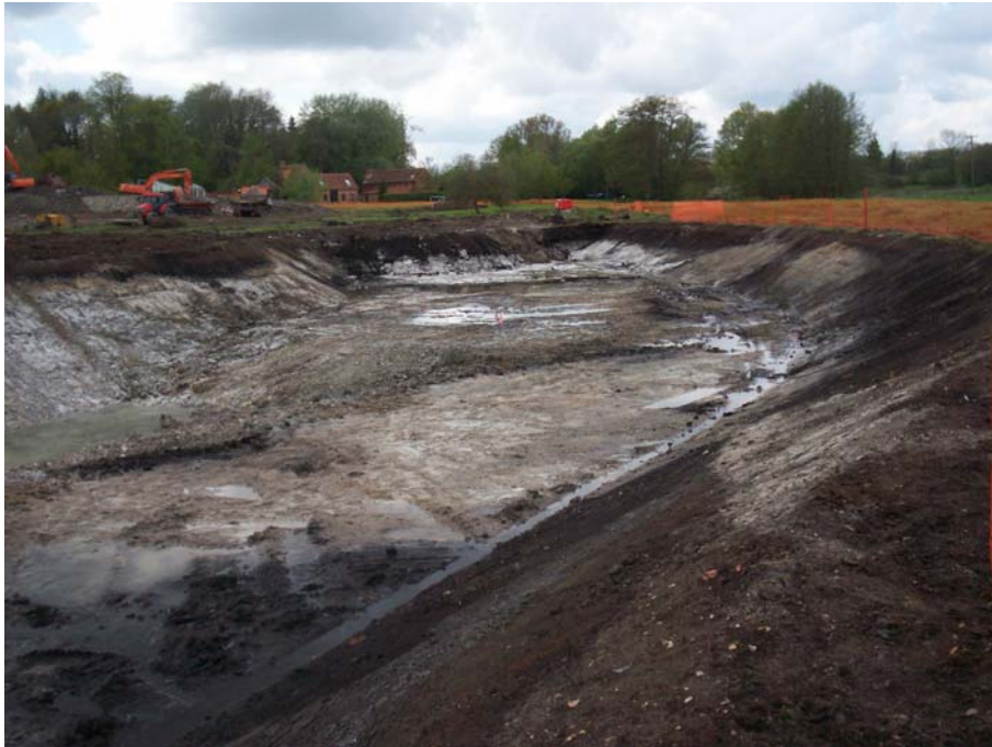
Plate 1: The lake during excavation, facing southwest
