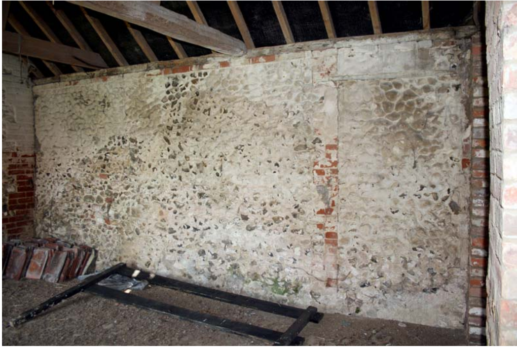
Plate 3. Blocked northern door way in eastern cell of Building B1
