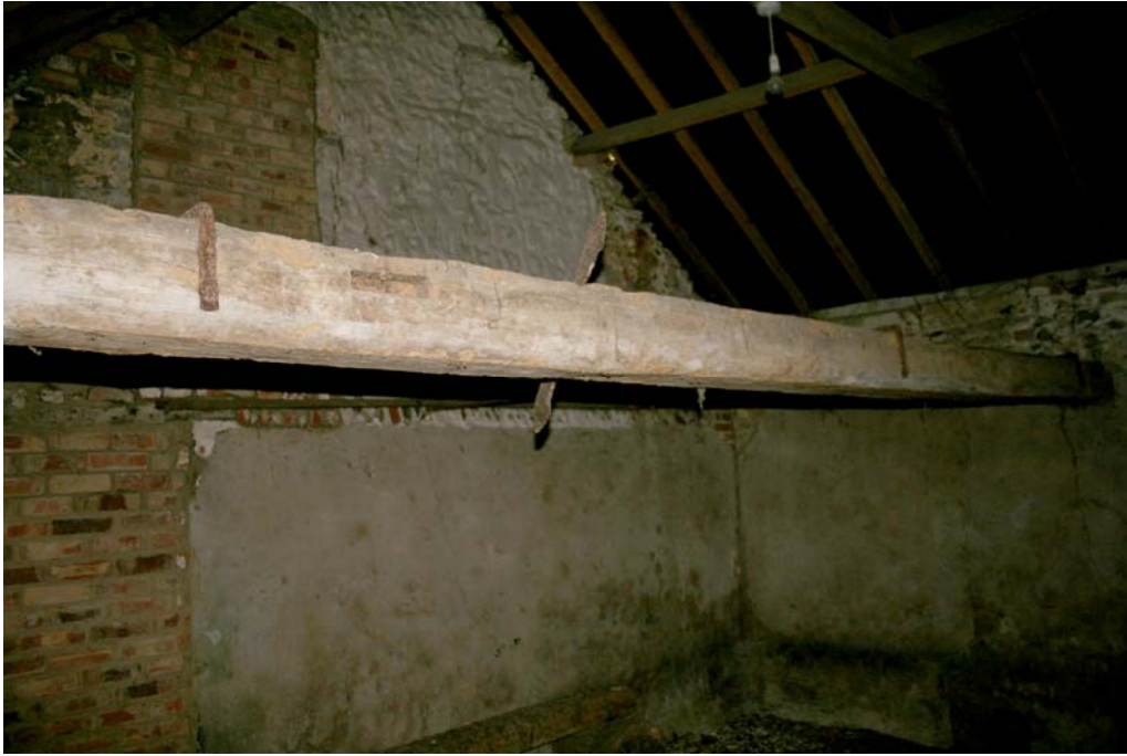
Plate 12. Cross joist for upper floor, northern cell of Building B2
