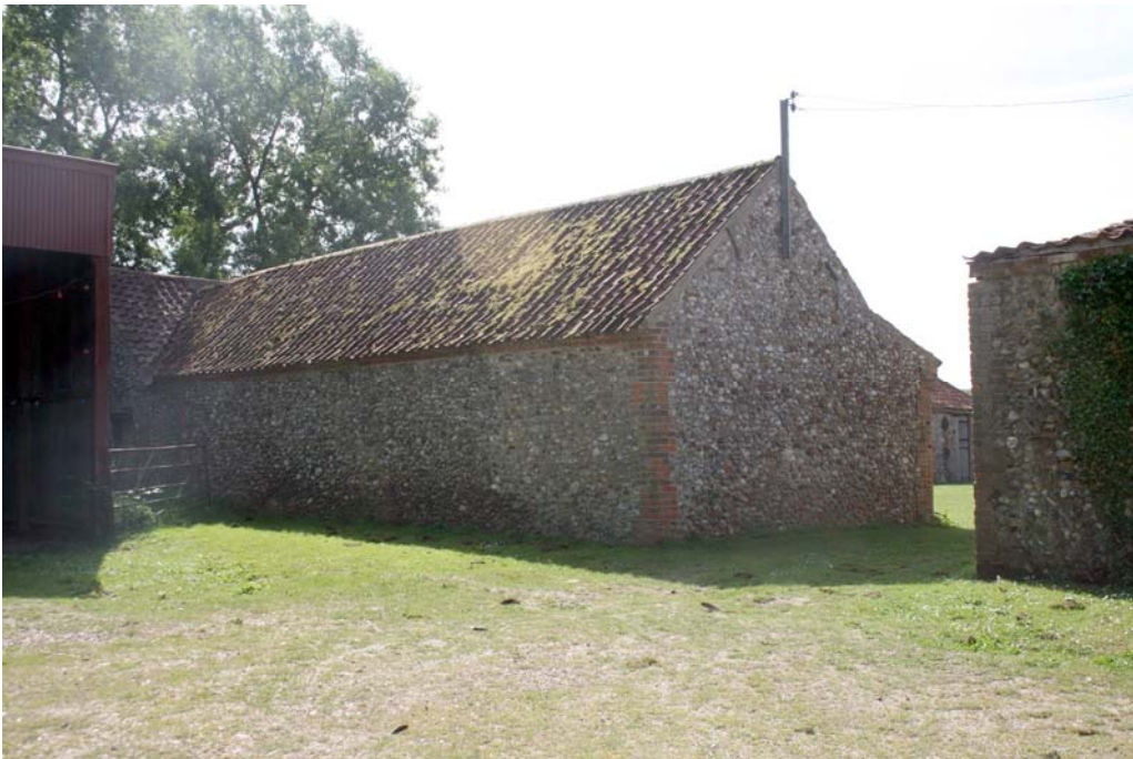
Plate 2. West gable and northern elevation of Building B1
