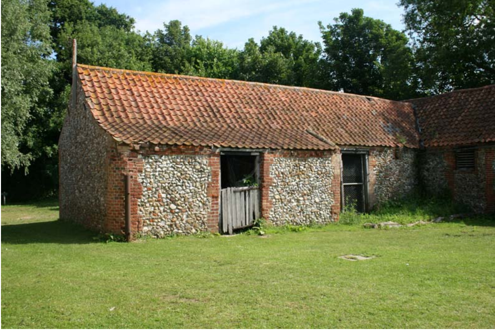
Plate 1. South elevation of Building B1
