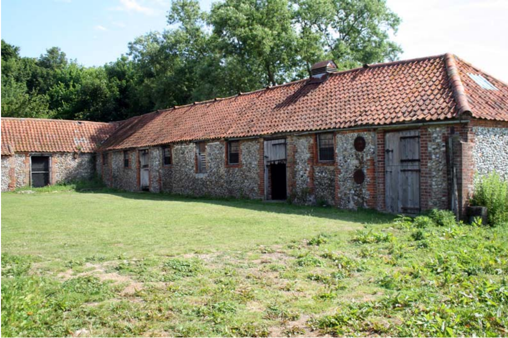
Plate 7. Western elevation of Building B2
