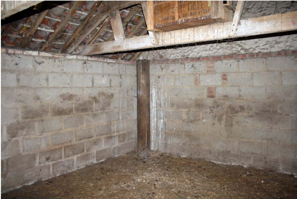
Plate 25. Tethering post in building B3
