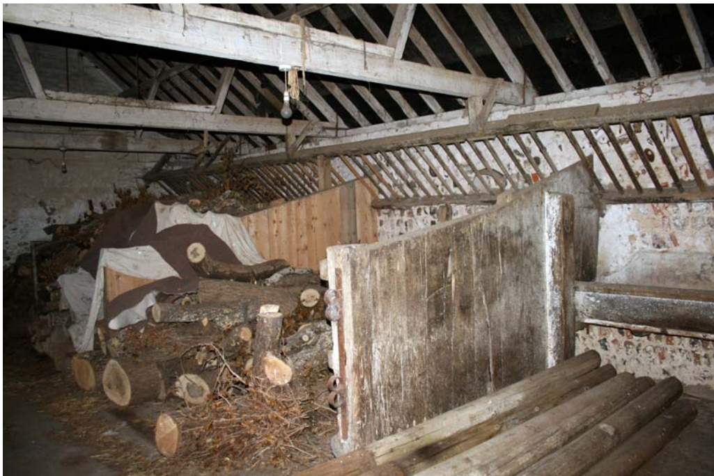
Plate 15. Central cell of Building B2 facing north
