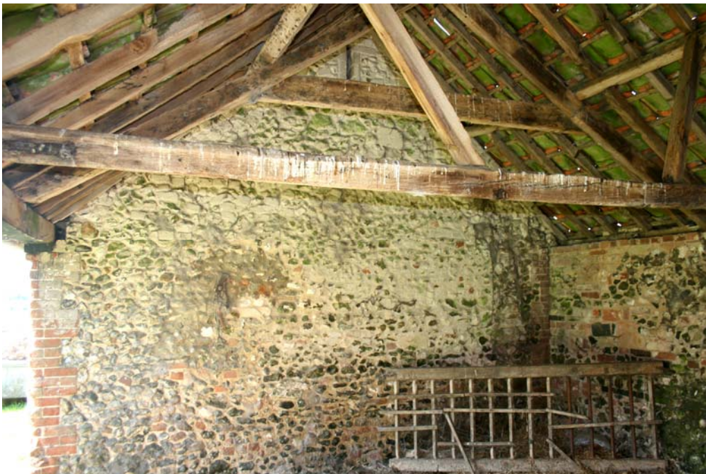
Plate 26. Interior of building B3, northern cell facing south
