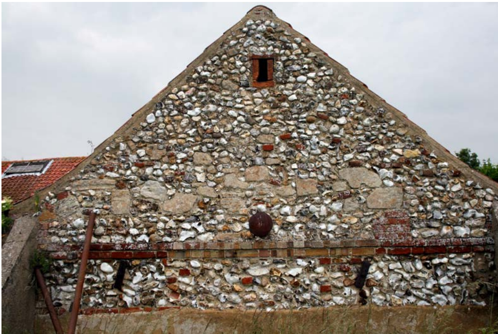
Plate 24. Ventilation hole south elevation building B3
