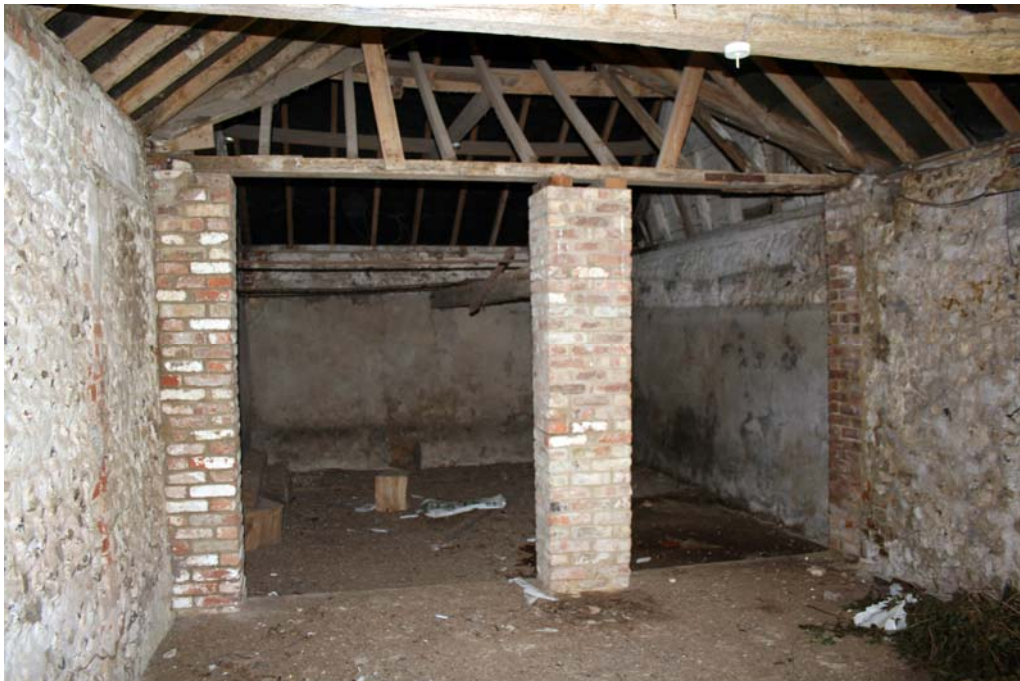
Plate 4. Modern brick piers dividing eastern cell of Building B1 from building B2
