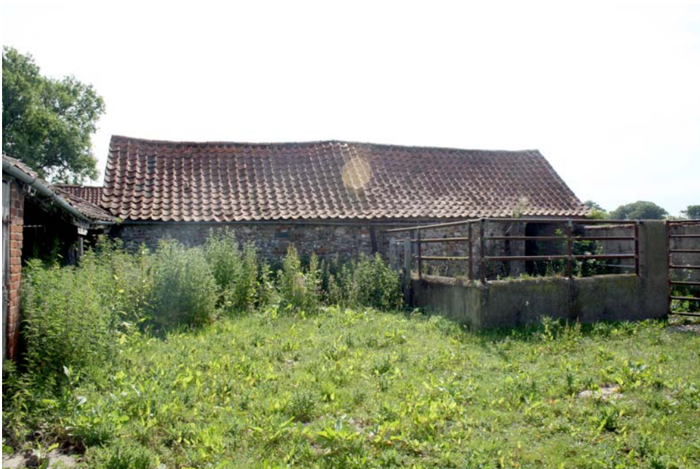
Plate 22. Western elevation of building B3, doorway to right
