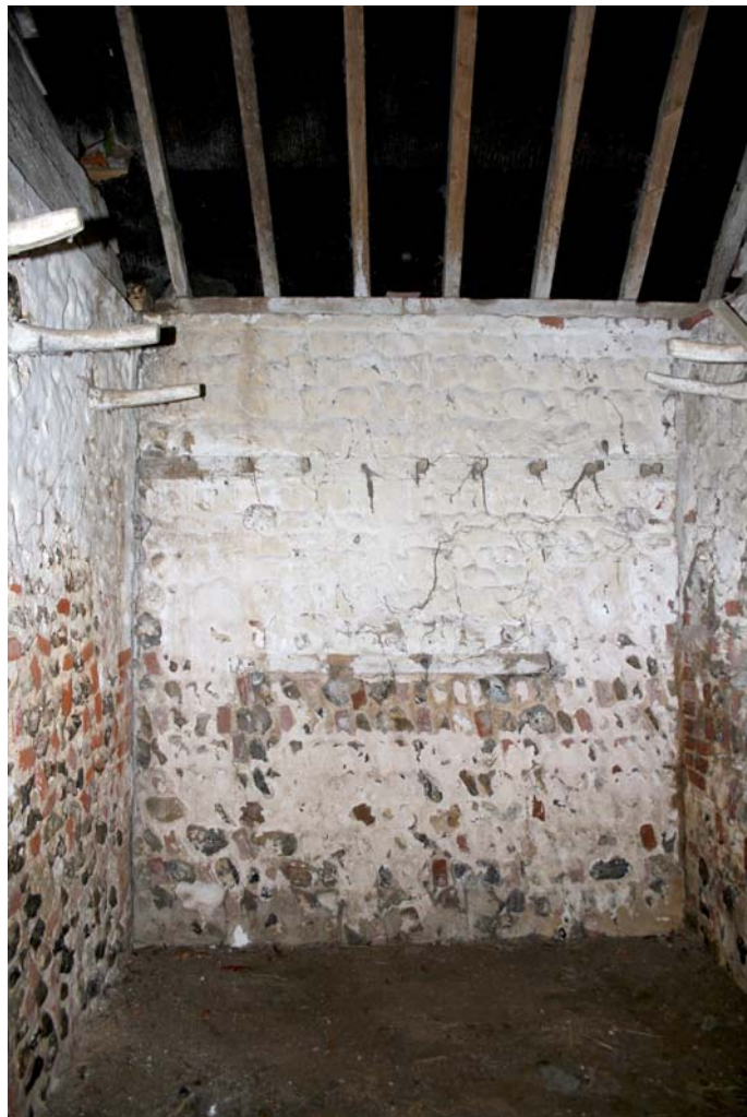
Plate 13. Tack room in Building B2
