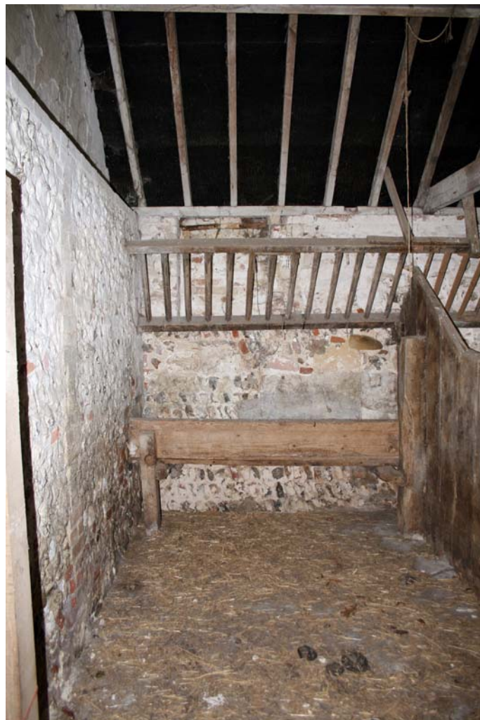
Plate 10. Blocked window behind hay rack on eastern wall of Building B2
