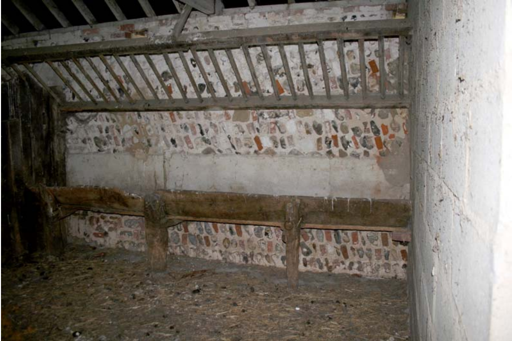
Plate 8. Eastern internal elevation of Building B2
