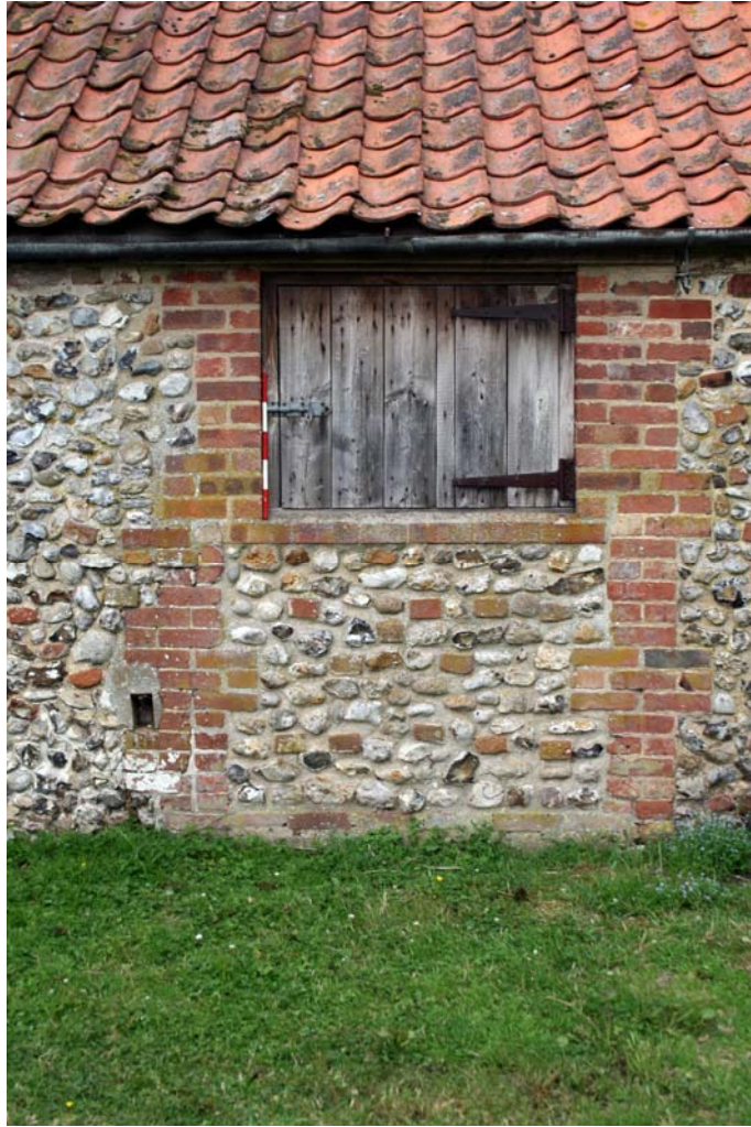
Plate 23. Doorway converted into window on eastern elevation of building B3
