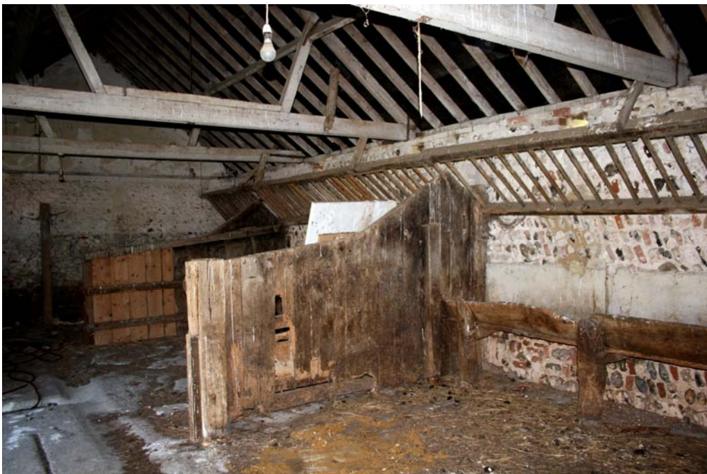
Plate 17. Second-most southerly cell, Building B2 facing north
