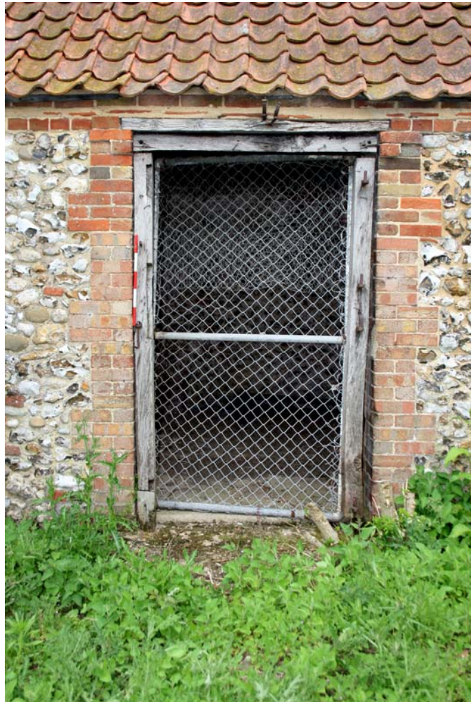
Plate 27. Southern doorway, eastern cell Building B1
