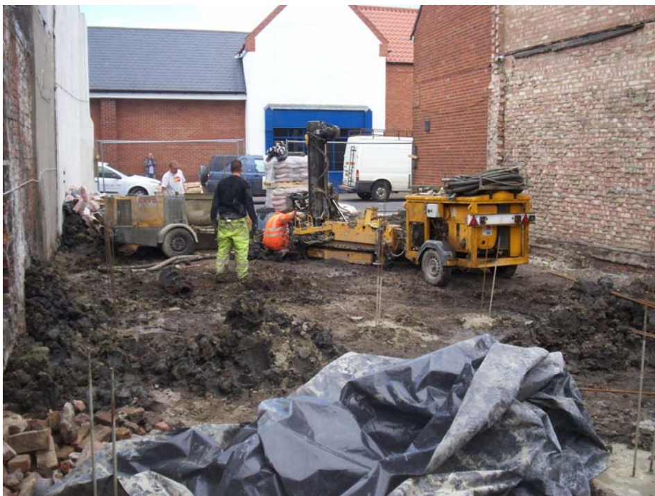
Plate 1. The piling operation in progress, facing north
