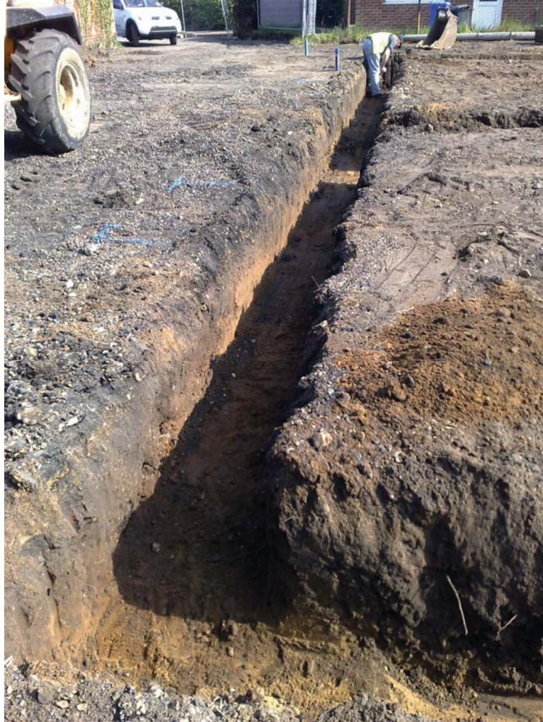
Plate 2 Close up of foundation trenches, looking south
