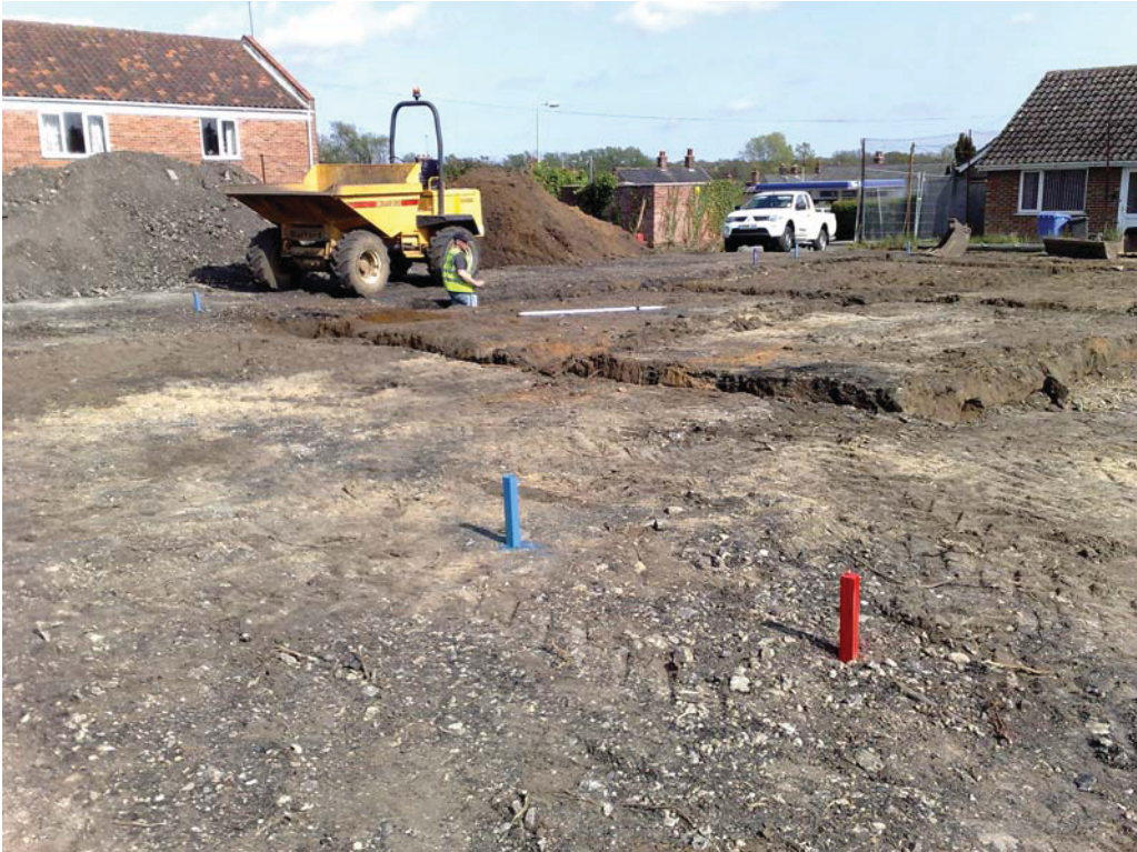
Plate 1 The site, looking south
