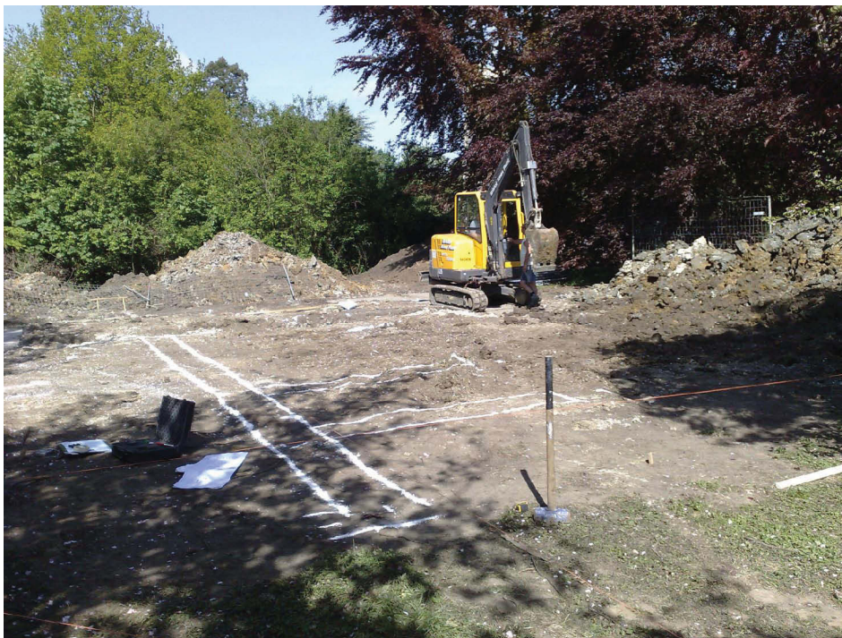
Plate 1. The site, looking north-west
