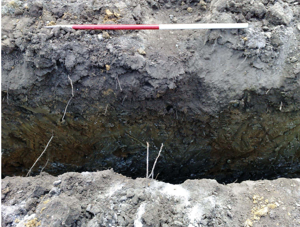
Plate 3. Close up of the foundation trench edge, looking north
