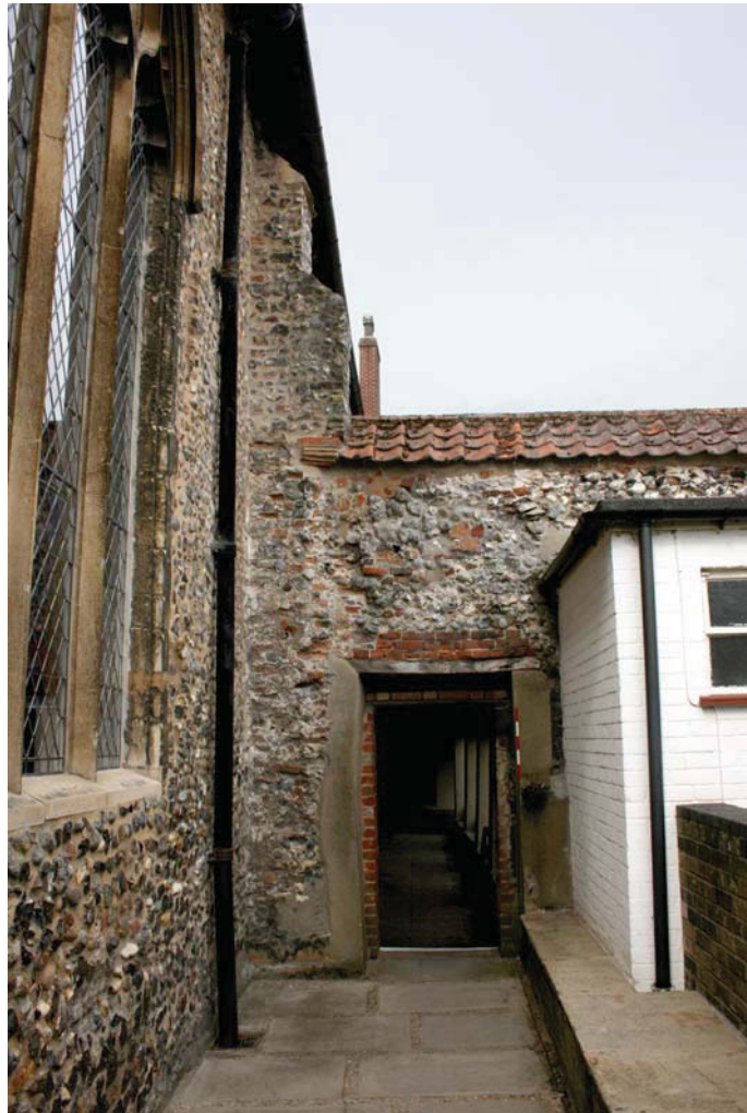
Plate 4 View of buttress facing west
