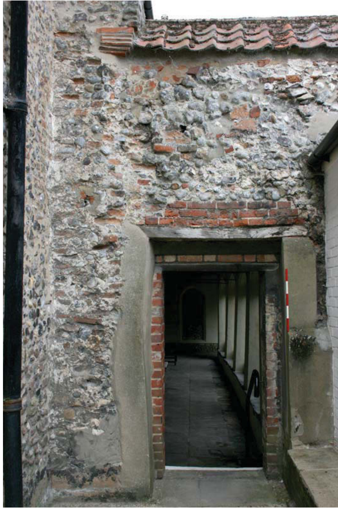
Plate 5. East side of opening facing west, 1m x 0.20m scale
