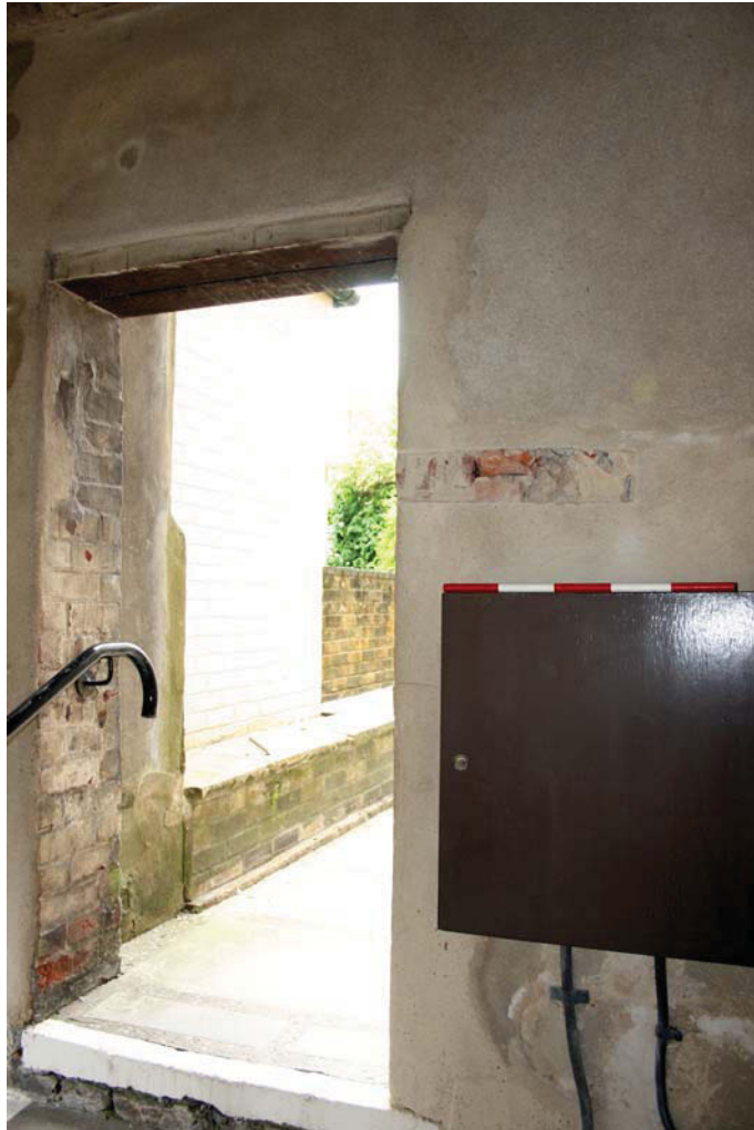
Plate 1. Plaster removed from interior, facing east, 1m x 0.20m scale
