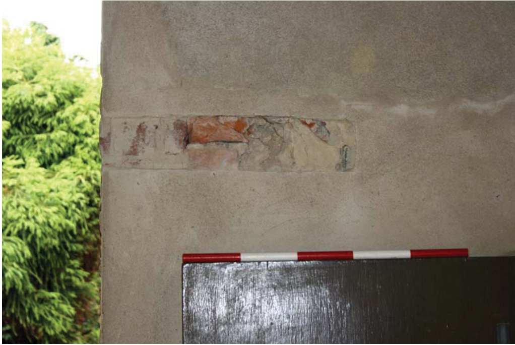
Plate 2. Close up of removed plaster, 1m x 0.20m scale
