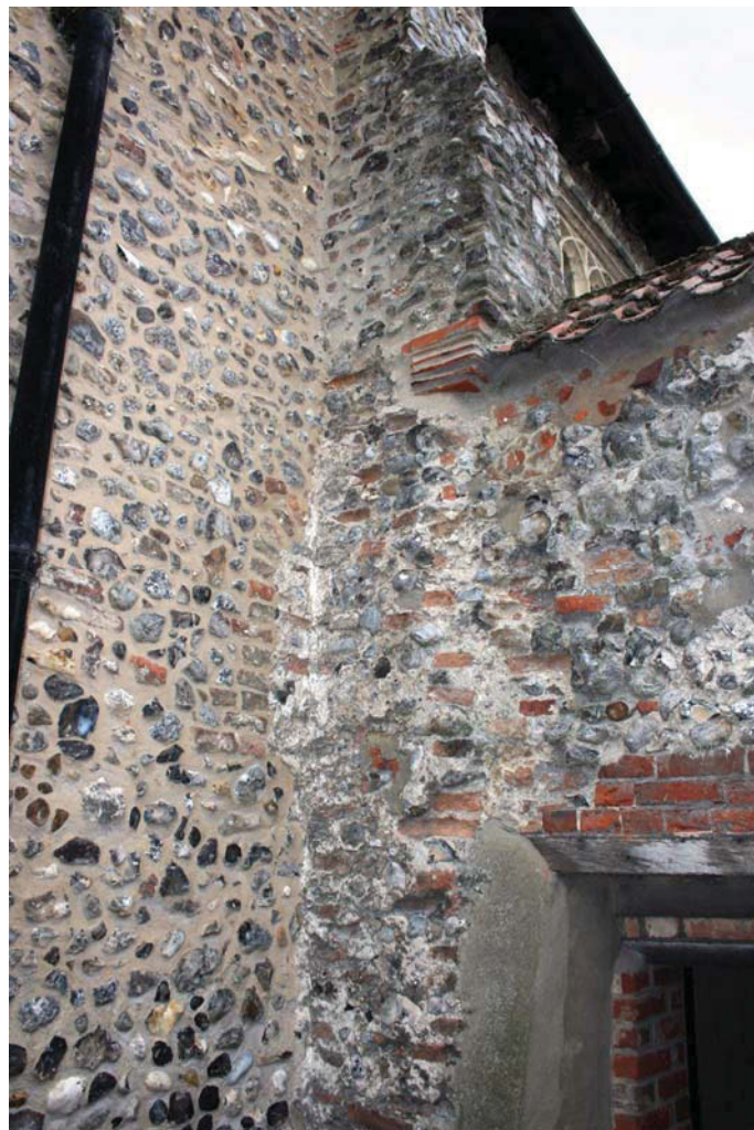
Plate 3. Blocked window obscured by later buttress
