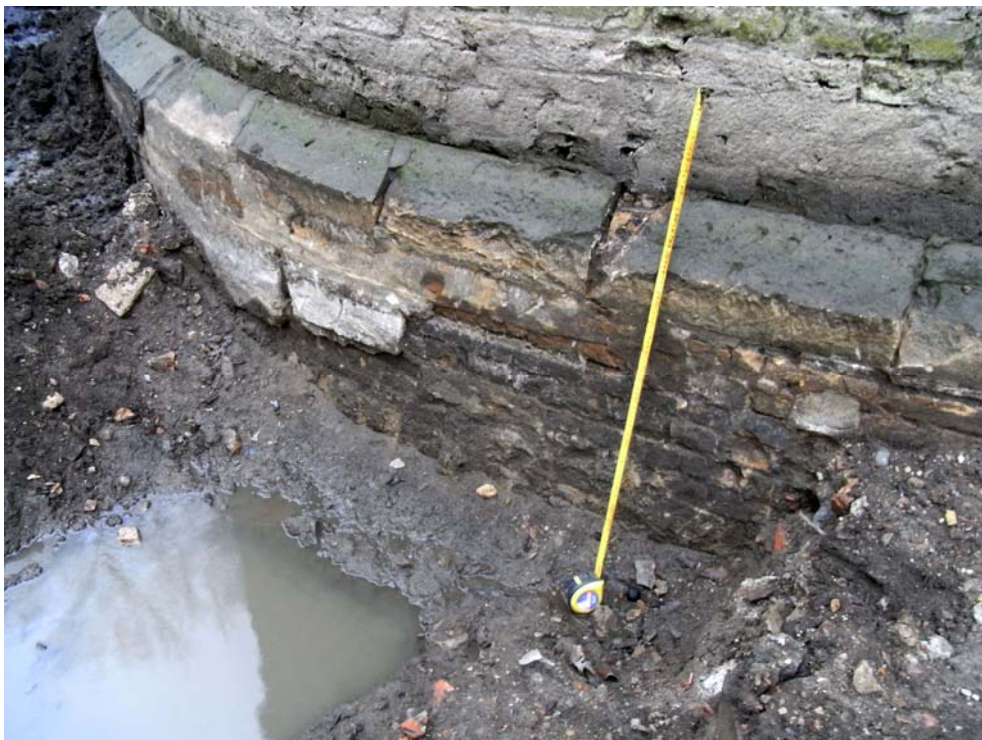
Plate 16. Brickwork at base of tower
