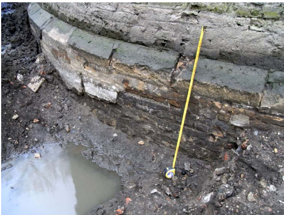
Plate 16. Brickwork at base of tower
