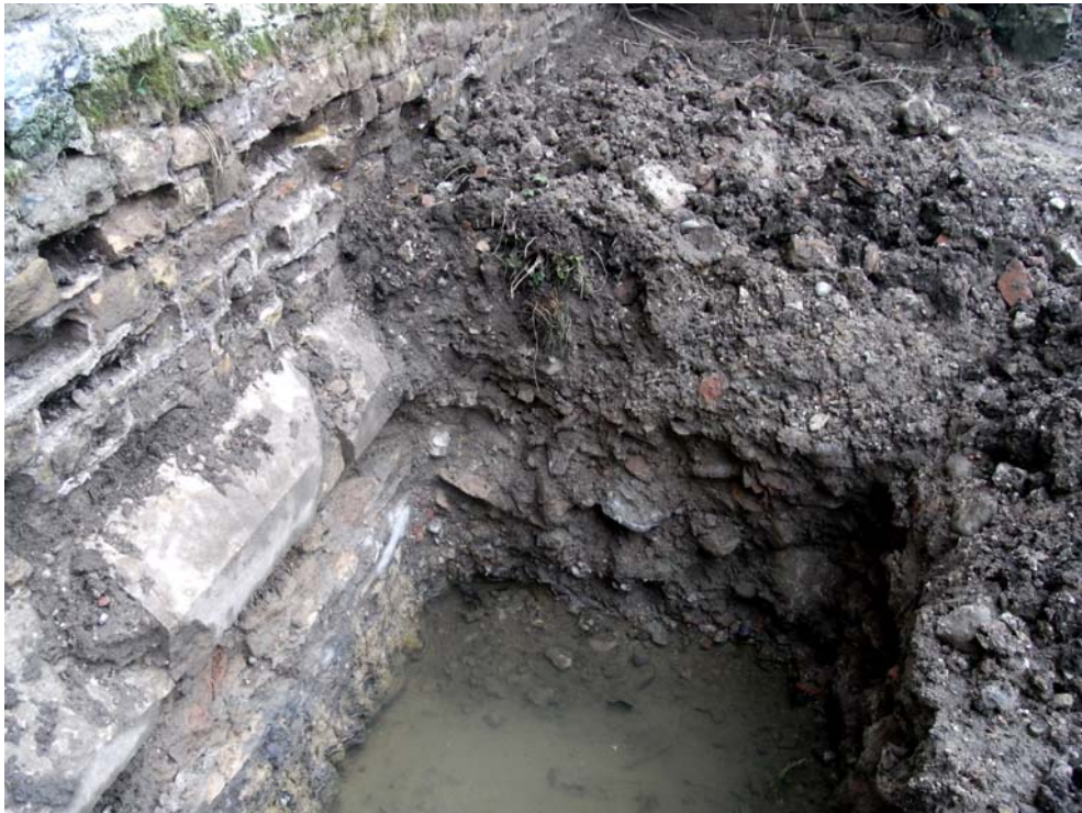
Plate 15. Test pit 3 (demolition rubble)
