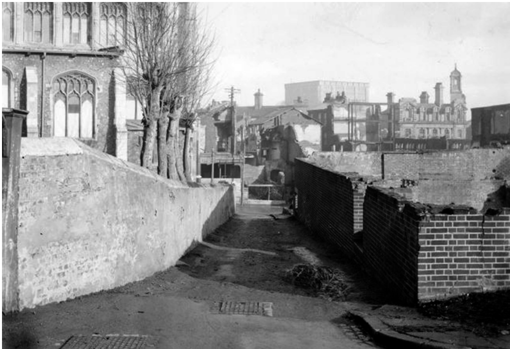
Plate 2 St Stephens Street (now Malthouse Lane) looking north at demolished buildings
