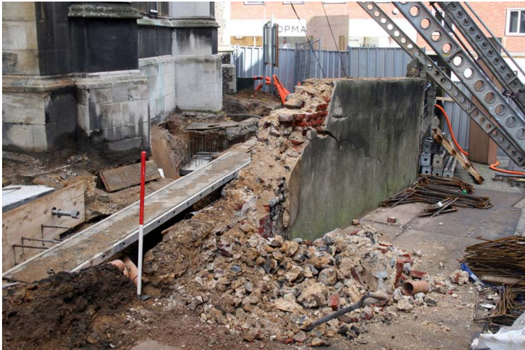
Plate 4. Wall during demolition, looking north-west, 1m scale
