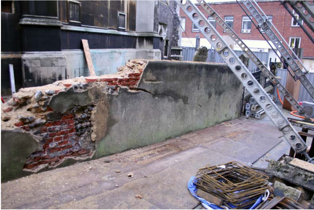
Plate 5. Wall during demolition looking north-west, with cobble panel within brickwork
