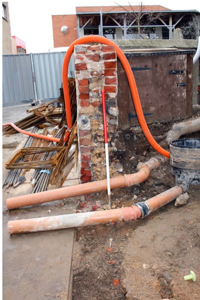
Plate 3. South end of wall, looking south, 1m scale. Image shows flint rubble core, later brick facing and repair
