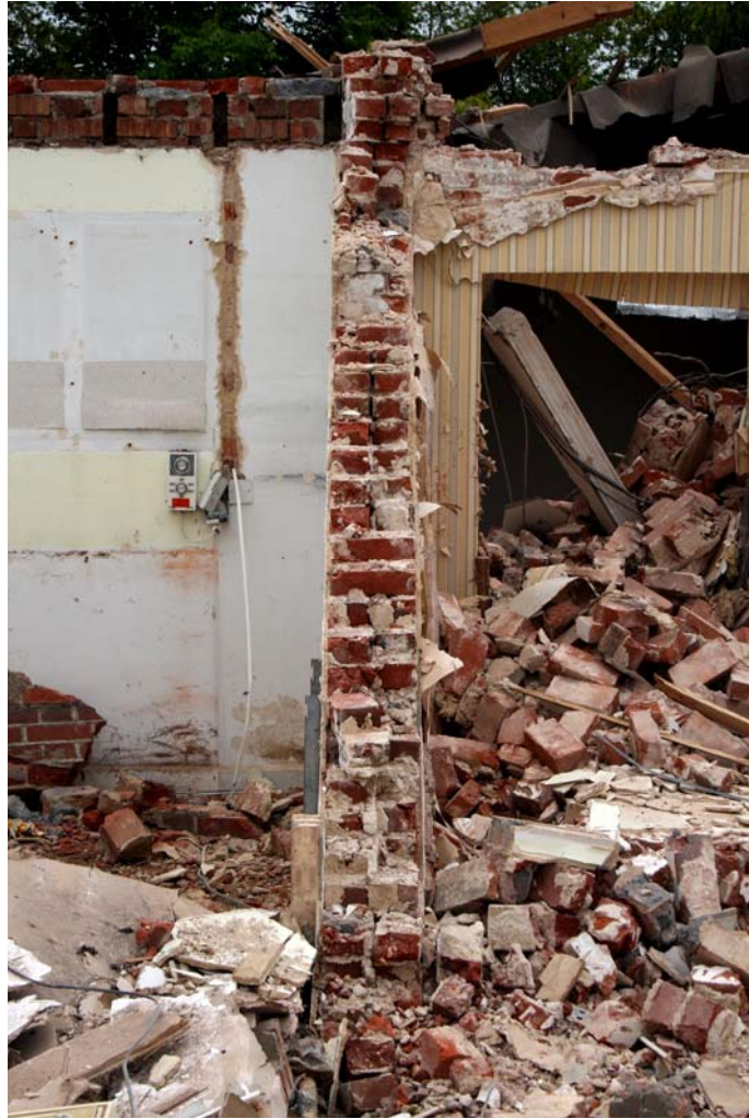
Plate 17. Construction of internal wall during demolition
