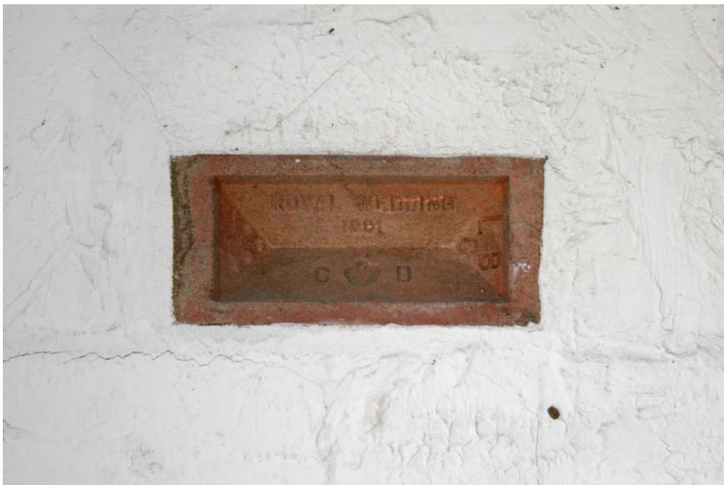
Plate 4. Commemorative brick in rear porch
