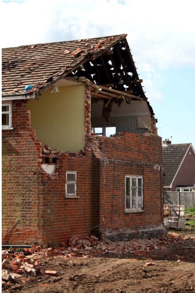
Plate 16. North-western elevation during demolition
