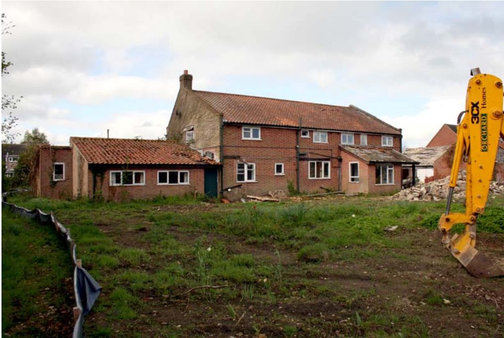
Plate 2. North-eastern elevation and south-east gable, facing west
