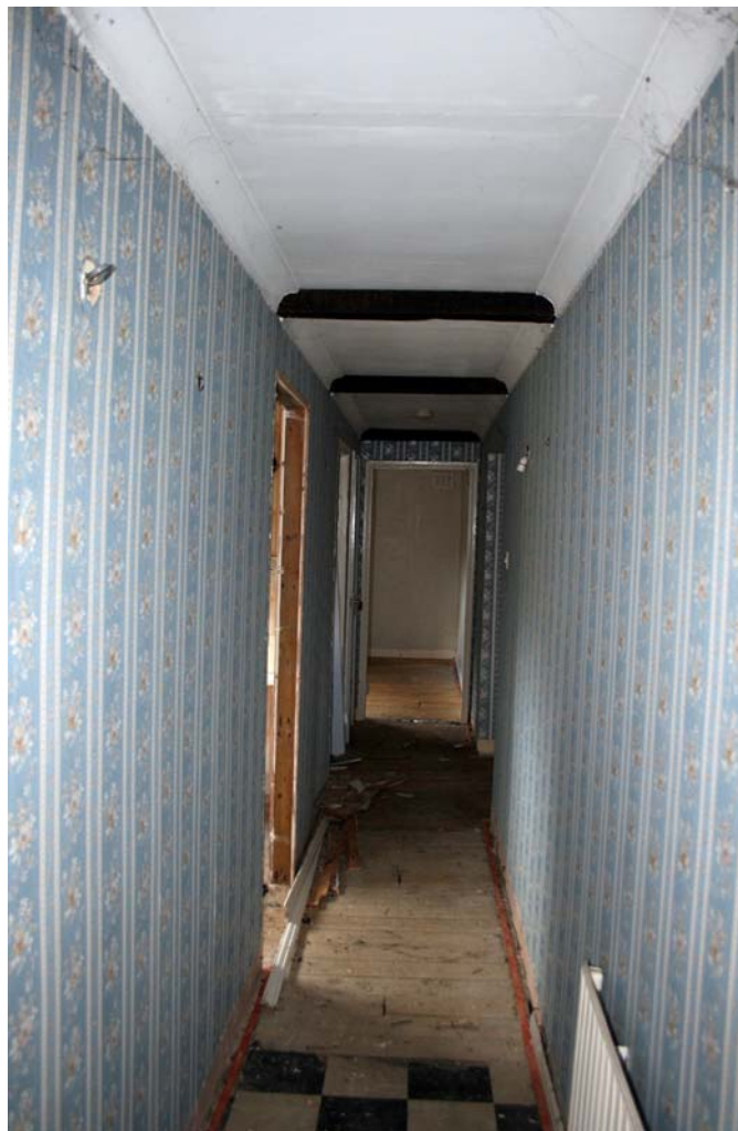
Plate 15. Upstairs corridor facing south-east
