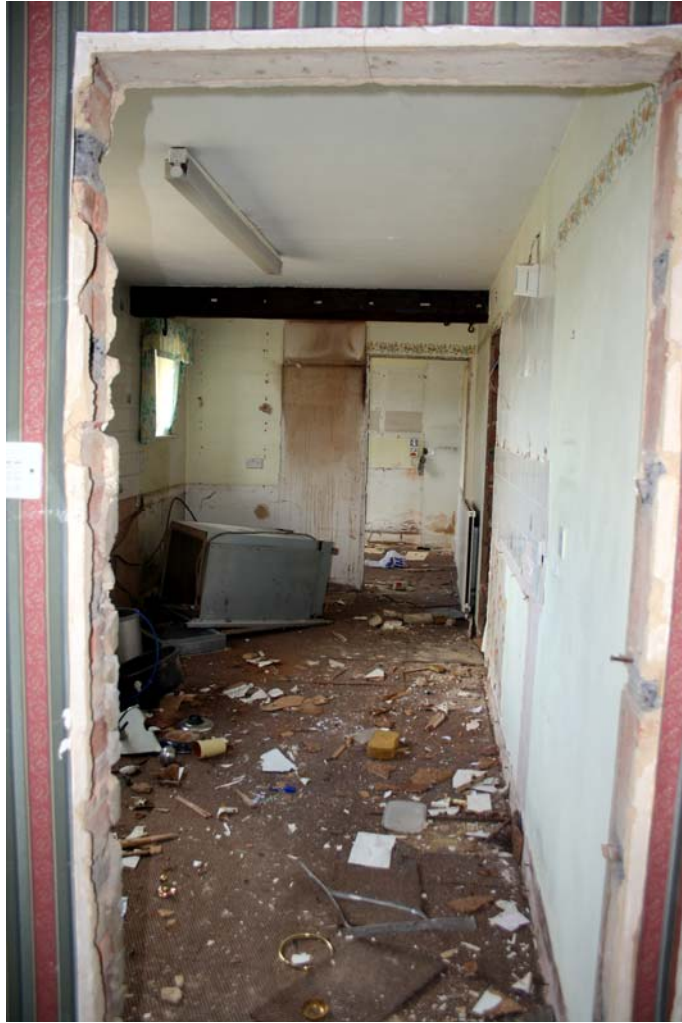
Plate 11. Kitchen with laundry room beyond, facing south-east
