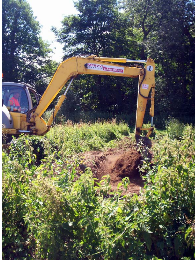
Plate 2. General view, looking south
