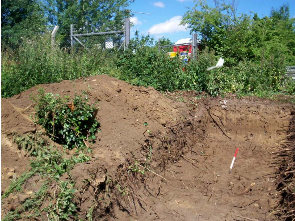
Plate 1. General view, looking north
