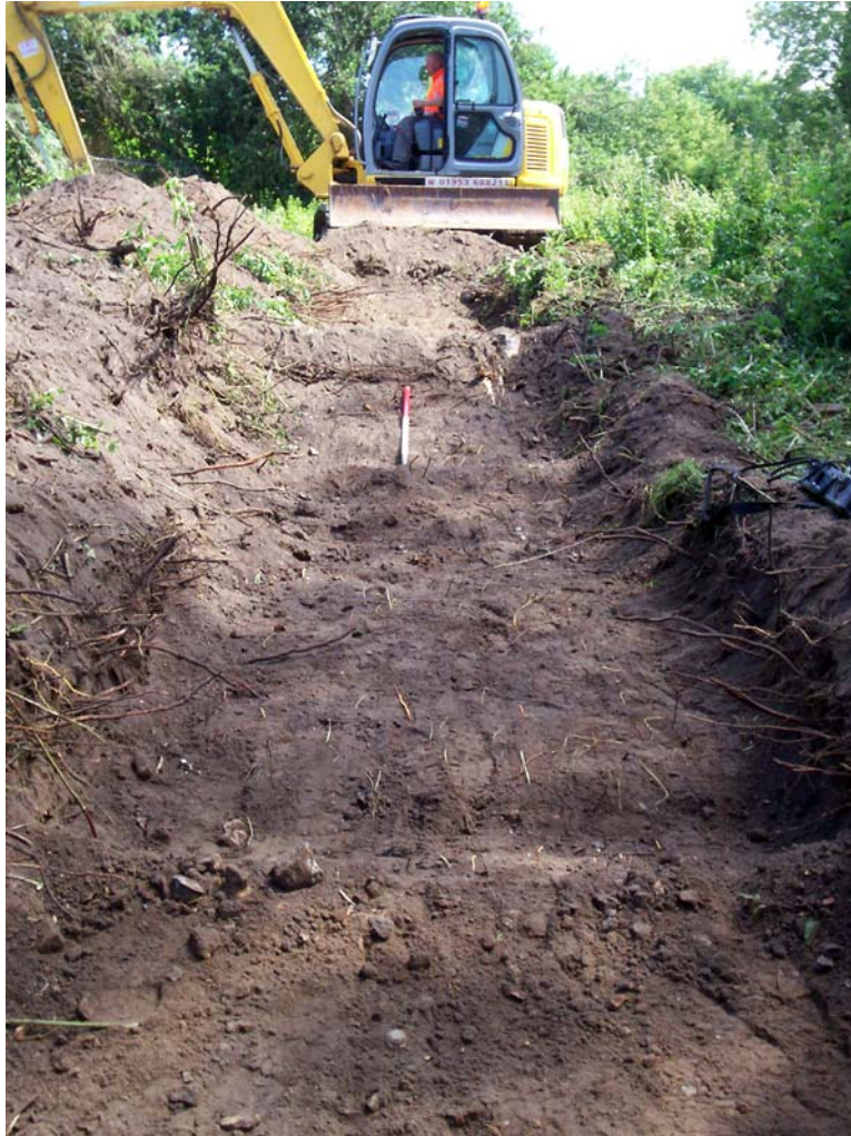
Plate 5. Area 2, looking north-east
