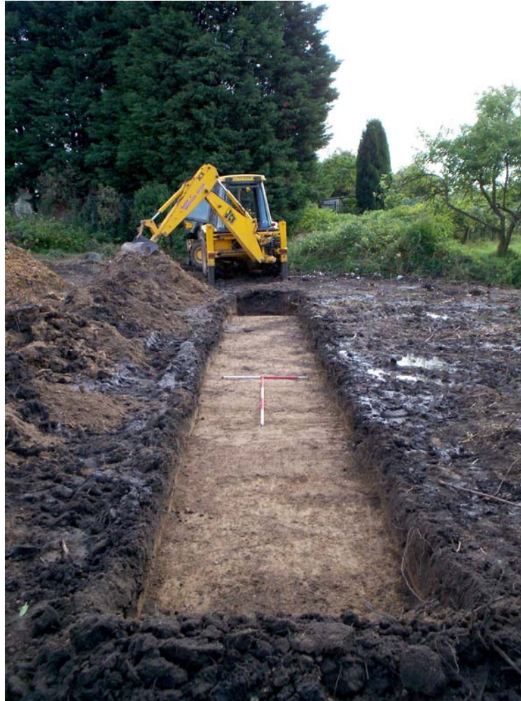
Plate 1. General view of trench, facing east
