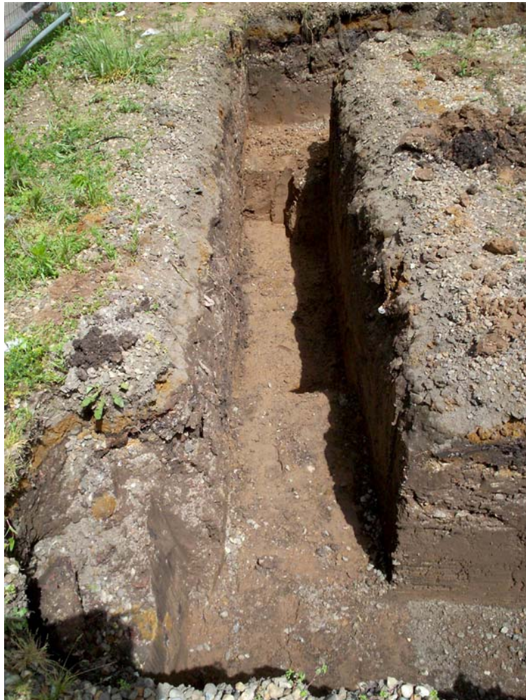
Plate 2 A view of the westernmost trench, looking north
