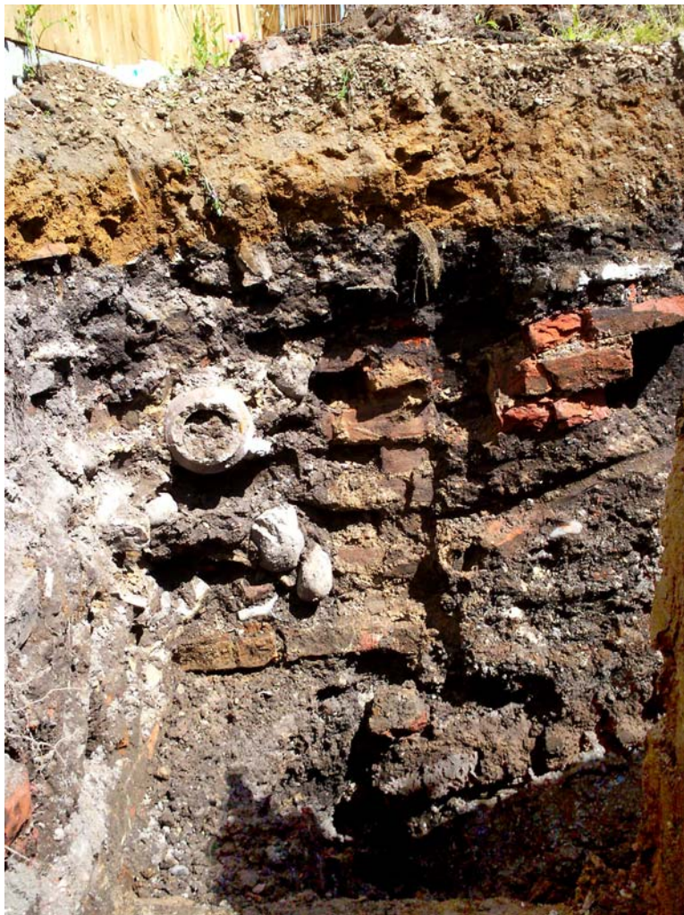
Plate 4. Remains of the probable Victorian wall <15> and ceramic pipe (fill (17)) in the north-eastern corner of the foundations
