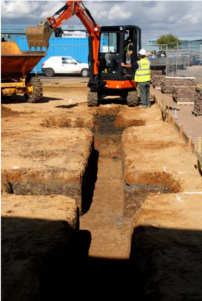
Plate 1. Trench 3, looking north-west
