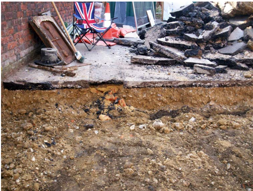
Plate 6. Trench 2, north-facing section
