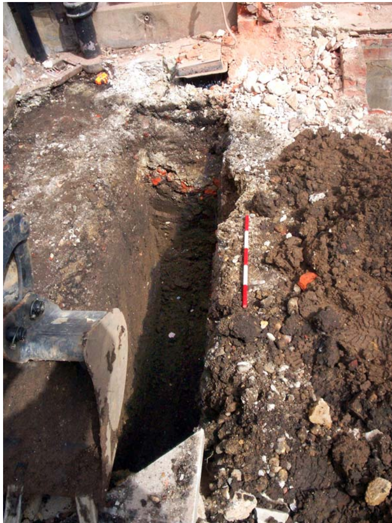
Plate 1. Test trench 1, looking north
