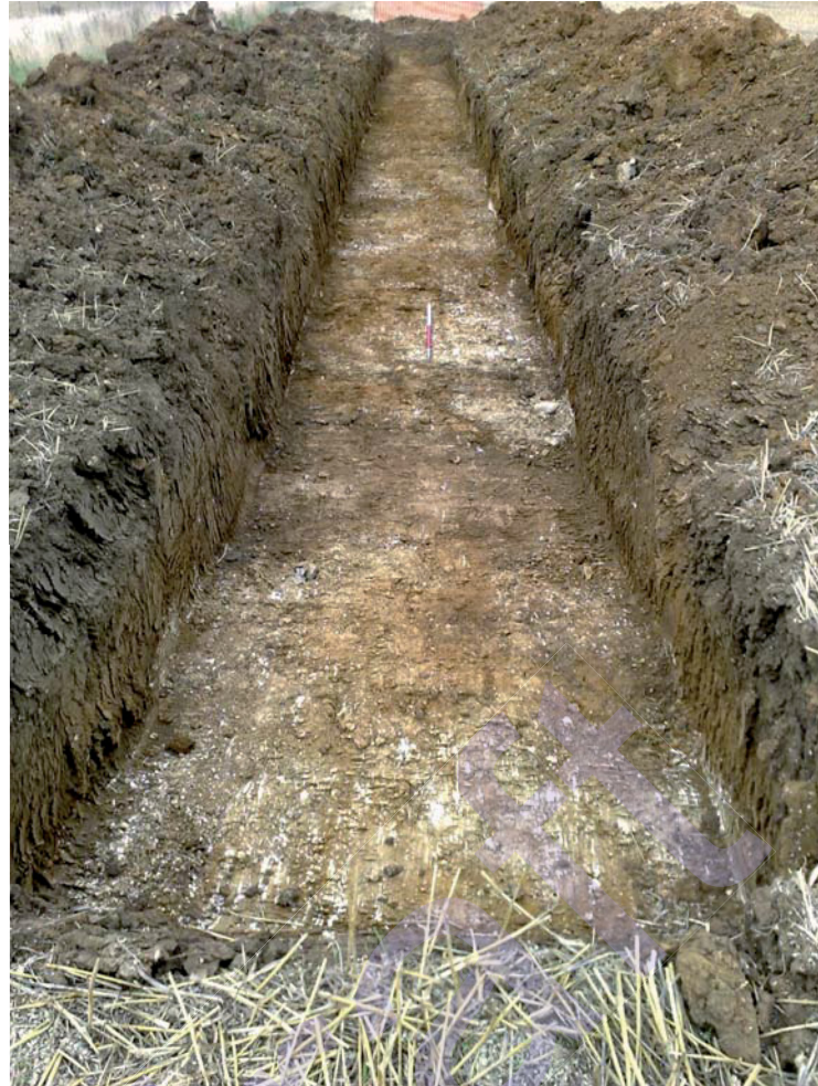
Plate 9. Trench 5, pre-excavation, looking north
