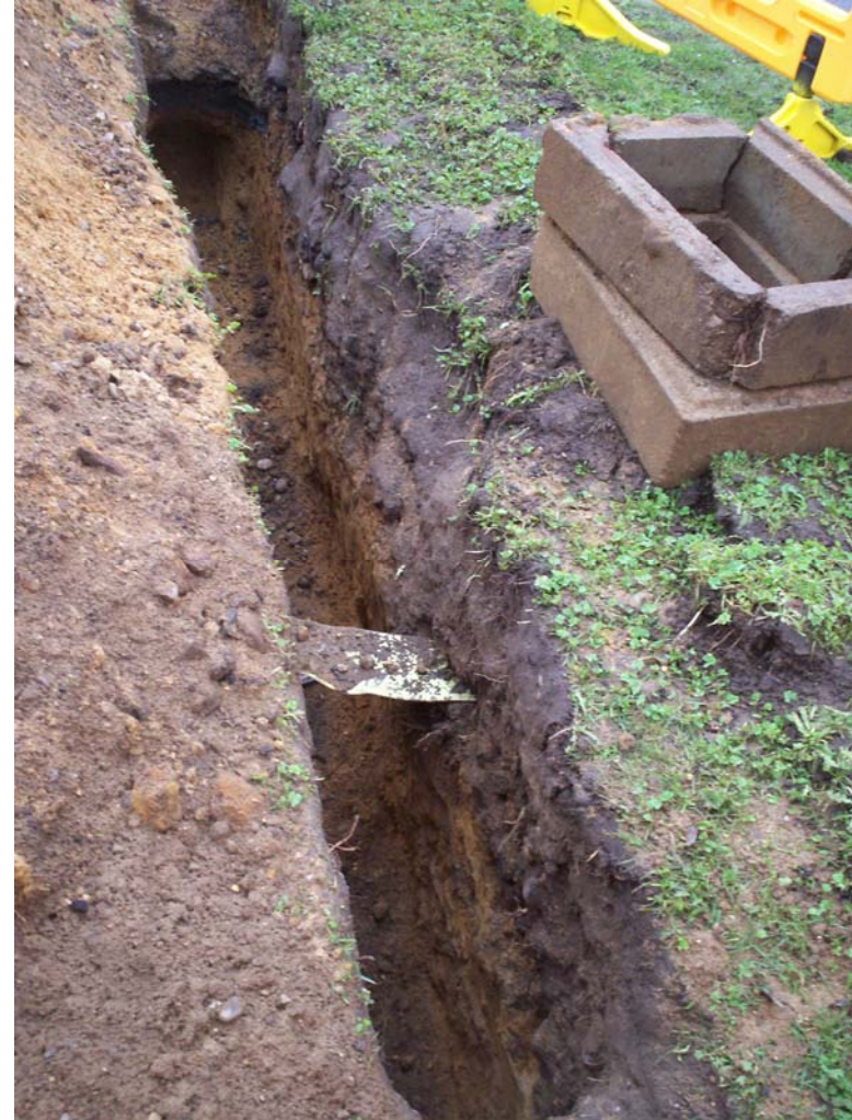
Plate 8. The north end of the roadside trench – at Bridge Foot Corner
