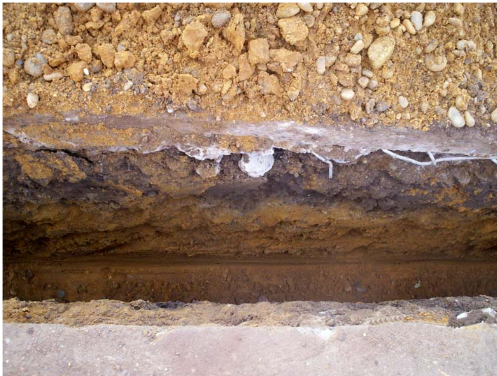
Plate 5. Deposits in the roadside trench
