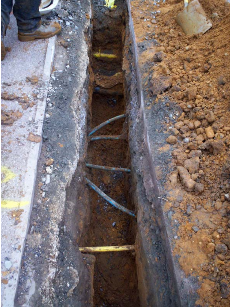
Plate 7. Modern services in the trench beside Might's Road
