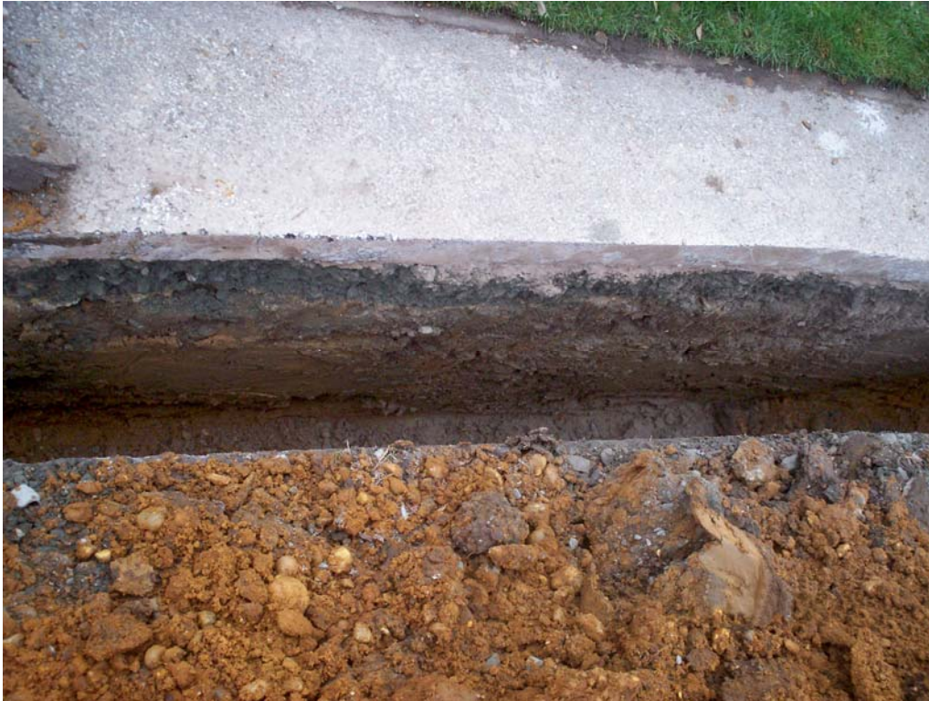
Plate 6. Deposits in the roadside trench
