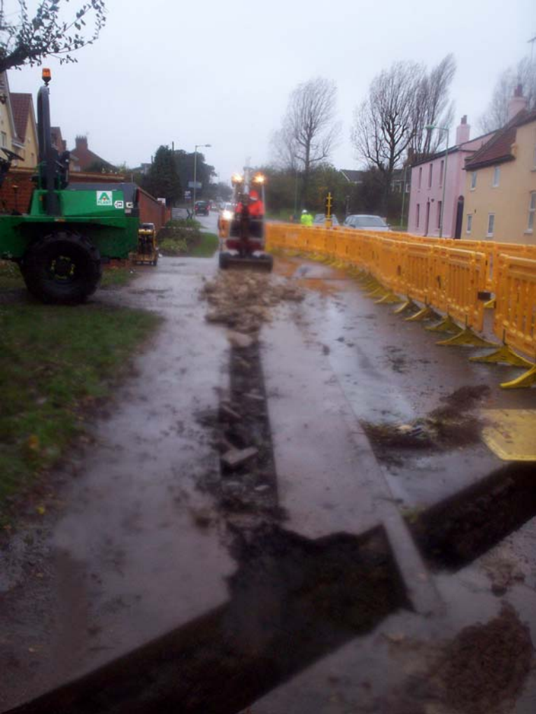
Plate 3. Looking north-west at work along the pavement beside Might's Road
