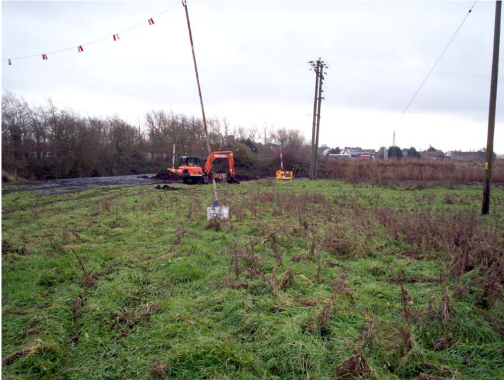
Plate 14. Excavation of Trench 4 (looking south-east)
