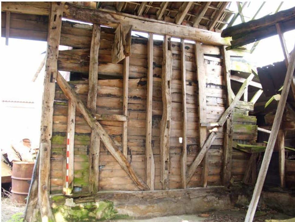
Plate 4. North wall with reused stud, 1m scale
