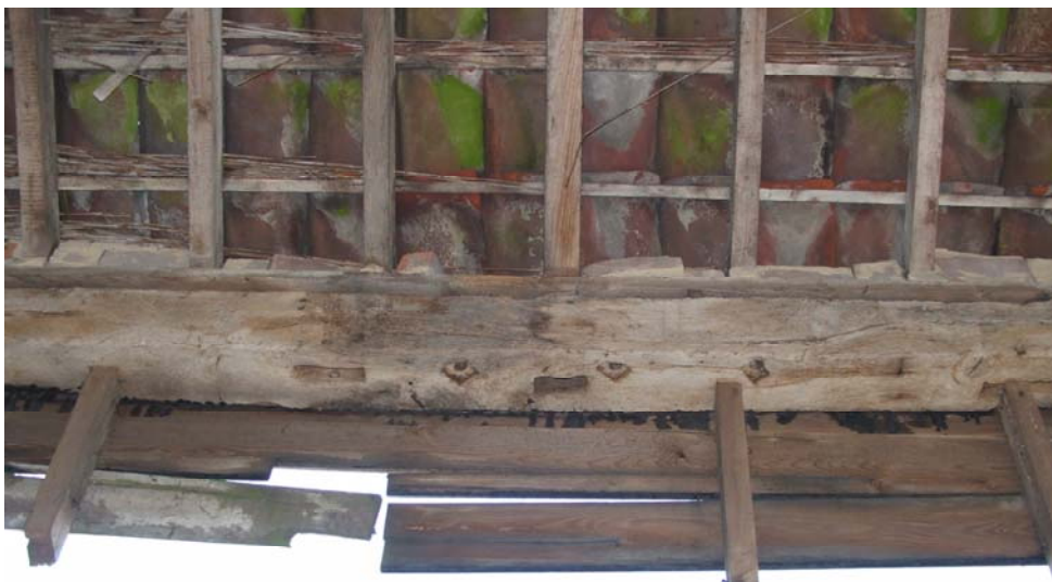
Plate 6. Wallplate with diamond mullion sockets over cart door, looking north-east
