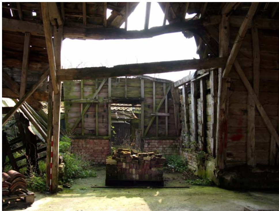
Plate 8. Porch looking south, 1m scale
