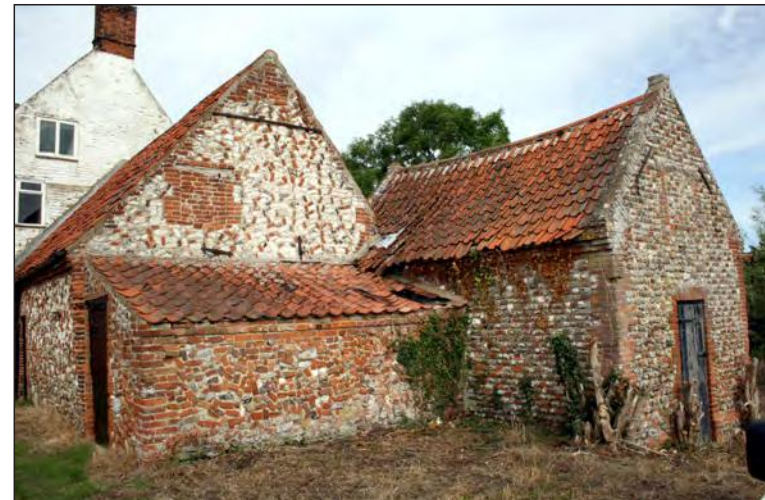
Plate 40. Building E east elevation
