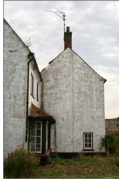
Plate 14. Western elevation of Building B
