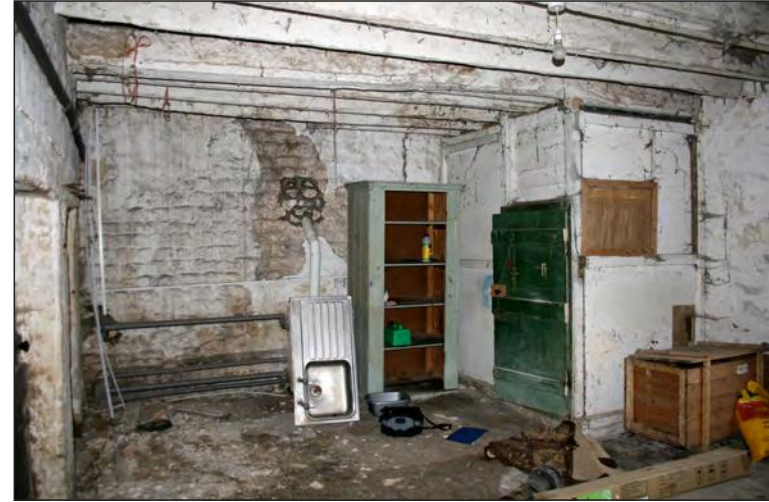
Plate 34. Interior of Building C, west end
