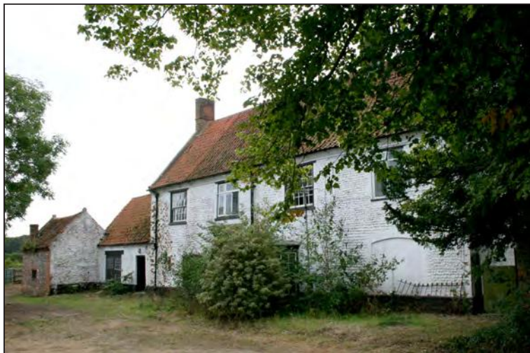
Plate 3. Building A north elevation facing south-east
