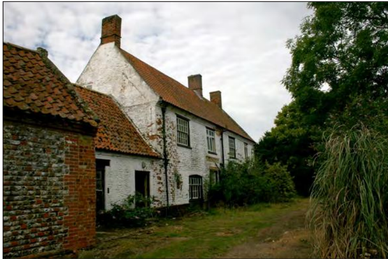
Plate 1. Building A, north elevation facing south-west
