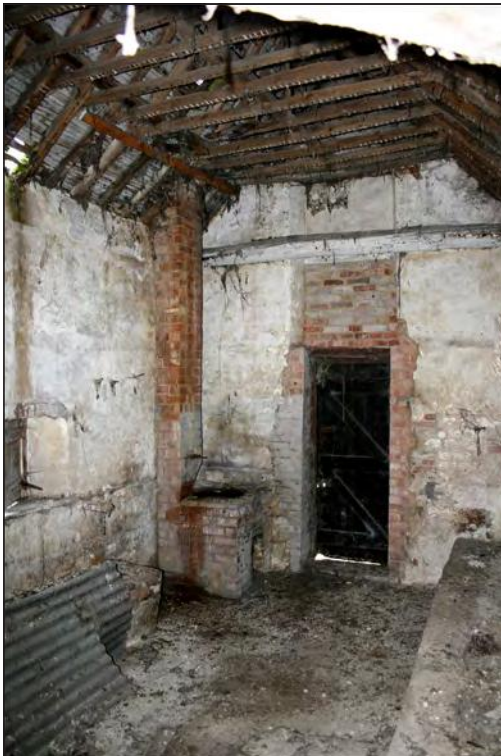
Plate 39. Interior of Building D
