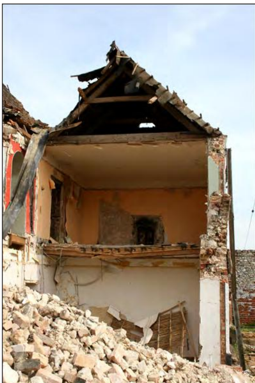
Plate 29. Construction of Building B's walls
