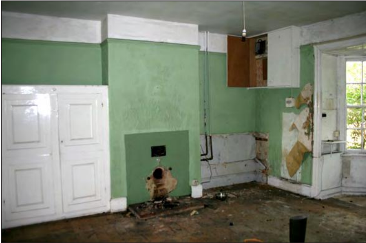
Plate 21. Central ground floor room, Building A
