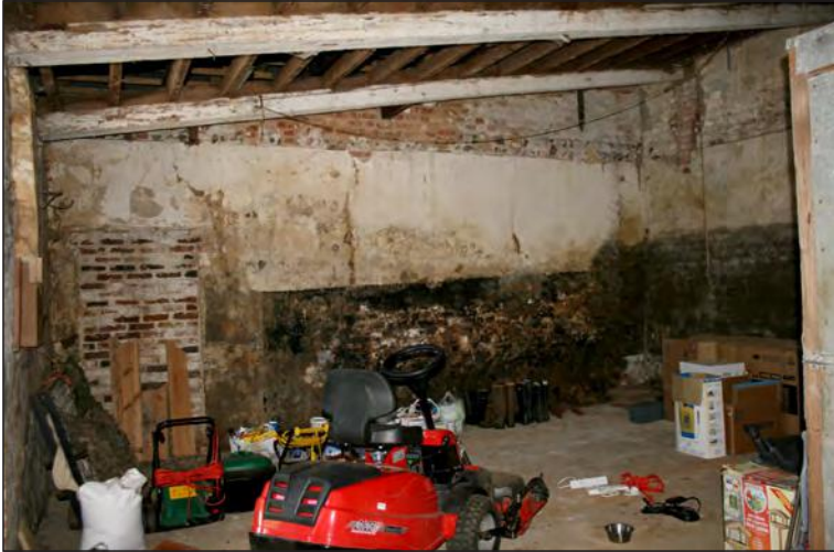
Plate 49. Interior of northern cell Building G
