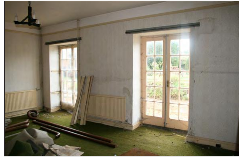
Plate 18. French windows, ground floor, Building B
