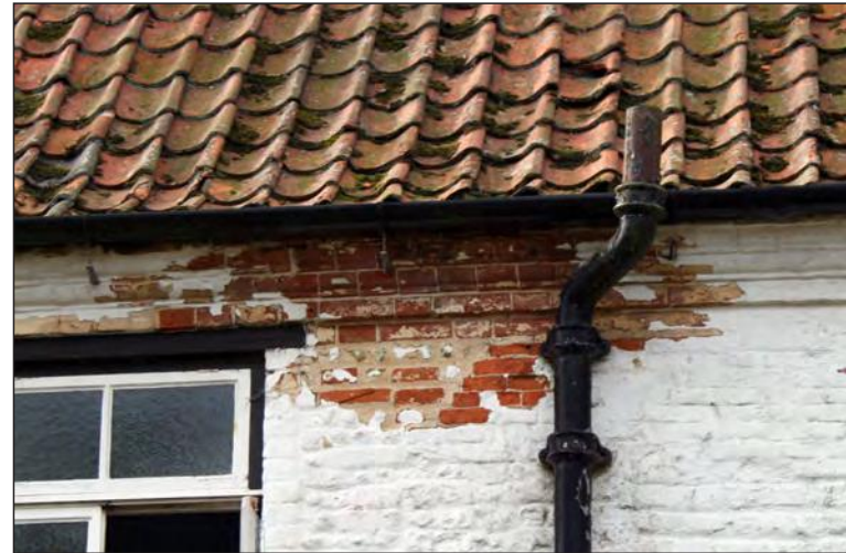
Plate 2. Moulded brick cornice on Building A north elevation
