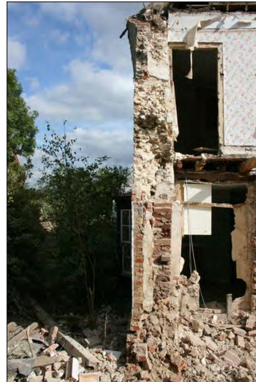
Plate 28. Construction of Building A's walls
