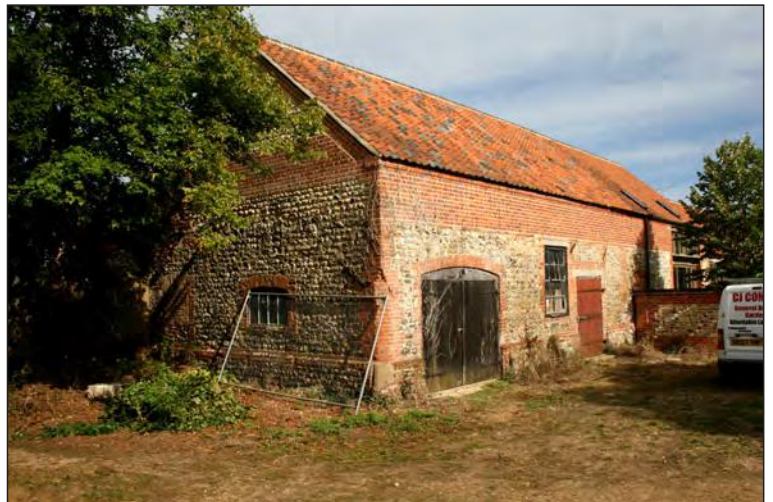
Plate 44. Building G facing north-west
