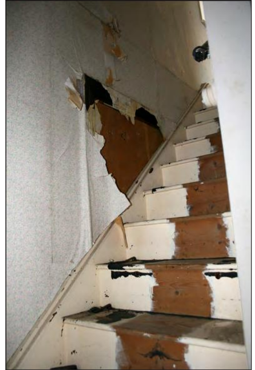
Plate 22. Blocked doorway formerly leading into Building B
