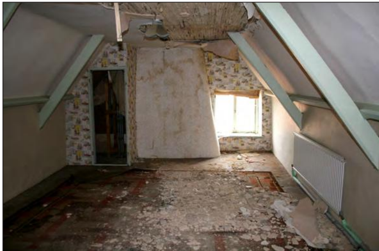
Plate 27. Second floor east bedroom
