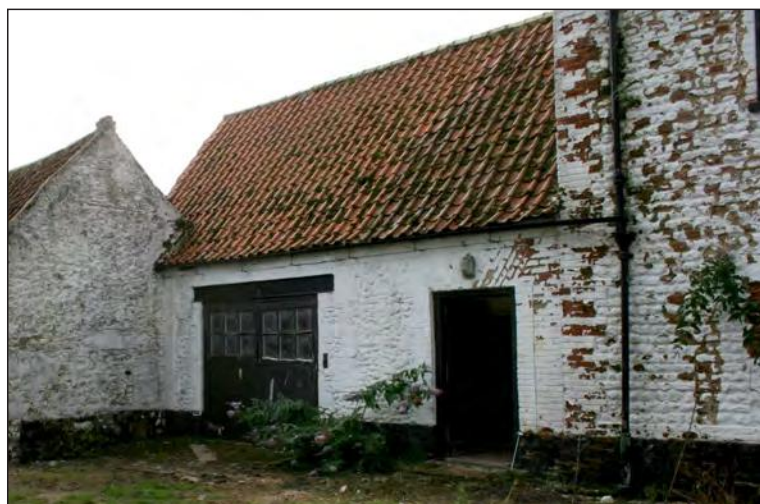
Plate 31. Building C north elevation
