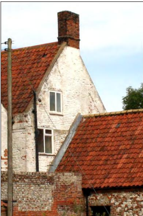
Plate 11. East gable of Building A showing tumble-in detail at eaves
