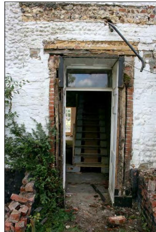
Plate 4. Front door with porch surround removed
