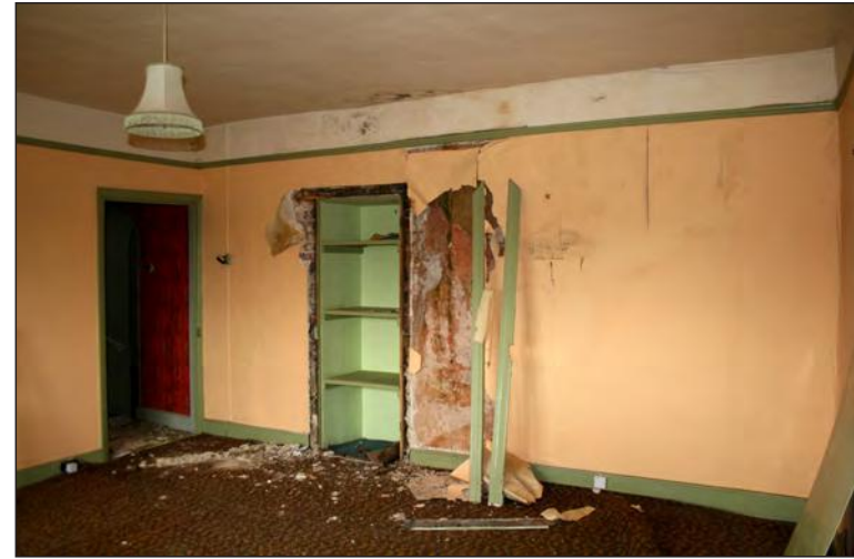
Plate 26. Niche indicating previous doorway in Building A
