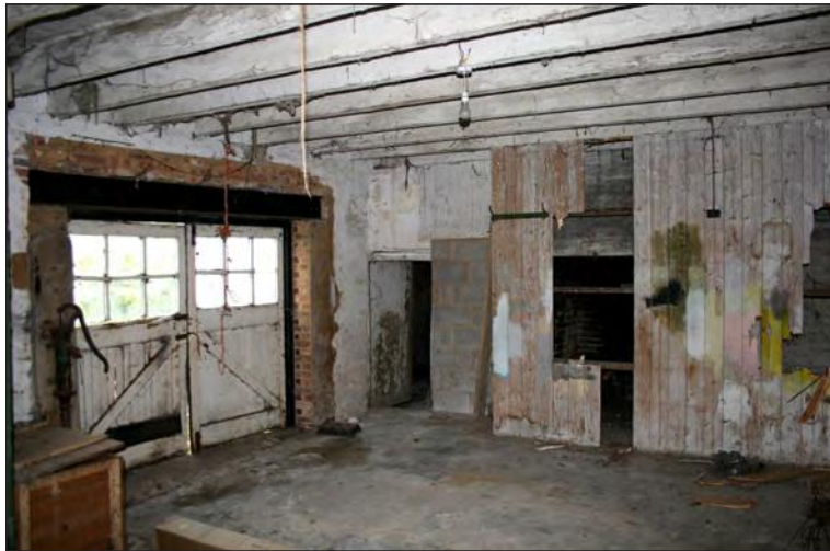
Plate 35. Interior of Building C, fireplace to right
