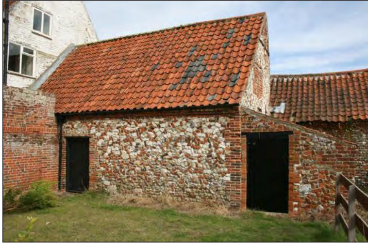
Plate 33. Southern elevation of Building C
