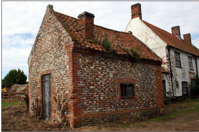
Plate 37. Building D facing south-west
