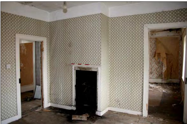
Plate 23. Fire-place first floor central bedroom Building A
