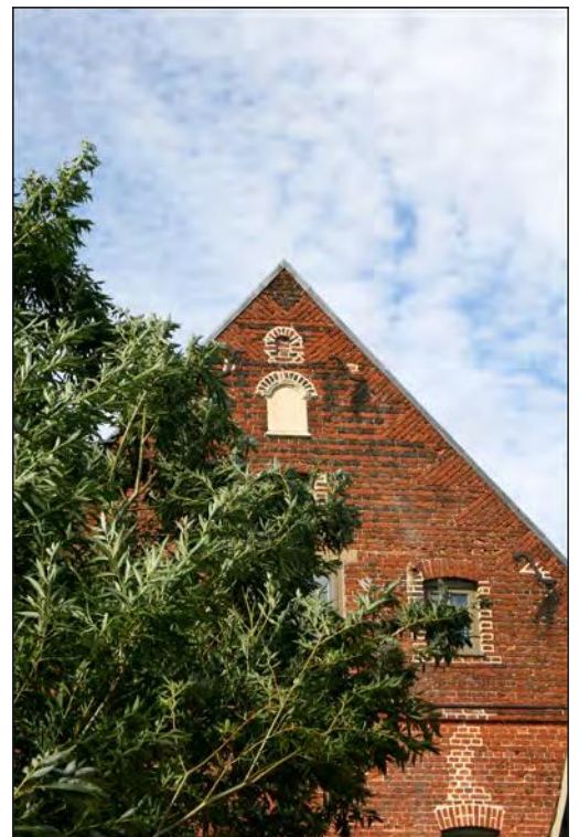
Plate 52. Ivy Farm barn southern elevation
