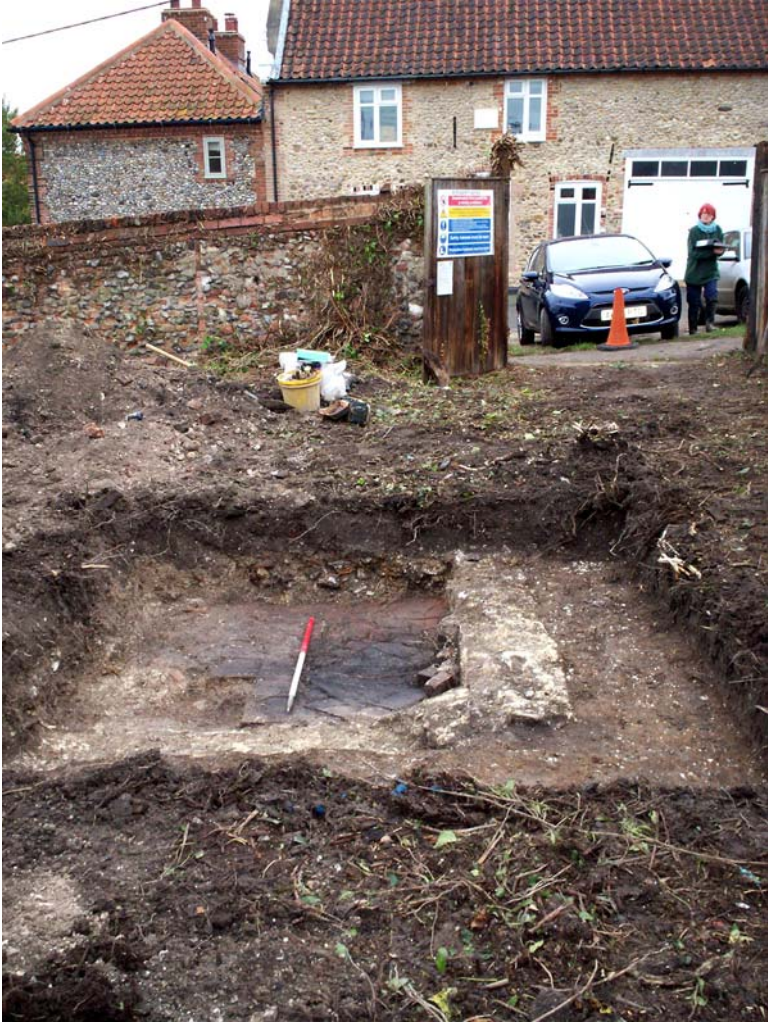
Plate 2. Post-excavation showing building with Jolly Sailors Yard beyond, looking east, 1m scale
