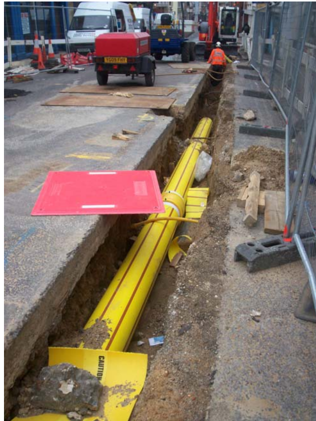
Plate 5: Groundworks in the area of St. Augustine's Gates, facing south
