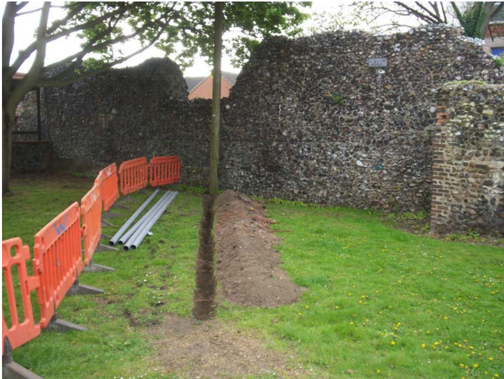
Plate 2. New service trench with the city wall in the background
