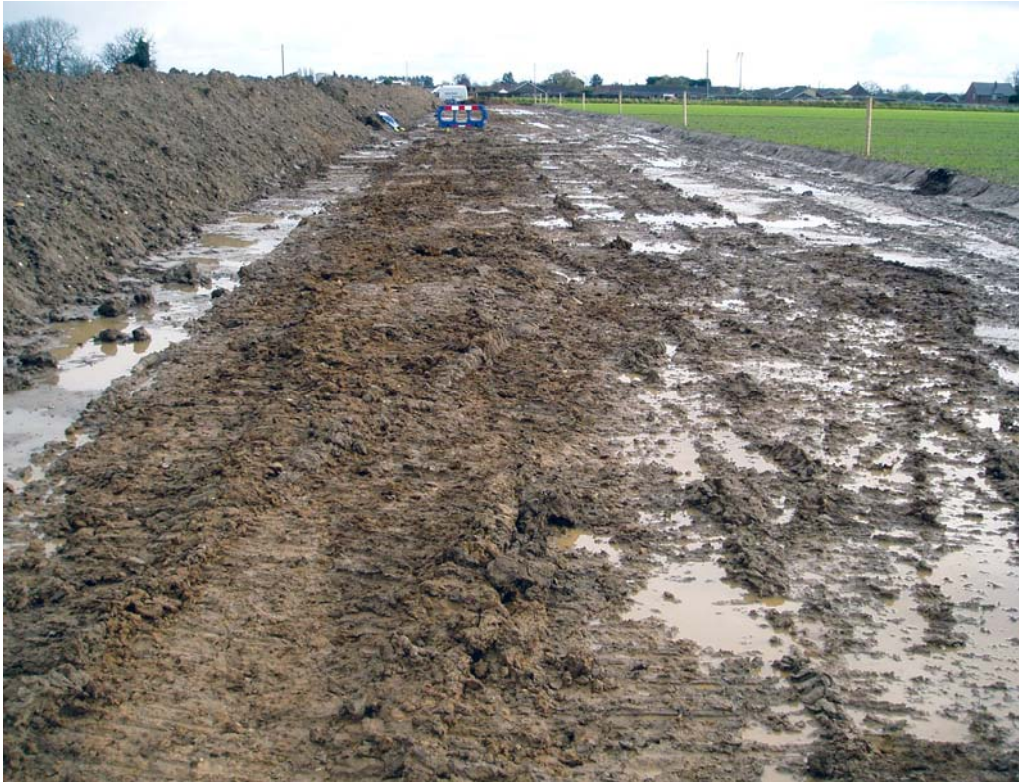
Plate 2. Pipeline easement and spoil heaps
