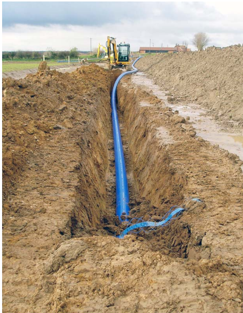
Plate 1. Natural deposits into which pipe trench was cut
