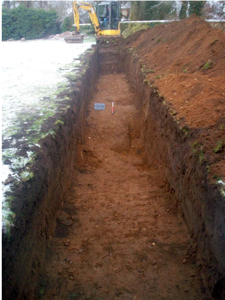
Plate 1: The trench facing north-east
