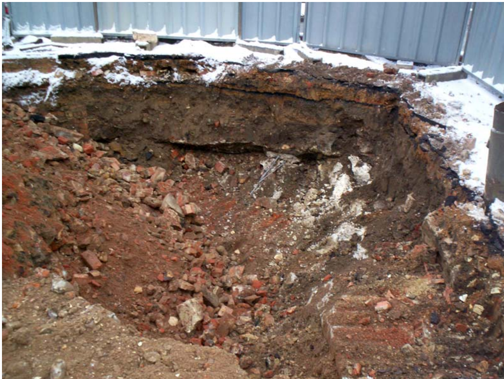
Plate 1. North end of site facing west showing brick rubble
