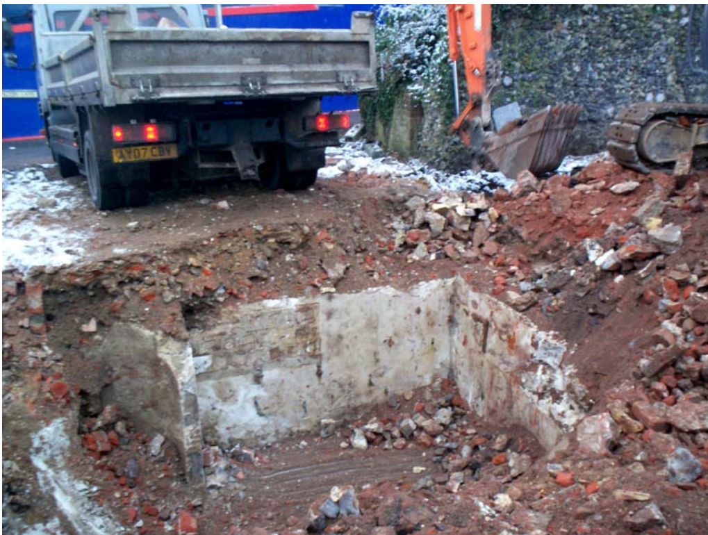
Plate 3. Below-ground elements of the former public conveniences, facing north-east,
