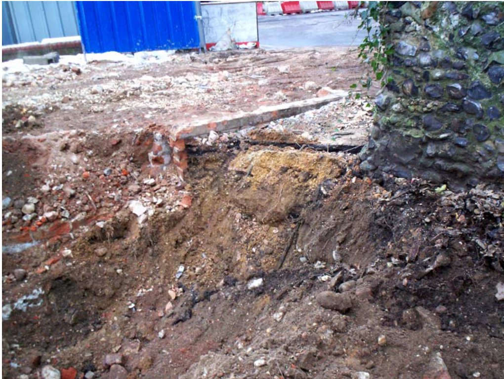
Plate 4 Medieval wall facing south showing base of wall exposed during excavation
