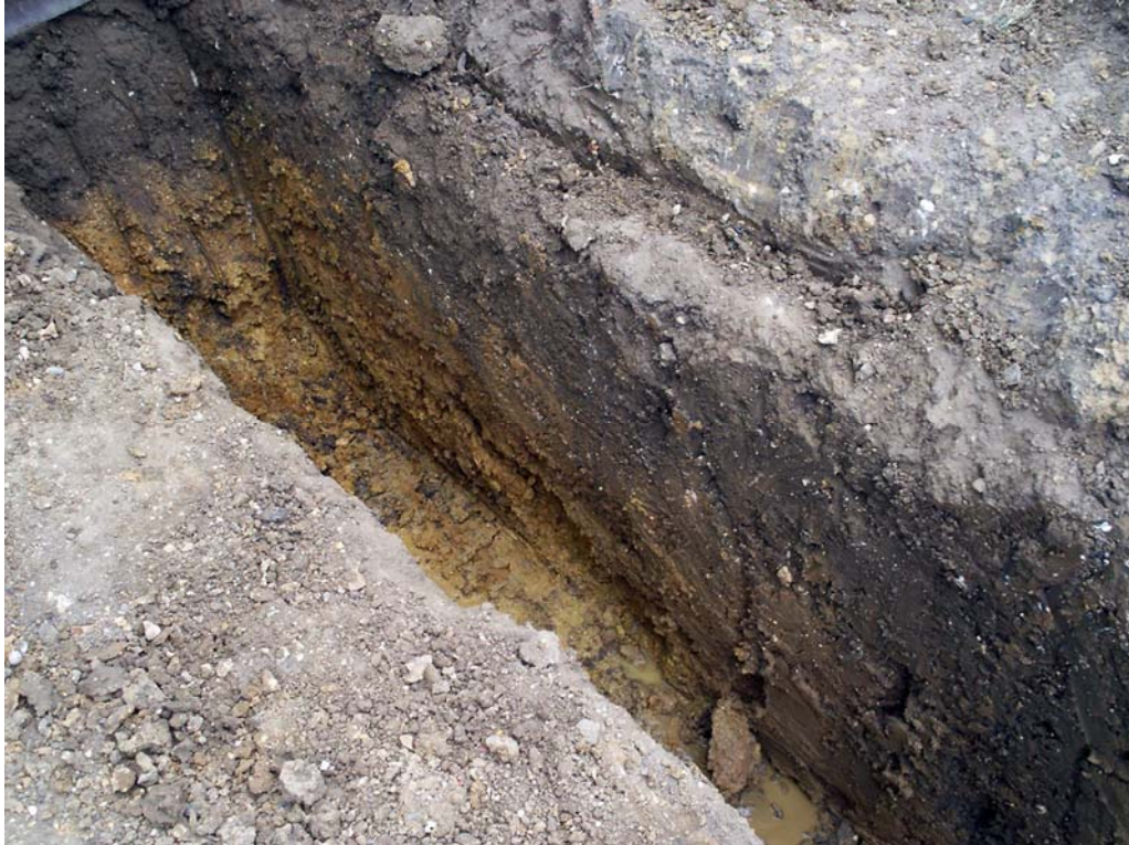
Plate 4. Trench at the south of the building showing where the level of the natural rises
