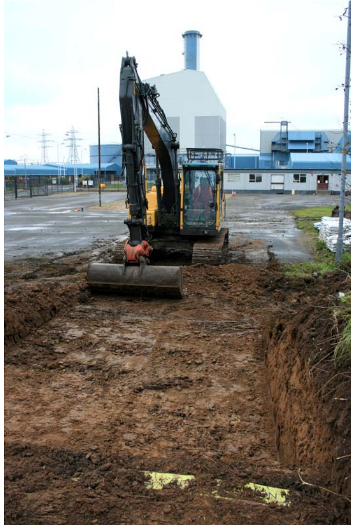
Plate 2. Machining Trench 3, looking south-west
