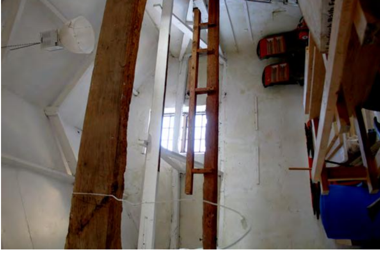
Plate 94. Building B north cell, facing north
