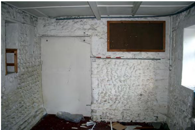
Plate 65. Building A, facing north
