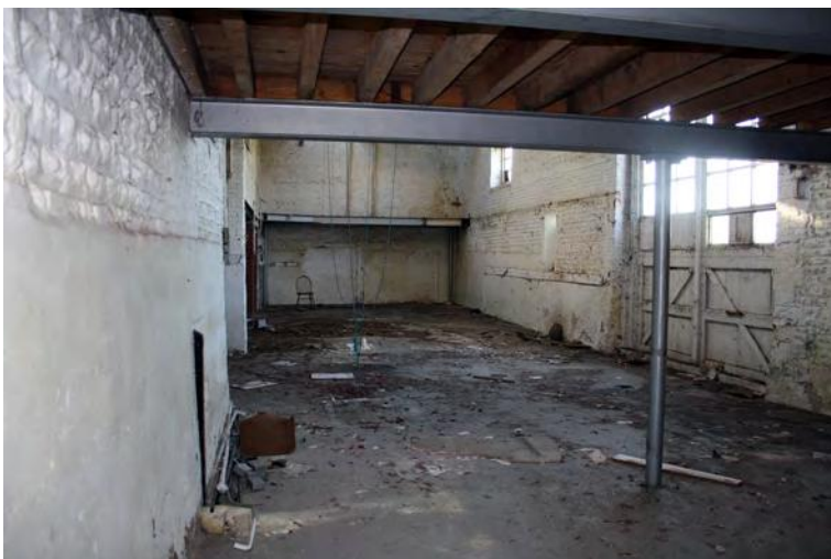
Plate 55. Building A interior, looking south
