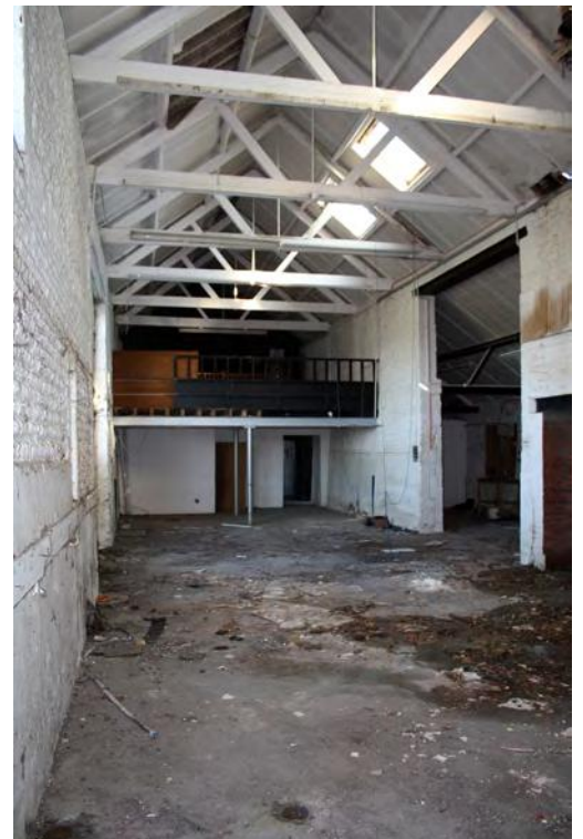
Plate 56. Building A interior, facing north
