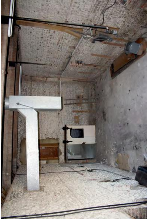
Plate 74. Building A interior, looking south from gantry
