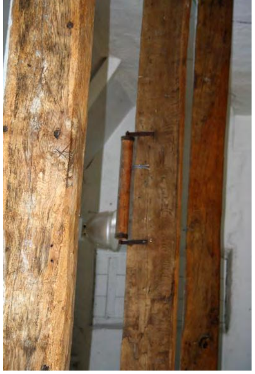
Plate 80. Building B northern roller
