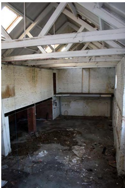
Plate 67. Building A, facing south-east from gantry
