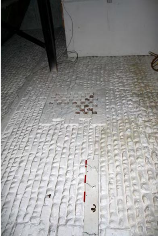
Plate 62. Geometric vent, facing north-west, 0.5m scale
