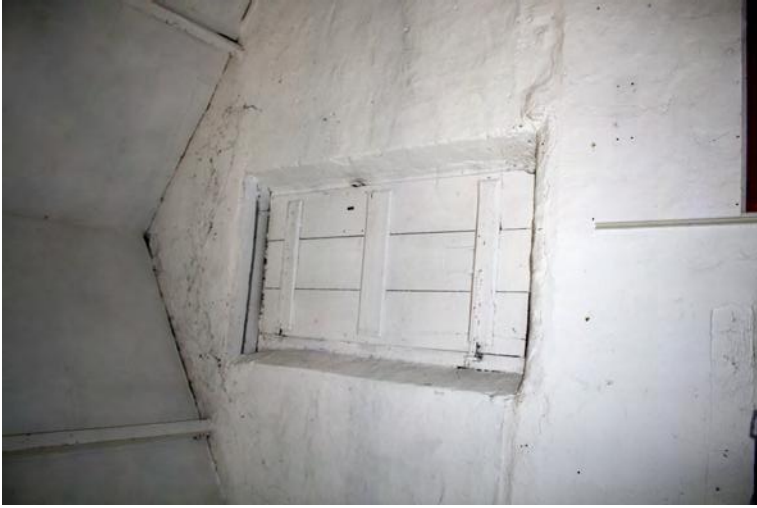
Plate 81. Building B partition wall hatch
