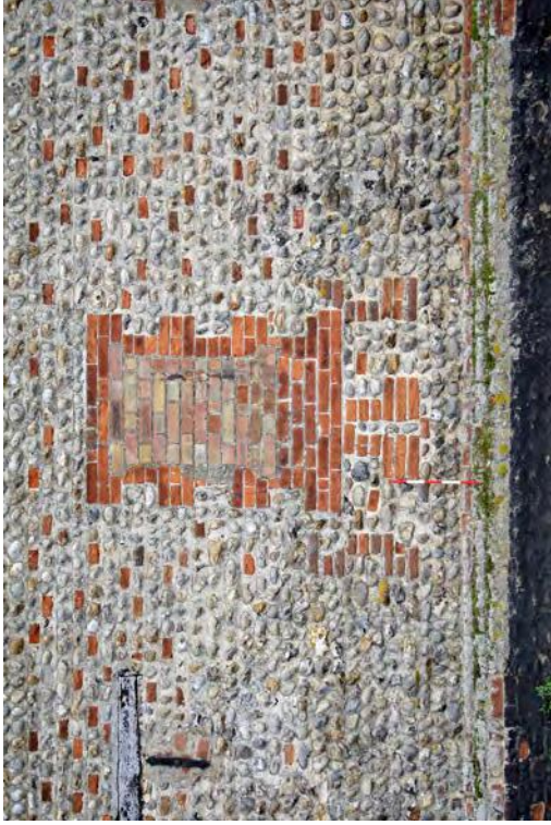
Plate 113. Blocked opening on Building A, 0.5m scale
