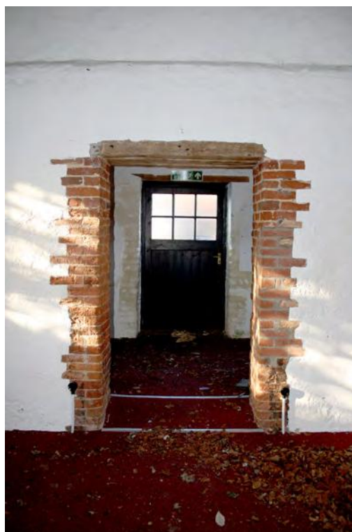
Plate 86. Building B interior southern cell, facing west
