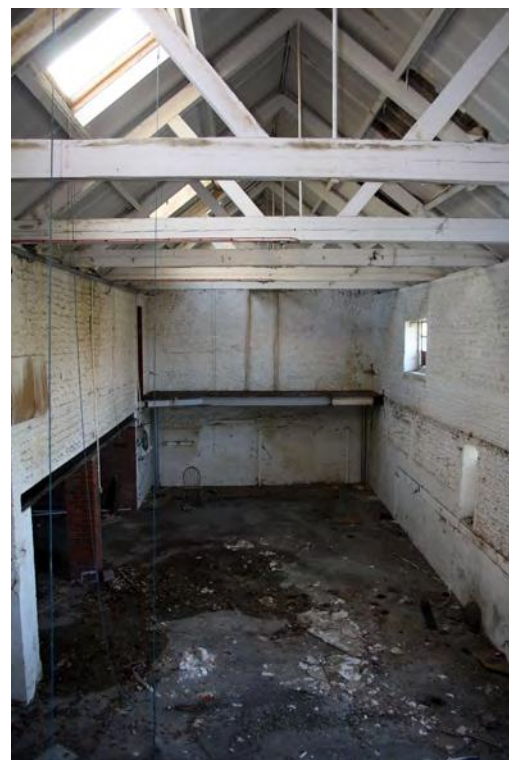
Plate 66. Building A, facing south from gantry
