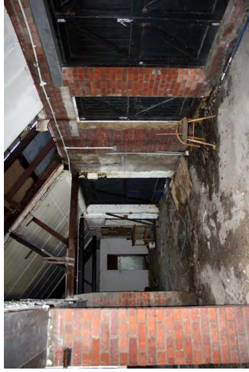
Plate 60. Interior building A, facing north
