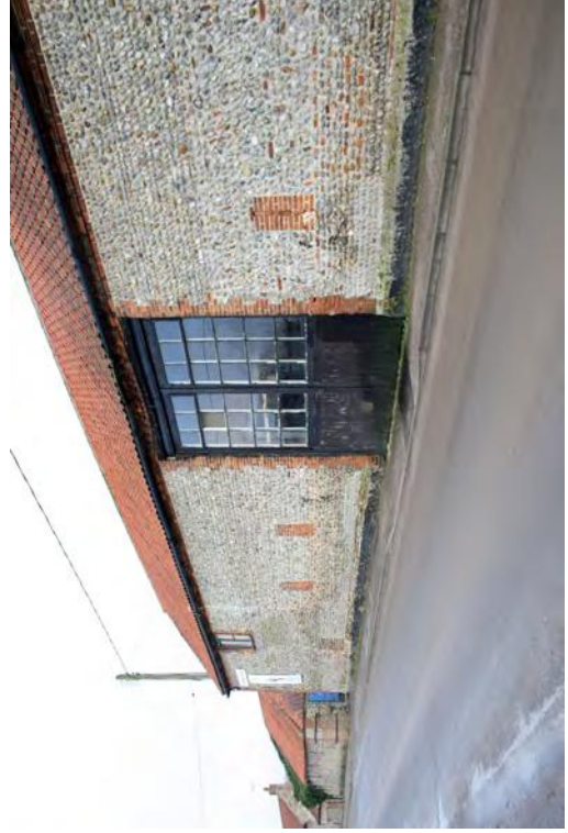
Plate 115. West elevation north end Building A
