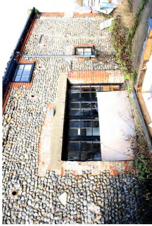
Plate 36. Building B, facing north-west
