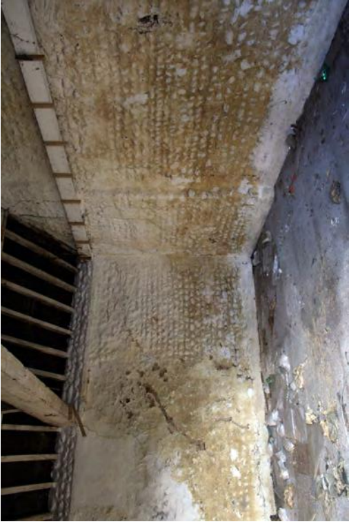
Plate 29. Building C interior, facing north-east
