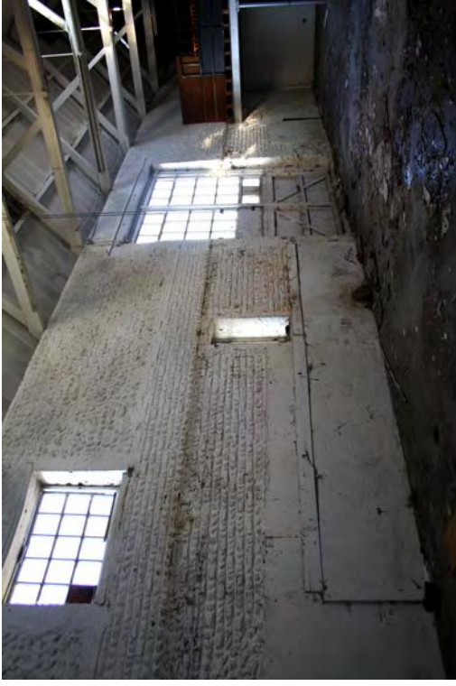
Plate 58. Building A interior, facing north-west
