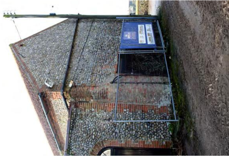
Plate 5. Building A north gable, facing east
