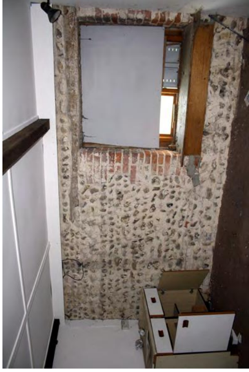
Plate 76. Building A interior north end upper floor, facing west
