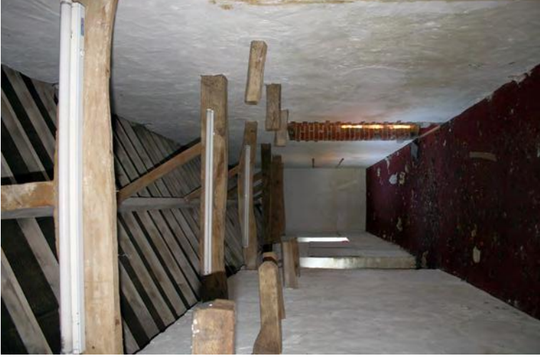
Plate 90. Building B corridor, facing north
