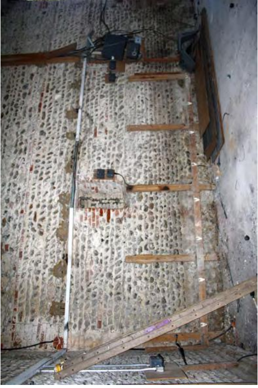
Plate 50. Building A interior, looking west
