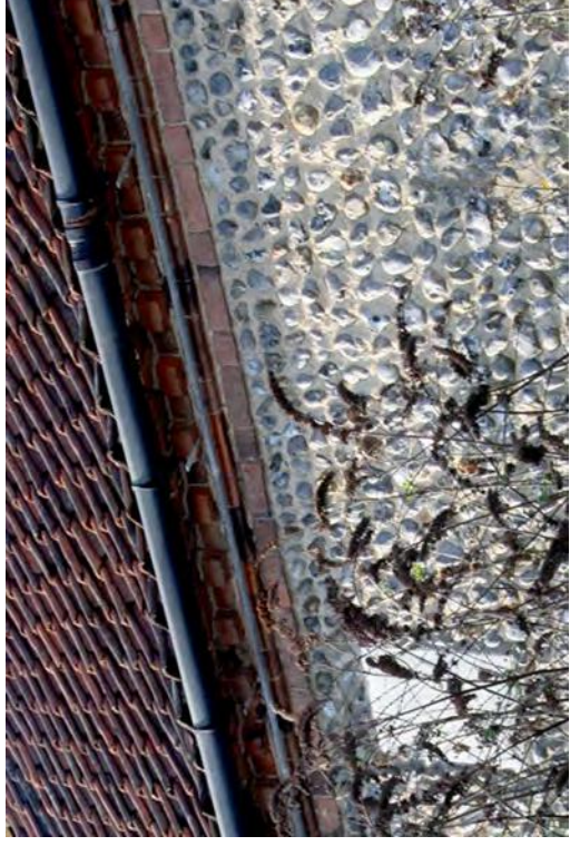
Plate 96. Dentil cornice on Building A
