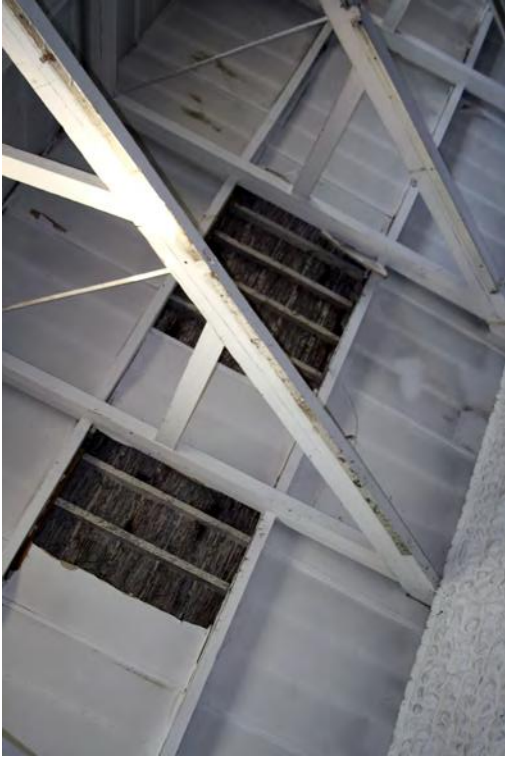
Plate 61. Interior of Building A, straw below tiles
