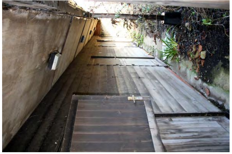
Plate 43. Building D, facing north
