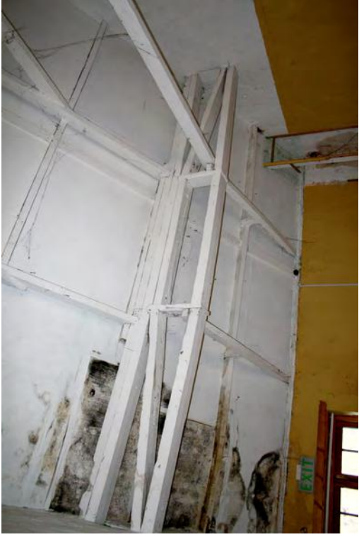
Plate 93. Building B central cell roof detail
