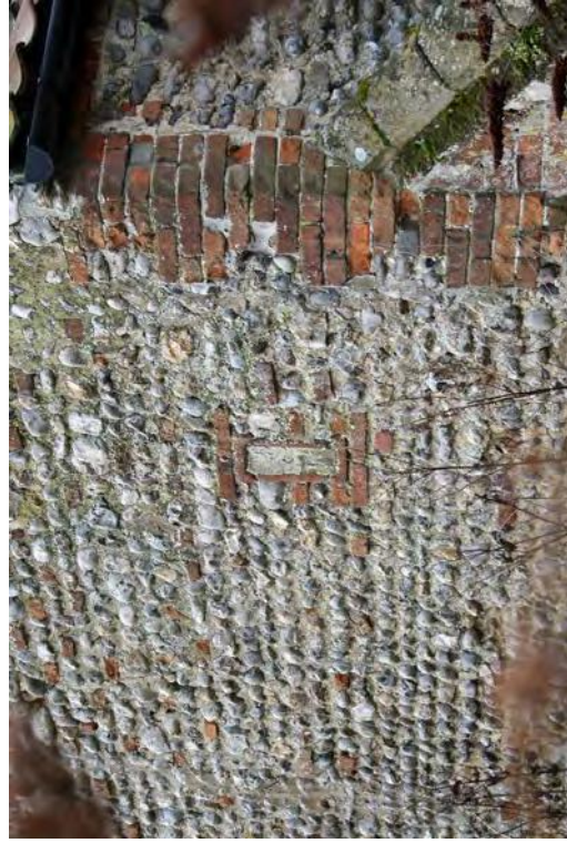
Plate 111. Blocked opening on Building C
