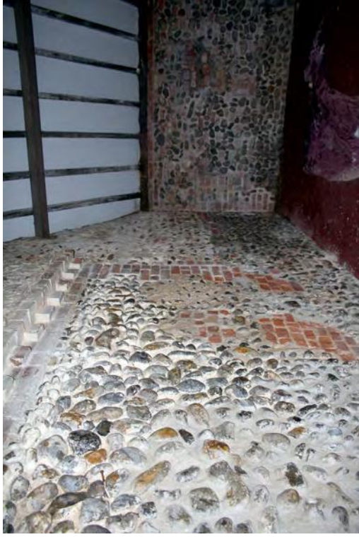
Plate 41. Interior of Building F, south end facing south
