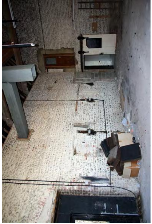
Plate 71. Building A interior, facing south
