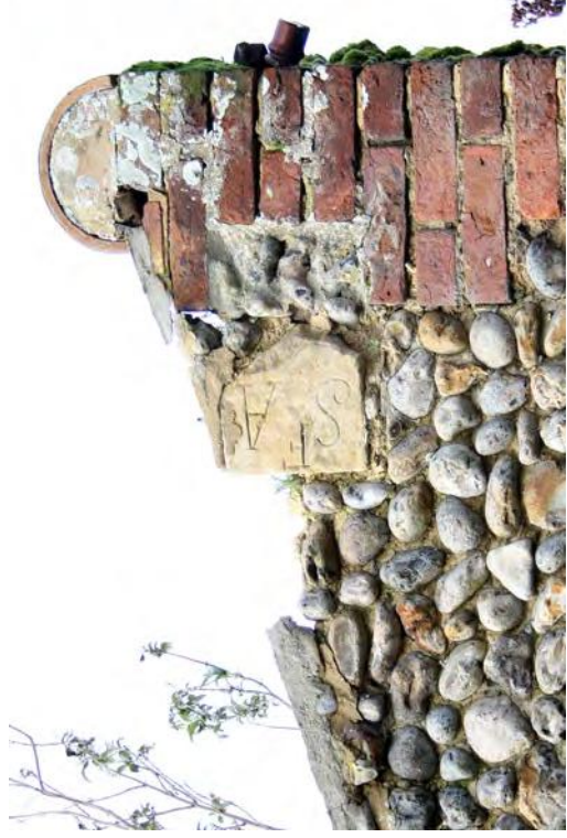
Plate 108. Initialled stone on north-east corner Building H
