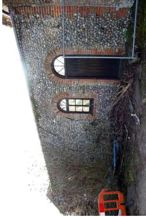
Plate 99. Building H north elevation
