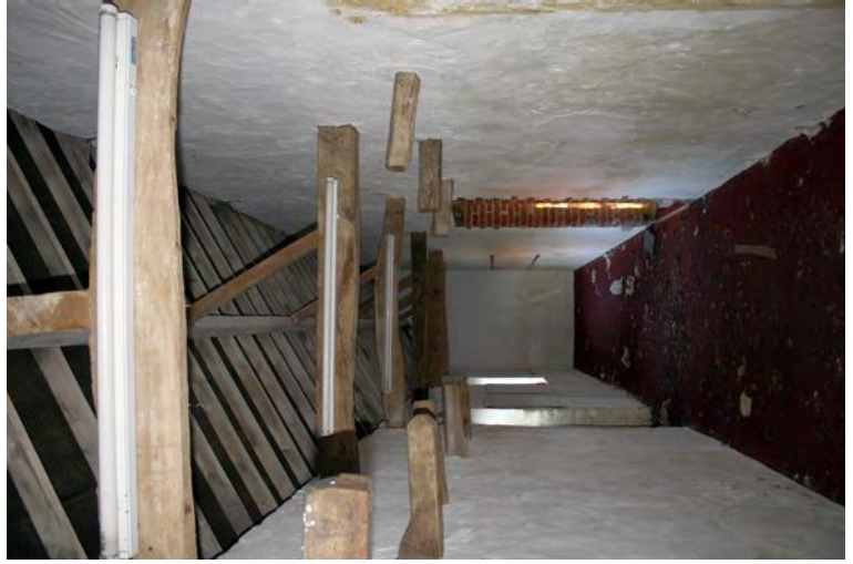
Plate 91. Building B corridor, facing south
