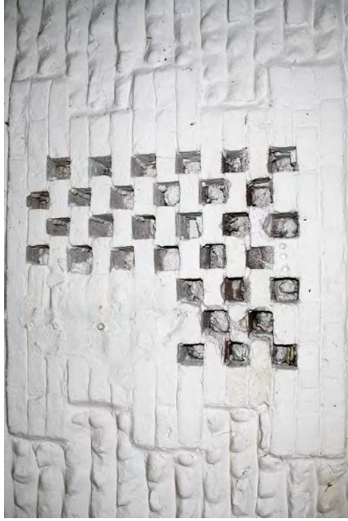
Plate 63. Geometric vent, facing west
