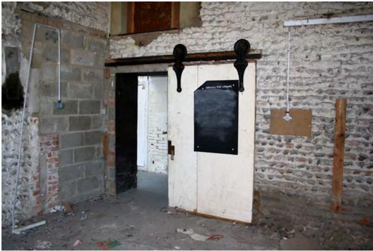
Plate 53. Building A sliding door, looking south
