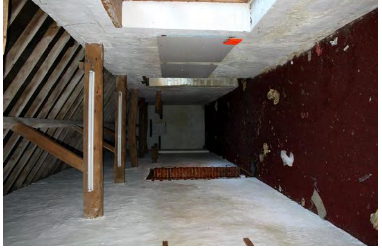
Plate 44. Building B south corridor, facing south
