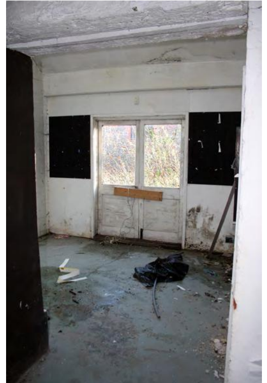
Plate 54. Interior of porch, Building A, facing east
