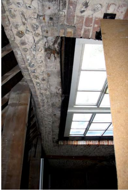
Plate 75. Door lintel Building A
