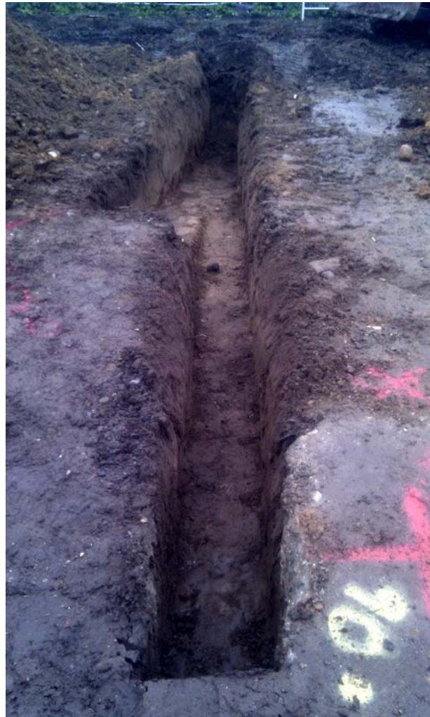
Plate 2. Small service trench alongside Trench 12
