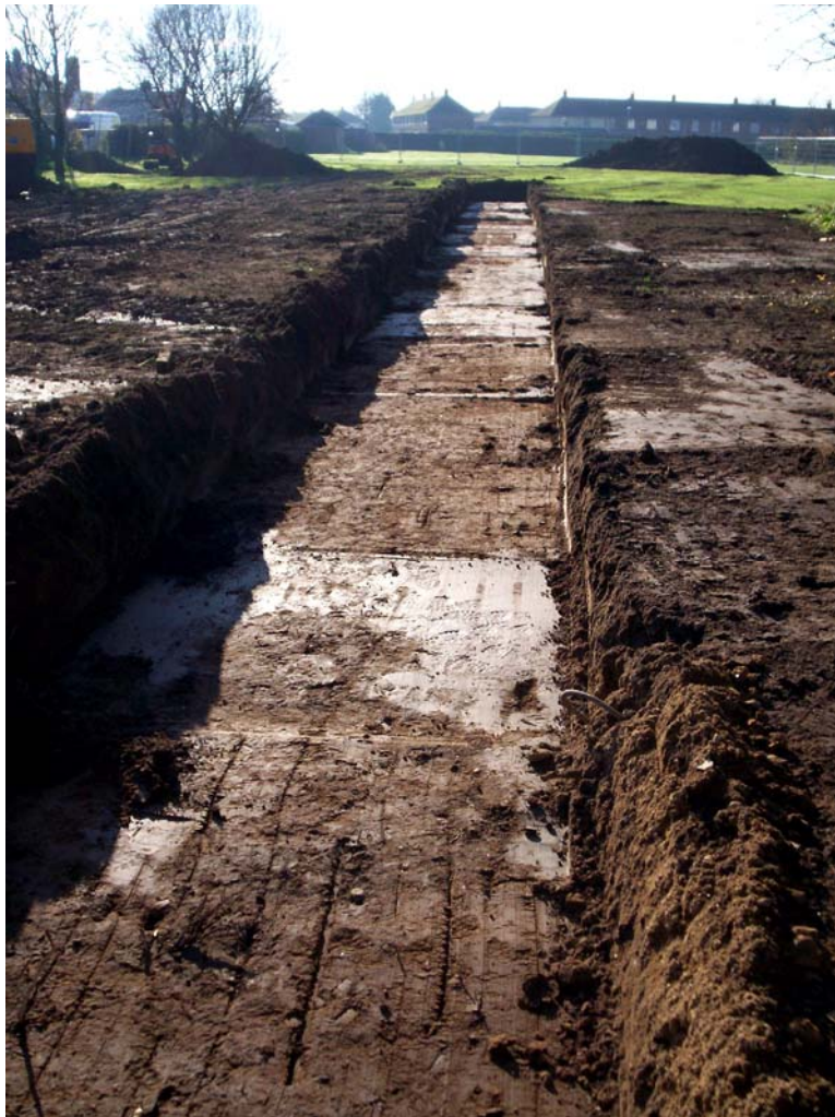
Plate 1. Groundworks for the temporary car park and works compound
